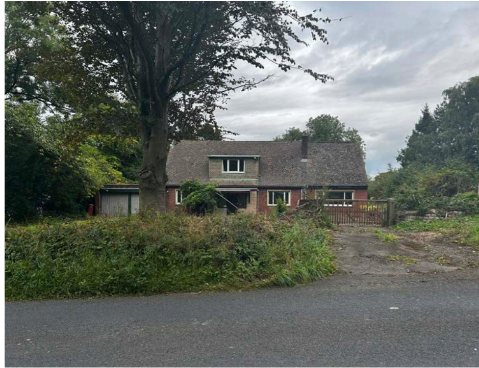
View of the site from Ribchester Road.
