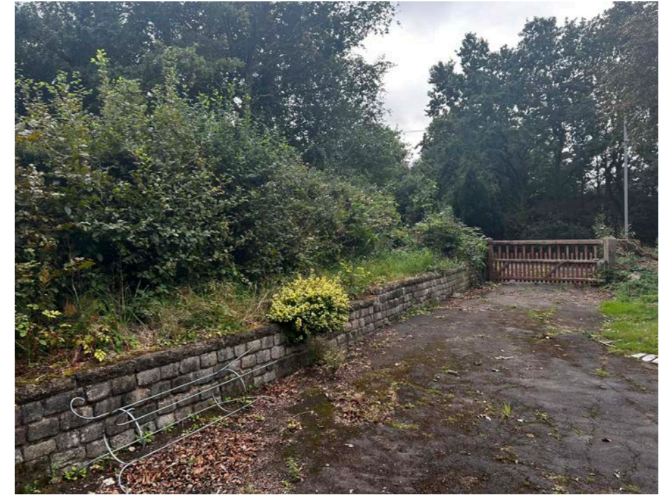
Retaining wall and planting between adjacent land.
