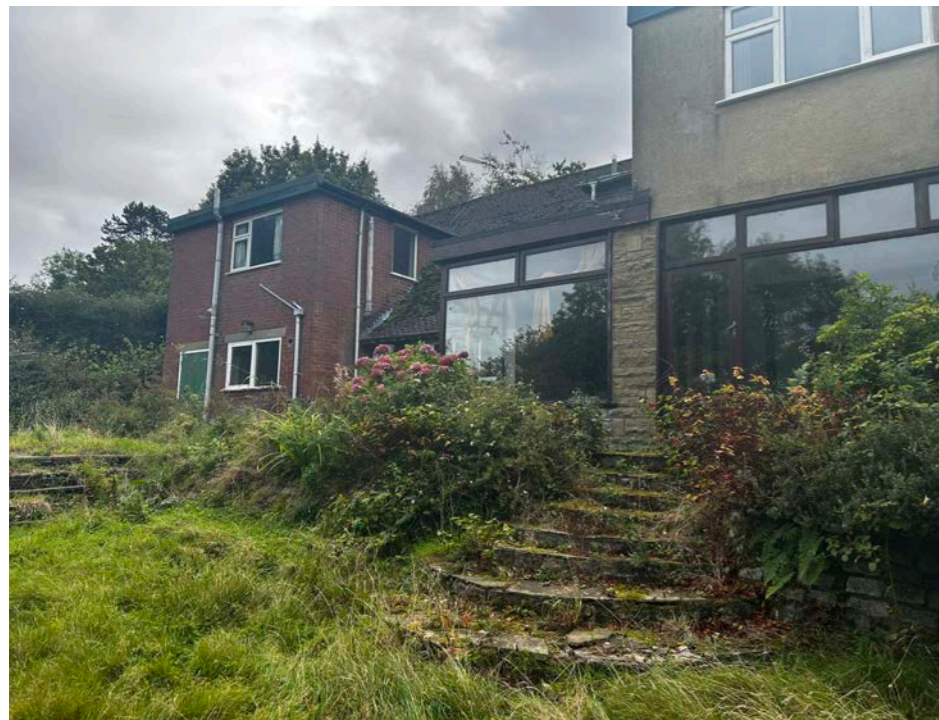
Rear elevation, terracing and steps.
