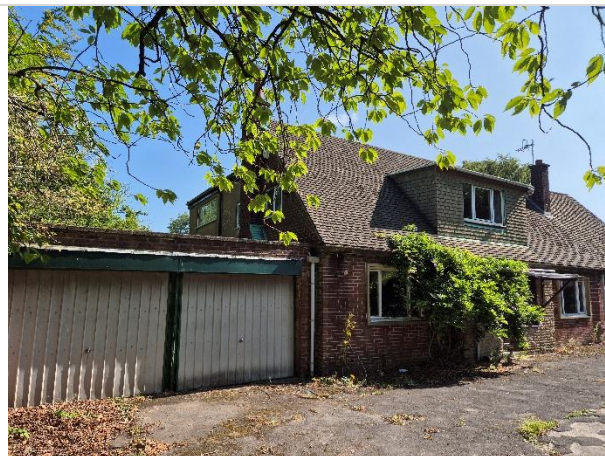
Photo 2: Southern elevation of the house showing hardstanding
