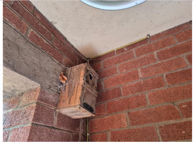
Photo 20: Sealed area beneath porch at eastern elevation (showing bird box)
