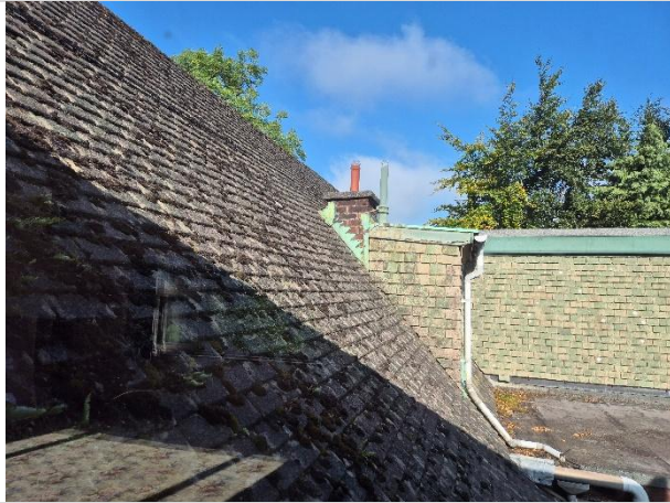
Photo 19: Intact tiles at roof pitch
