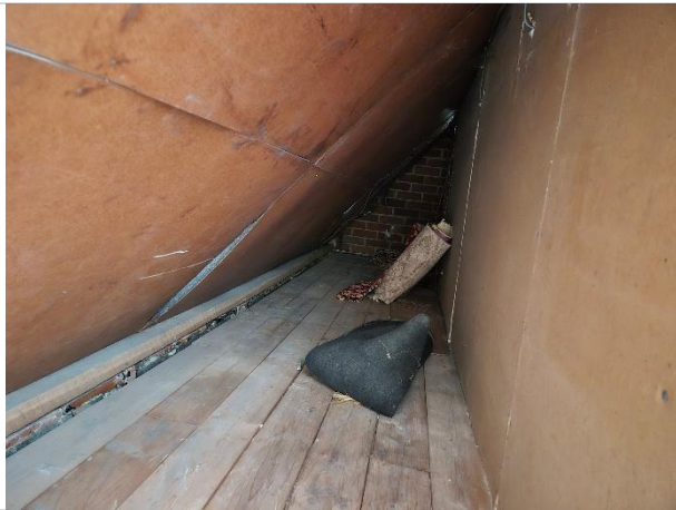
Photo 21: Under eaves roof void at house
