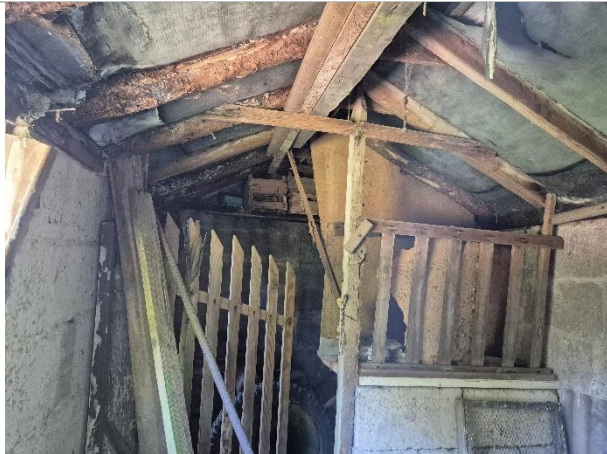
Photo 27: Interior of shed
