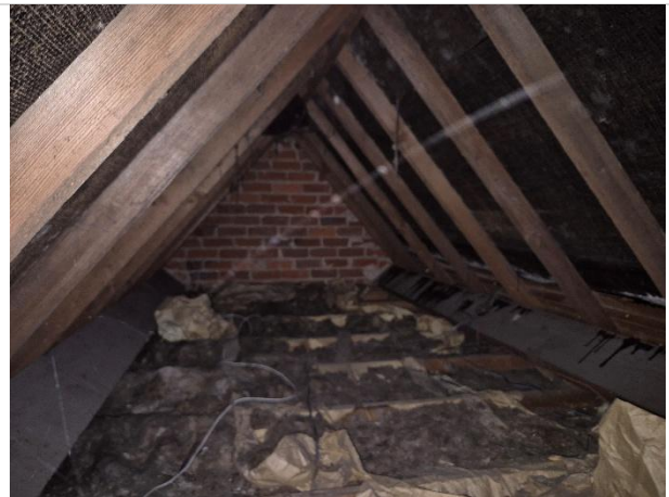
Photo 24: Roof void at western end of house
