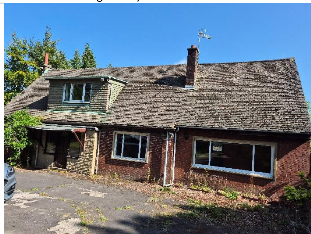
Photo 12: Southern elevation and roof of house
