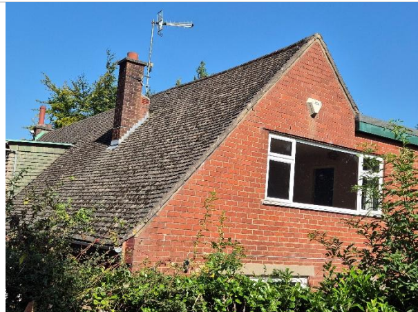
Photo 14: Eastern elevation of the house
