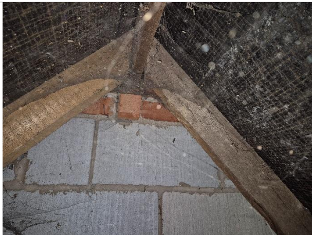
Photo 23: Roof void at eastern end of house
