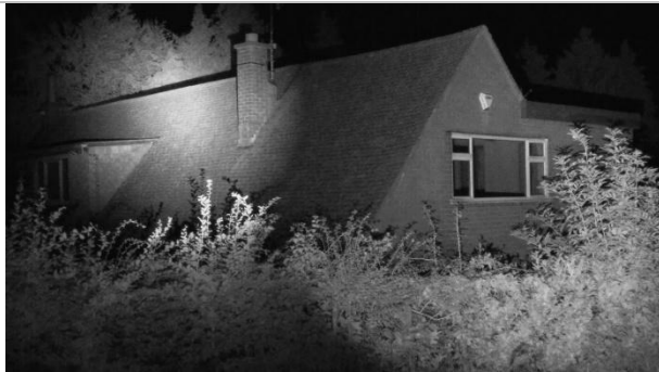
Photo 29: NVA view Survey Position 2
