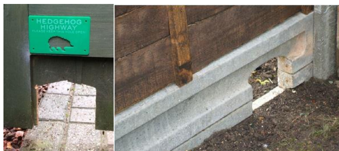
Insert 1: Showing wildlife access gap within fencing
