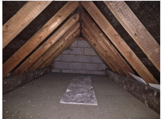
Photo 22: Roof void at eastern end of house
