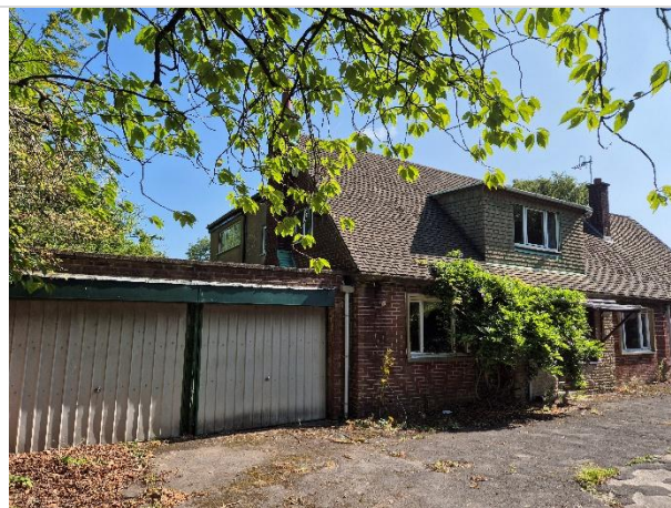
Photo 2: Southern elevation of the house showing hardstanding
