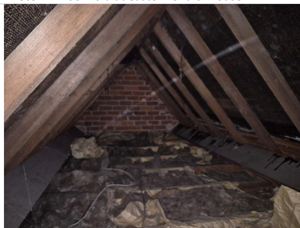
Photo 24: Roof void at western end of house
