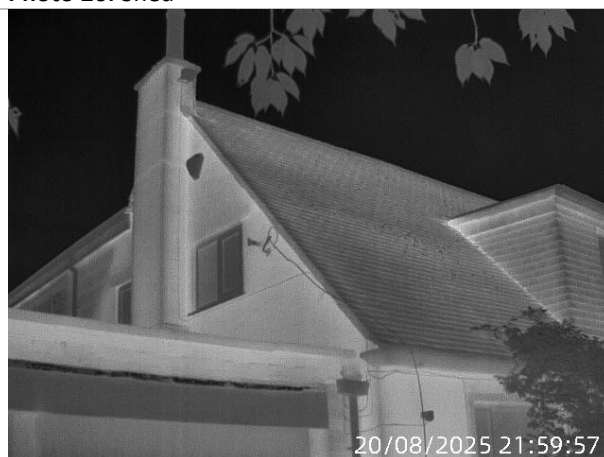
Photo 28: NVA view Survey Position 1
