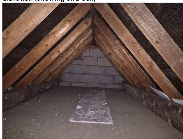
Photo 22: Roof void at eastern end of house
