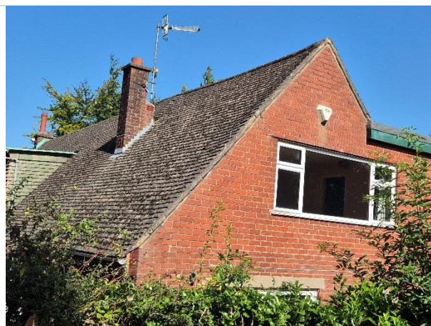
Photo 14: Eastern elevation of the house
