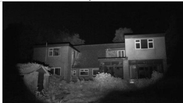
Photo 30: NVA view Survey Position 3
