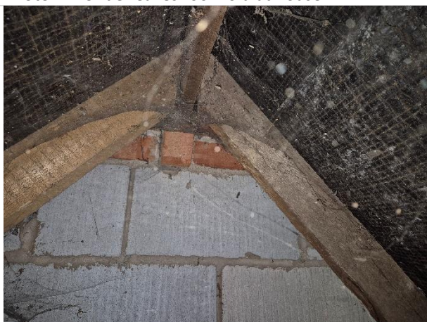
Photo 23: Roof void at eastern end of house
