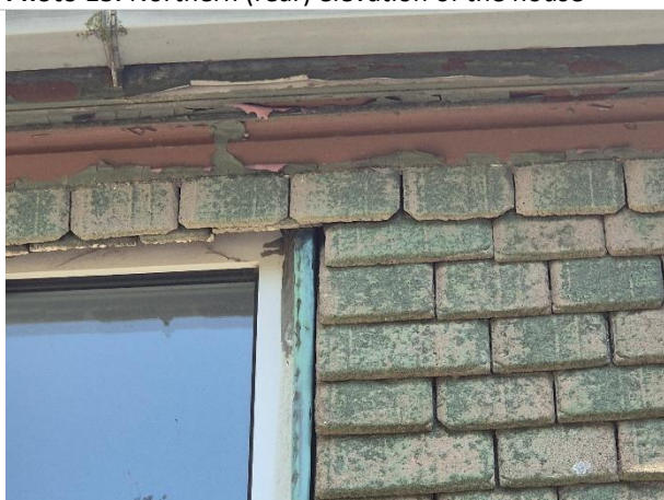
Photo 15: Gap / potential roost features (PRF) at frame between hanging tiles and window frame
