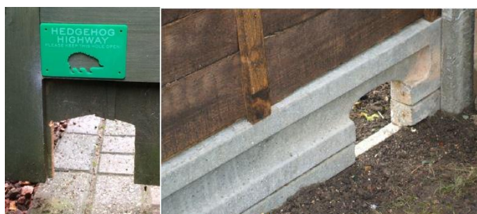
Insert 1: Showing wildlife access gap within fencing
