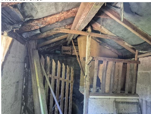
Photo 27: Interior of shed
