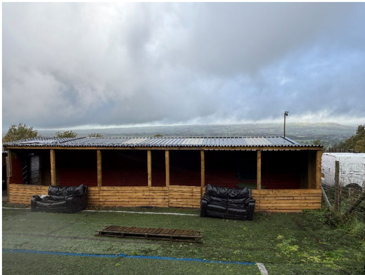
Retrospective permission is sought for the erection of a timber and corrugated metal lean-to/cover to the rear of the dog care facility
