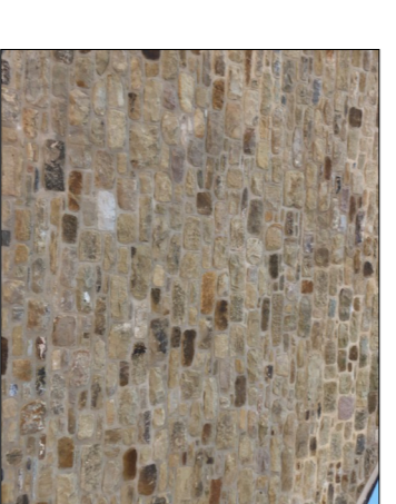
External walls finished in Traditional Stonework
