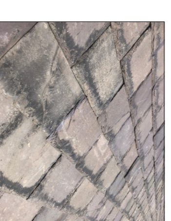
Roof finished in Natural Slate
