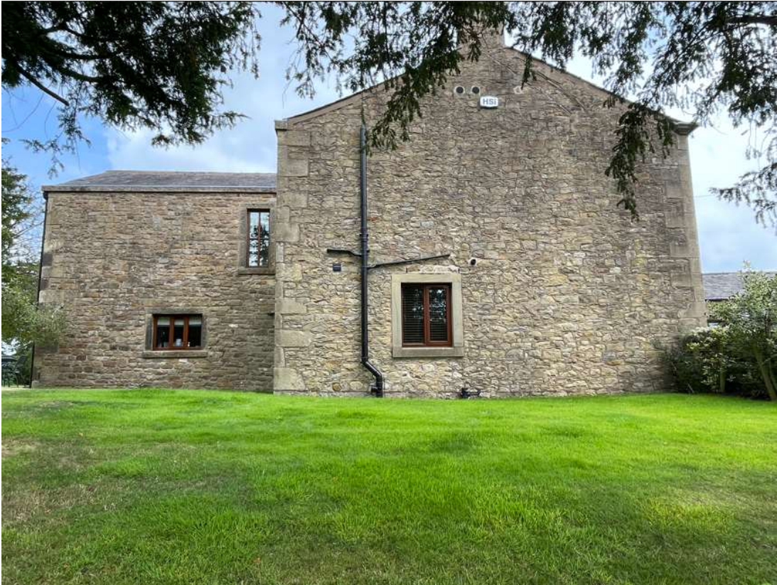
Photo showing Existing West Elevation where proposed extension is to be provided.
