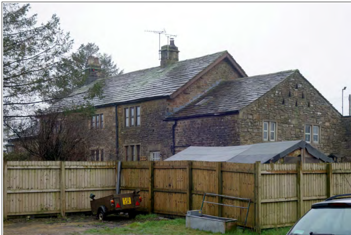
Photo 1: Lower Edge Farmhouse (the listed building): south front, viewed from the east
