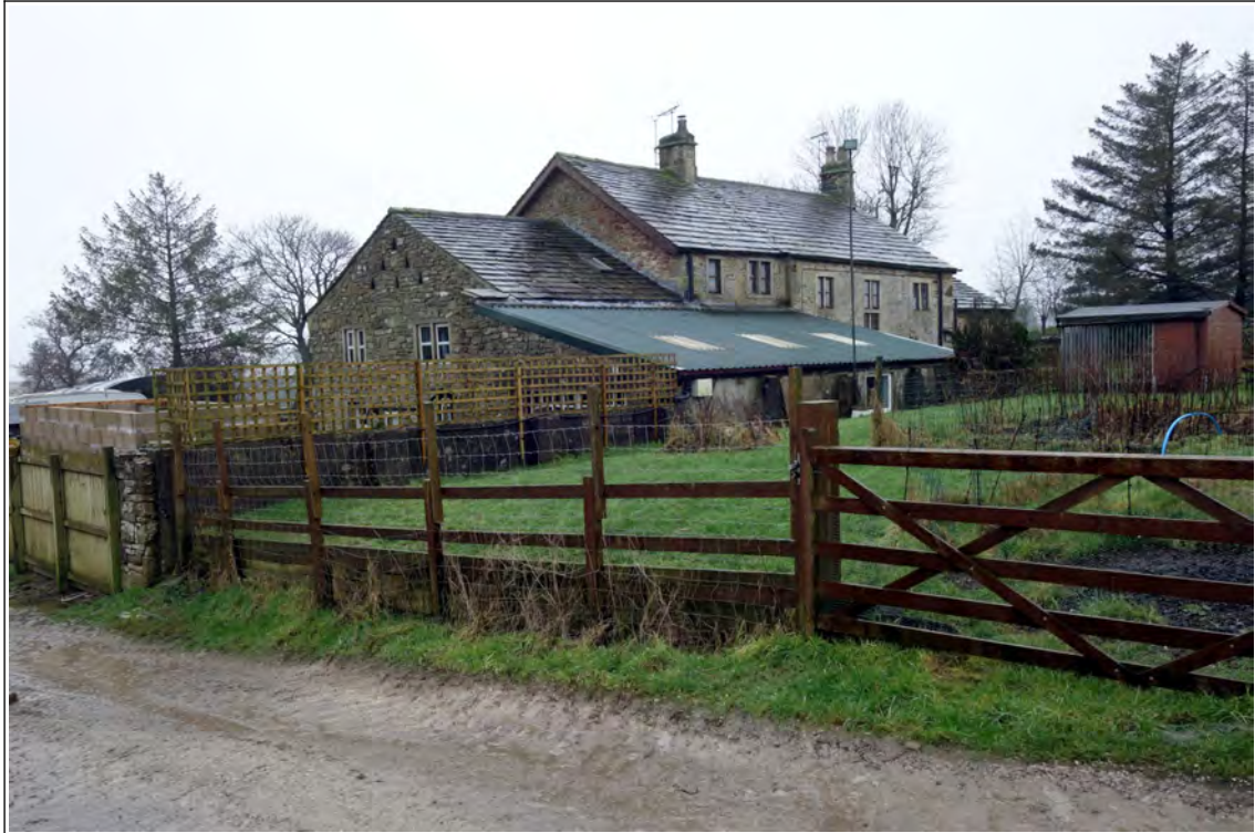
Photo 2: Lower Edge Farmhouse: rear elevation, viewed from the north-east
