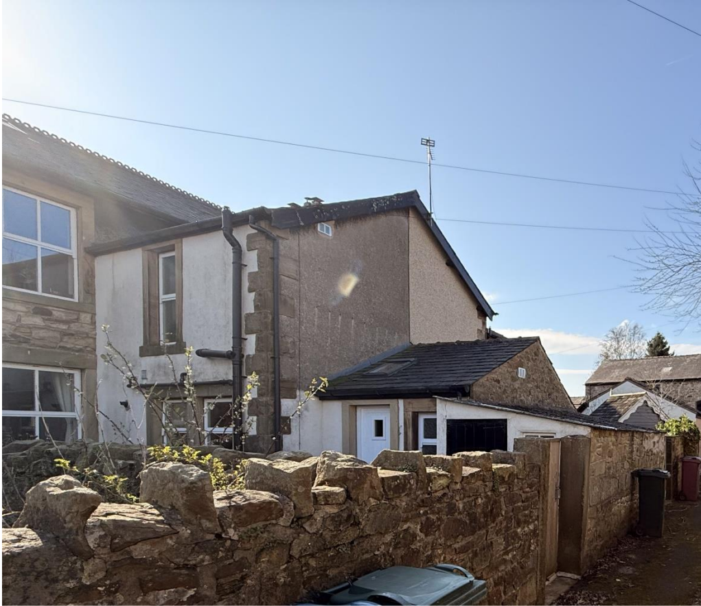
Photograph showing rear extensions at 3 Valley View
