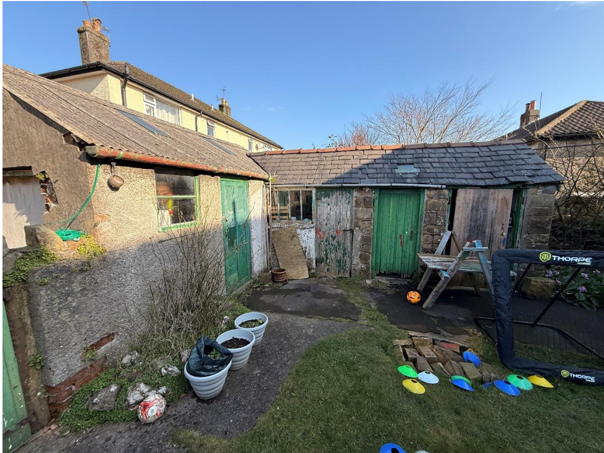
Photo showing outbuildings which have been proposed for demolition
