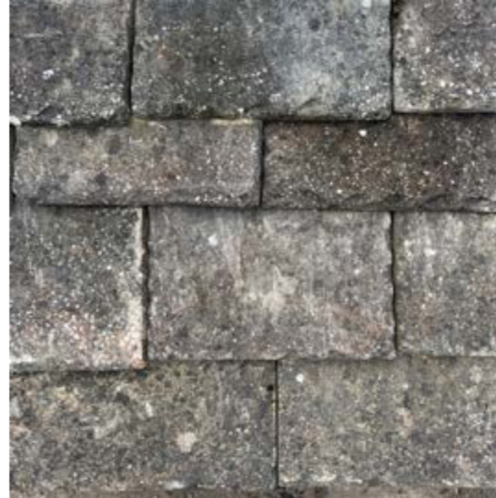
STONE ROOF PAVING FLAGS - RECLAIMED - To re roof front and rear elevations, numbering and reusing original roof flags wherever possible, topping up if required with reclaimed stone flags
