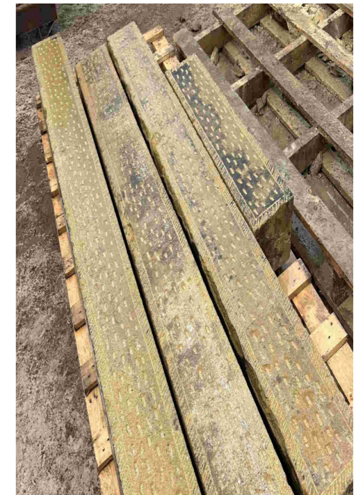
Reuse original Sandstone Quoins and Reuse original Sandstone Jambs for the Front Door Opening along with Sandstone Window
