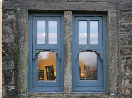
Existing windows viewed from outside
