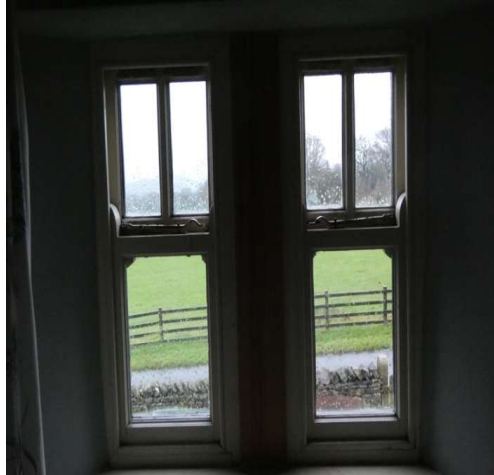
Existing windows viewed from inside
