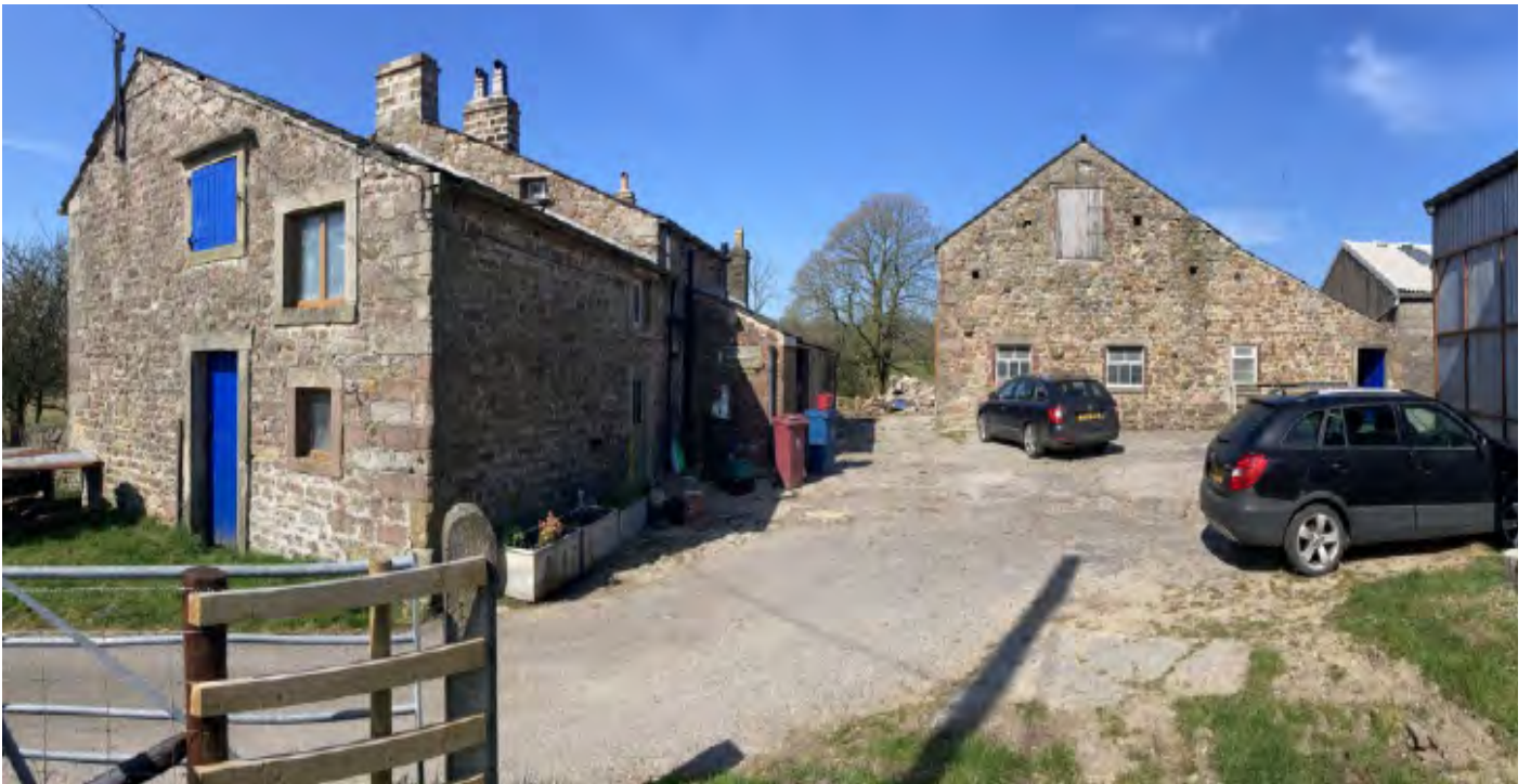
5. View of east approach to the farmyard showing the listed farmhouse to the left and the east gable of the barn to which this application related to the back.
