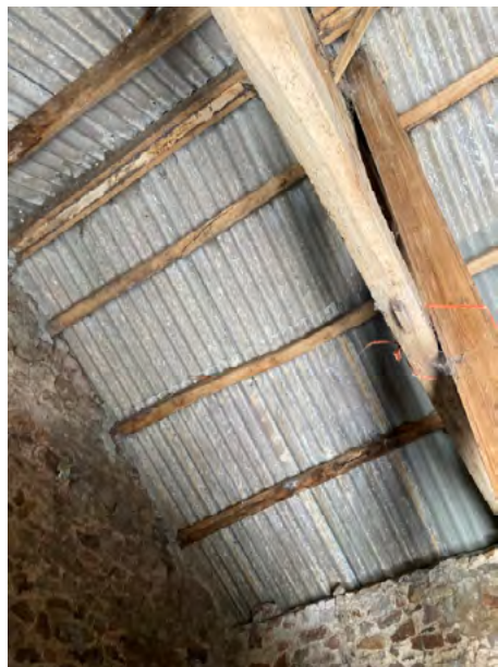
29. West bay north slope of main barn
