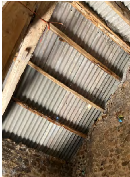
25. West end bay south slope of main barn.
