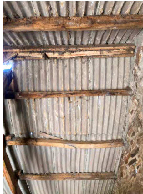
27. East end bay north slope of main barn
