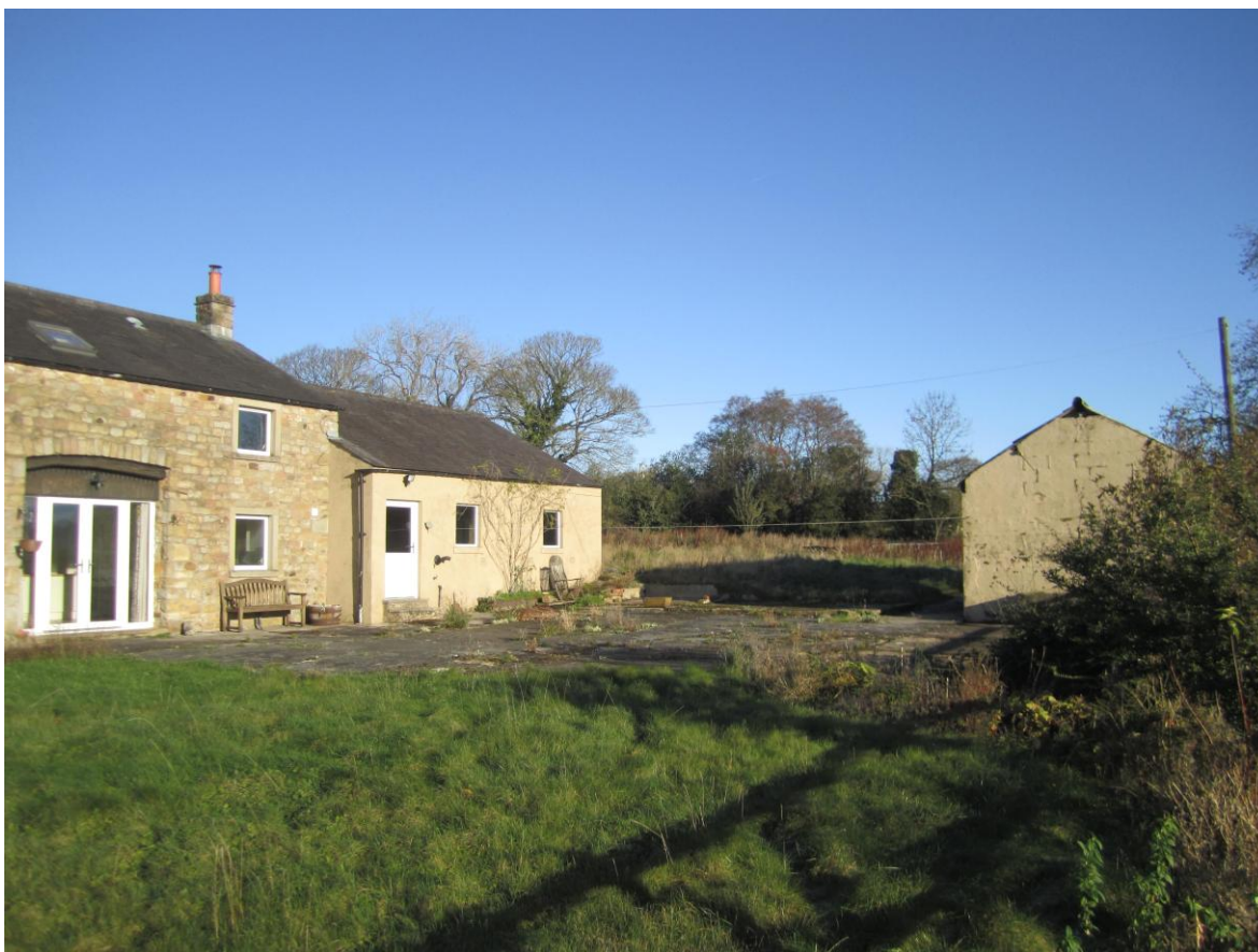
1. South east elevation of the attached garage.
