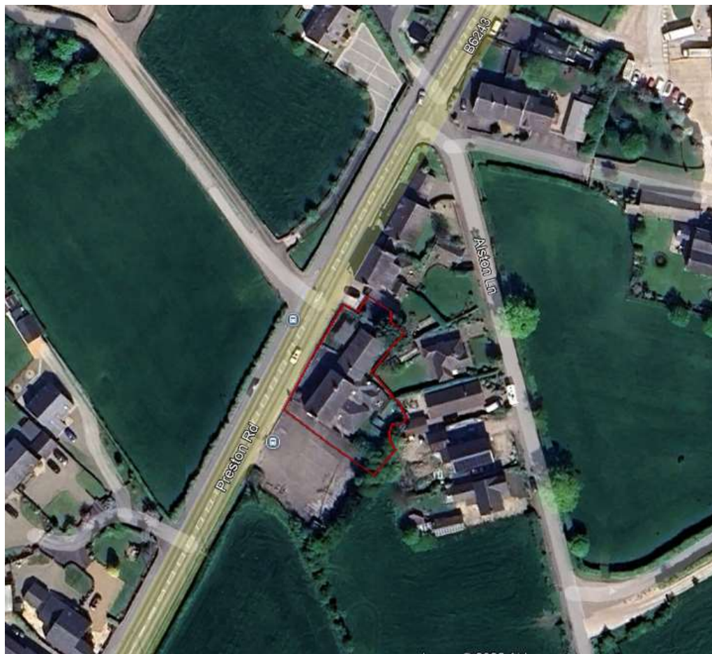
Figure 1: Aerial view of the approximate application site (edged red) and its wider setting
