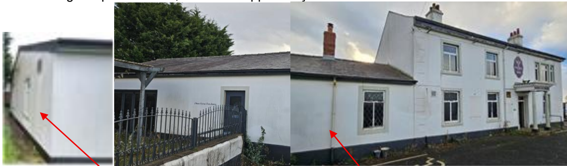
Front northwest Elevation.
