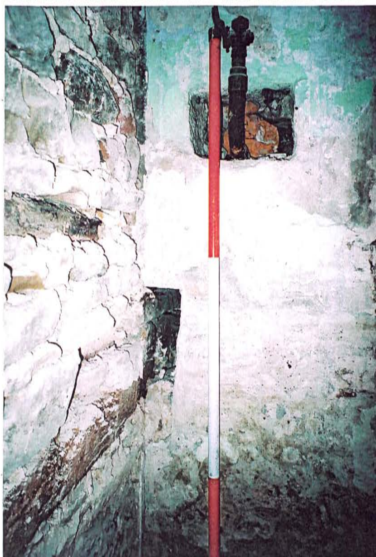
Pl. 2 West wall to former pantry of the farmhouse at its junction with the internal wall to the living room
