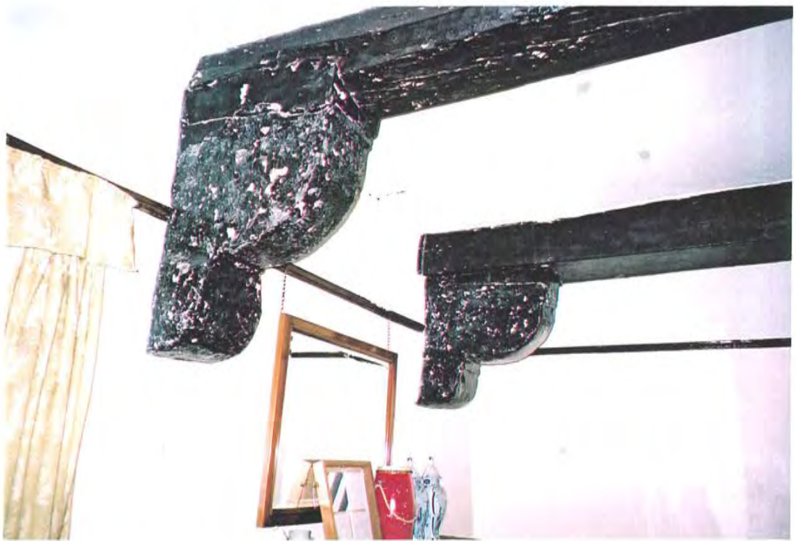
Pl. 14 Detail of corbels in external wall of living room
