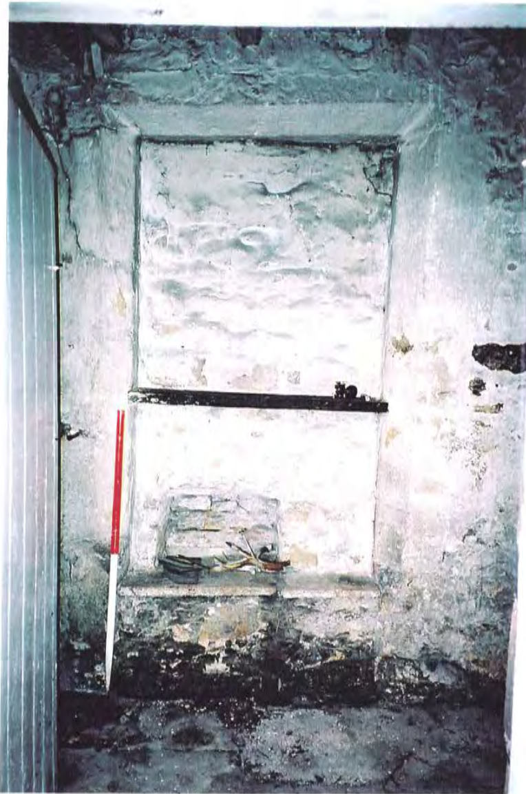
Pl. 17 Blocked doorway in farm cottage leading from stair turret porch to through-passage
