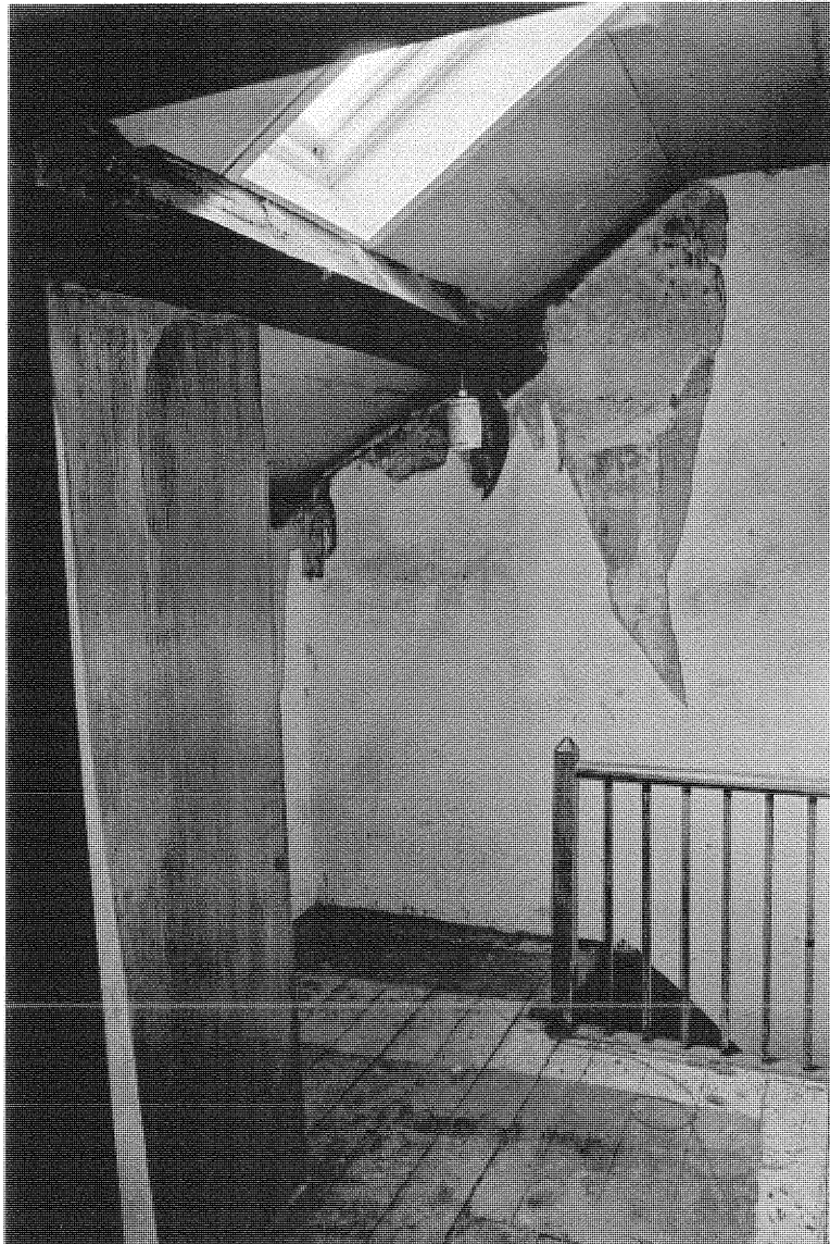
Pl. 18 First floor landing to the farm cottage
