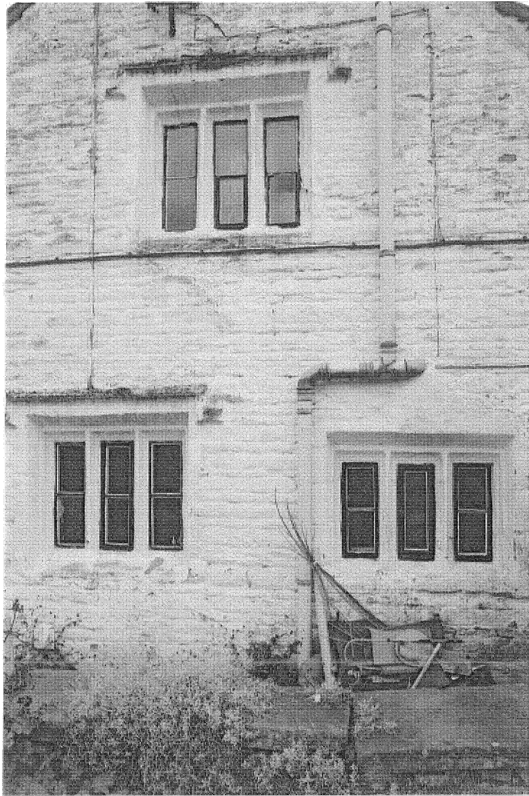
Pl. 7 Mullion windows to north elevation of the cross-wing
