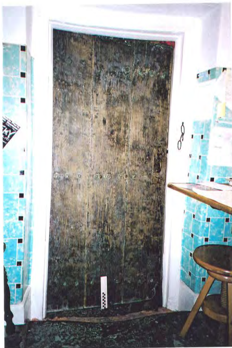
Pl. 15 Door between kitchen and pantry formed out of three oak planks
