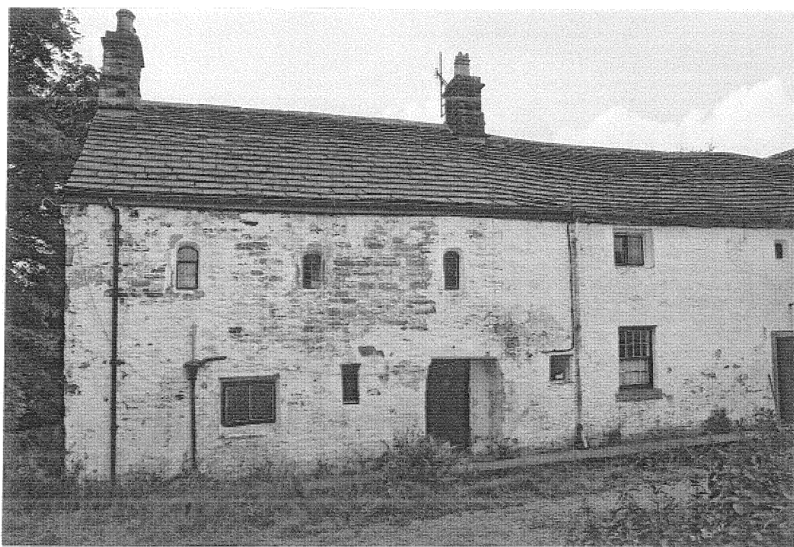
Pl. 8 Farm cottage showing the line of quoins at the junction with the farmhouse
