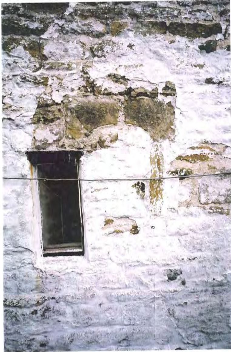
Pl. 9 Blocked-up round-headed window to ground floor of farm cottage
