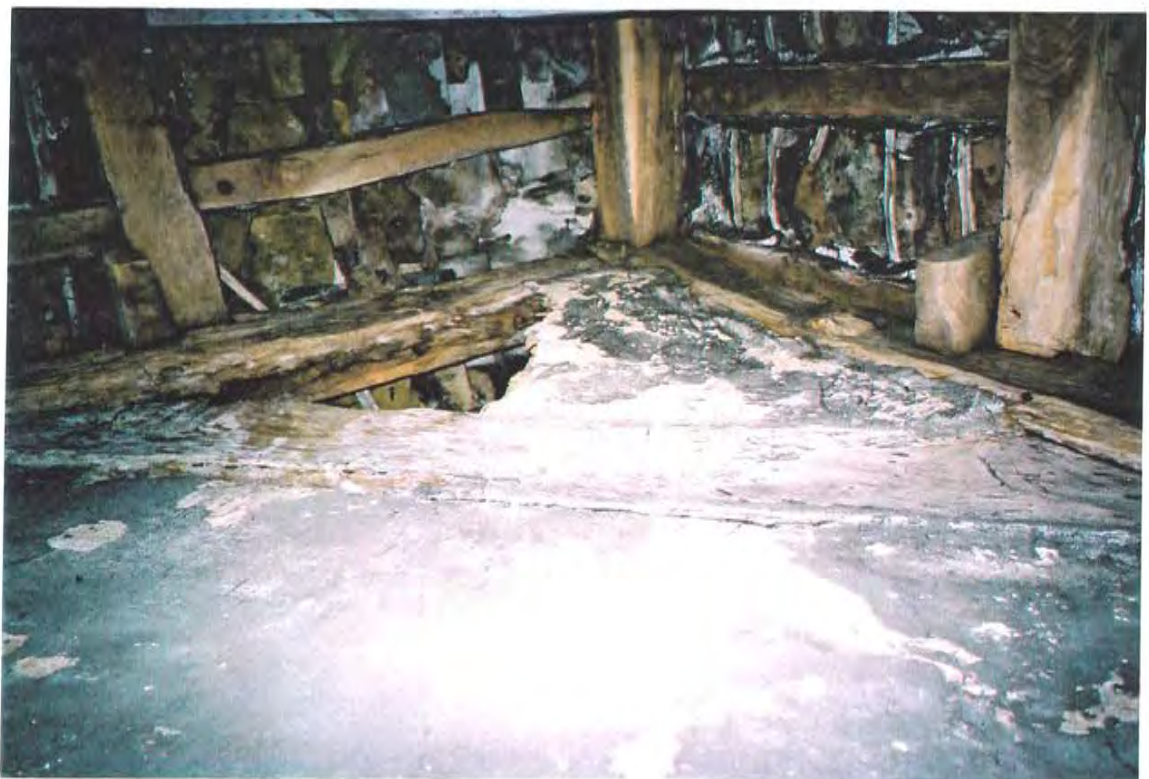
Pl. 16 Detail of roof truss over cross-wing to the farmhouse. The infill is wattle and daub
