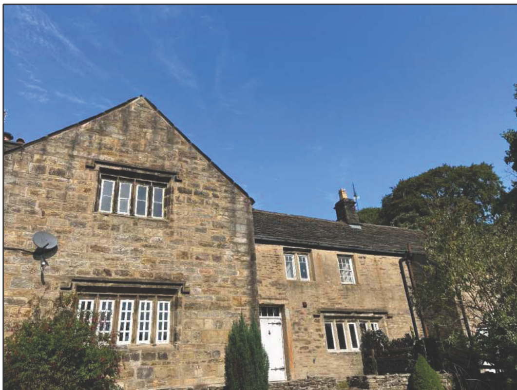
Figure 7: Building 1 located within the centre of the site.
