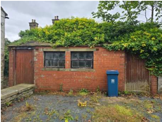
Figure 38: Exterior of the brick-built outbuilding
