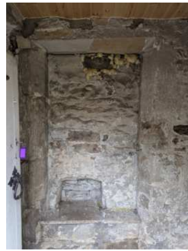
Figure 37 Internal shot of the stair turret
