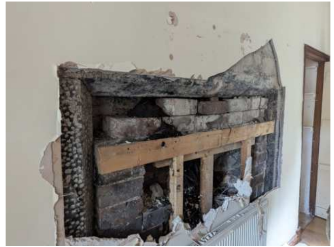
Figure 35 View of the blocked fireplace in the kitchen
