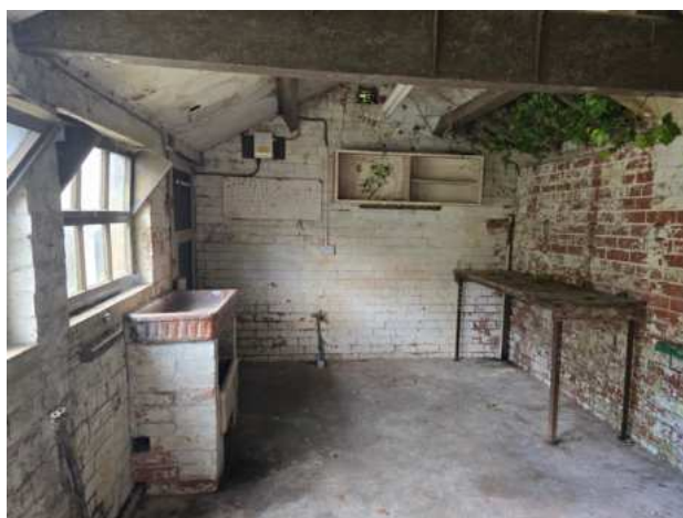
Figure 40: Interior of the brick-built outbuilding
