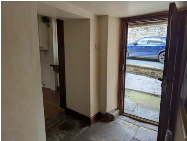
Figure 25 View of the through passage
