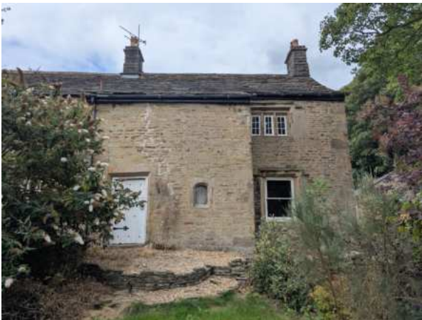
Figure 19 View of the principal elevation
