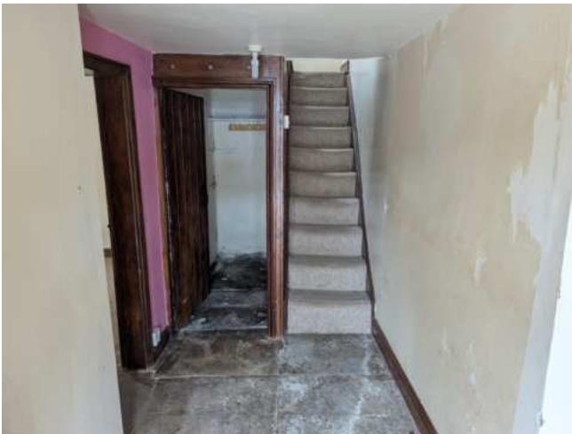
Figure 24 View of the through passage
