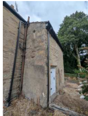
Figure 20 View of the projecting stair turret
