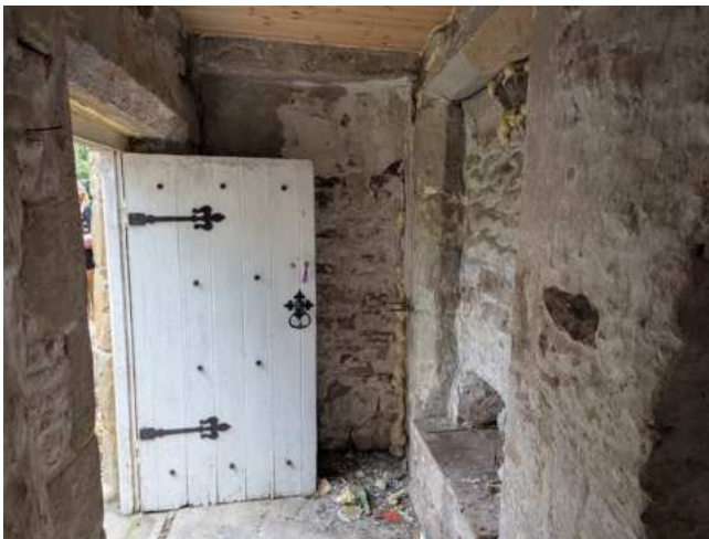
Figure 36 Internal shot of the stair turret
