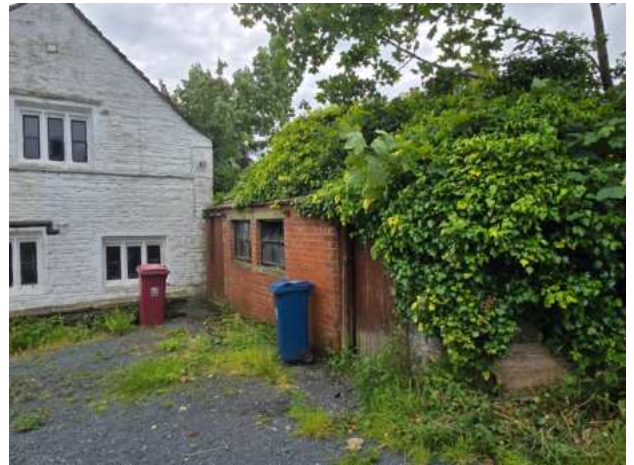
Figure 39: Exterior of the brick-built outbuilding
