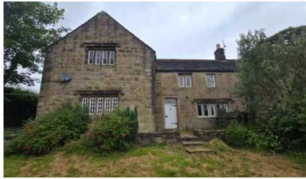
Figure 2: Principal south facing elevation of Cockshutts Farmhouse
