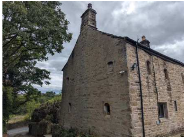
Figure 18 View of the east facing elevation
