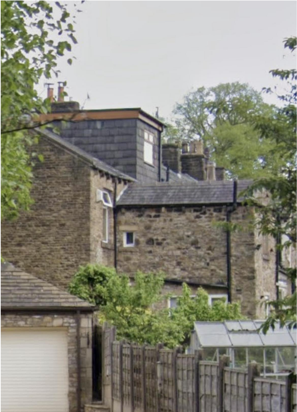
IMAGE SHOWING THE SIDE OF N06 CLITHEROE ROAD DORMER AND OUTRIGGER ROOF ALTERATION TO DEMONSTRATE THE OBSCURING NATURE UPON THE PROPOSED DEVELOPMENT
