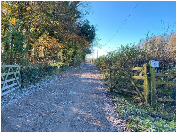
Plate 9: View southwest towards Siddows Farmhouse from the road bordering the northern parcel of the site
