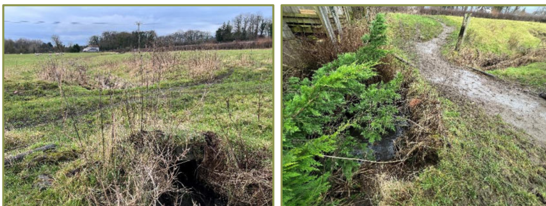
Left: \varnothing 500\text{mm} culvert crossing. Right: \varnothing 700\text{mm} culvert crossing.
