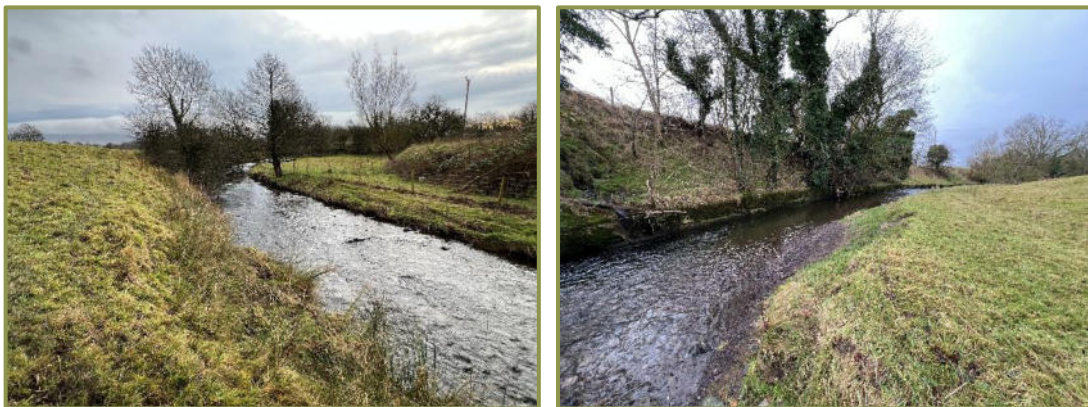
Left: View upstream (east) along Pendleton Brook, along the southern boundary of the eastern parcel. Right: View downstream (west) along Pendleton Brook, along the southern boundary of the eastern parcel.
