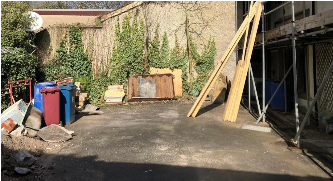
Photo shows the rear yard where the condensers will be located.
