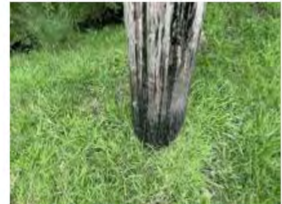
Photo 12— Telephone pole with apparent direct foundation.
