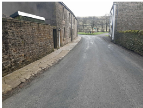
CONCRETE FOOTWAY STARTS IN FRONT OF 7 CHAPEL STREET SLAIDBURN
