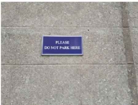
THERE ARE TWO 'PLEASE DO NOT PARK HERE' SIGNS LOCATED BETWEEN 3 CHURCH STREET AND CHAPEL STREET, SLAIDBURN
