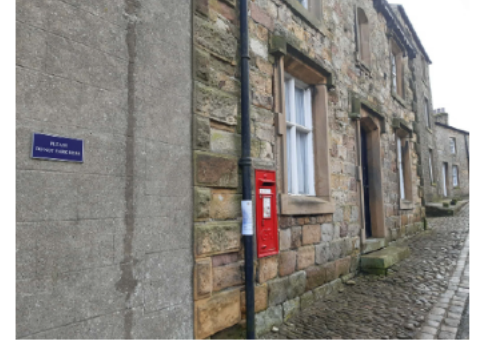
'PLEASE DO NOT PARK HERE' SIGN, LOCATED NEXT TO 3 CHURCH STREET, SLAIDBURN
