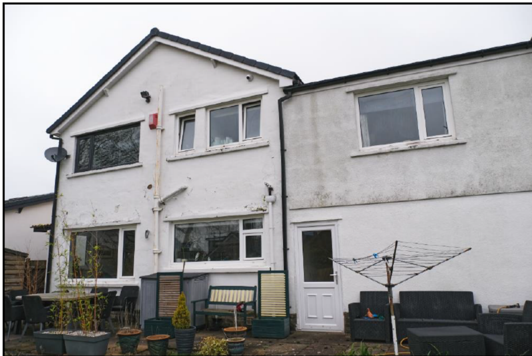
Image showing south (rear) elevation at 57 Edisford Road
