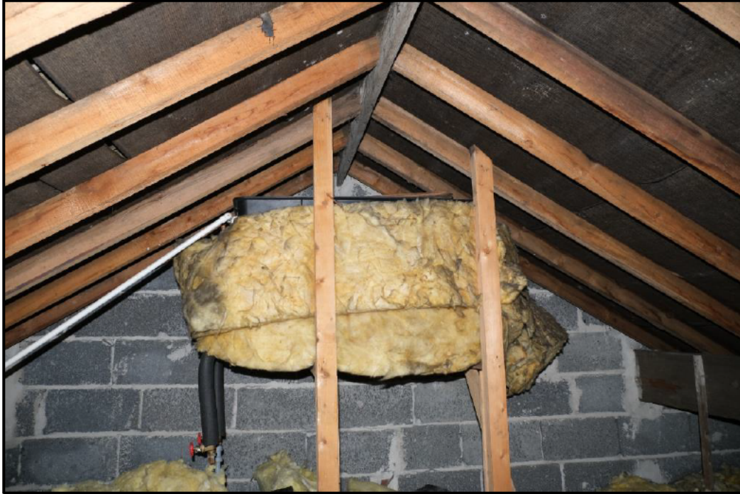
Image showing roof void, no potential access points present
