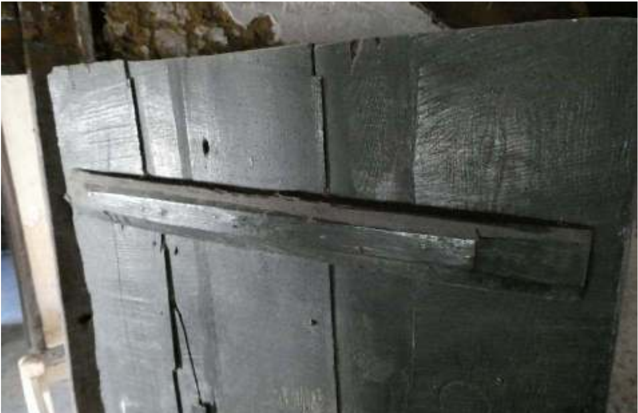
PL43: Western side of planked door.
