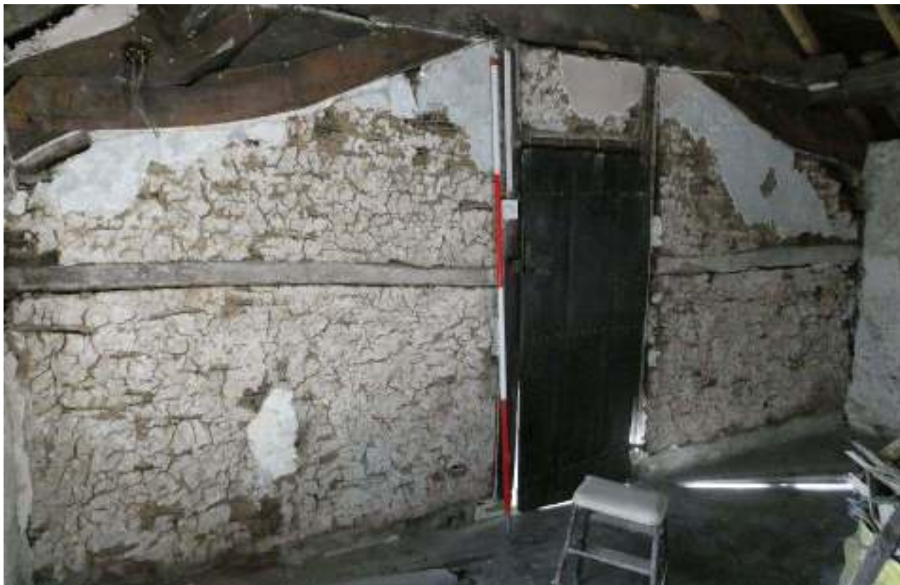
PL29: Central truss, eastern side.
