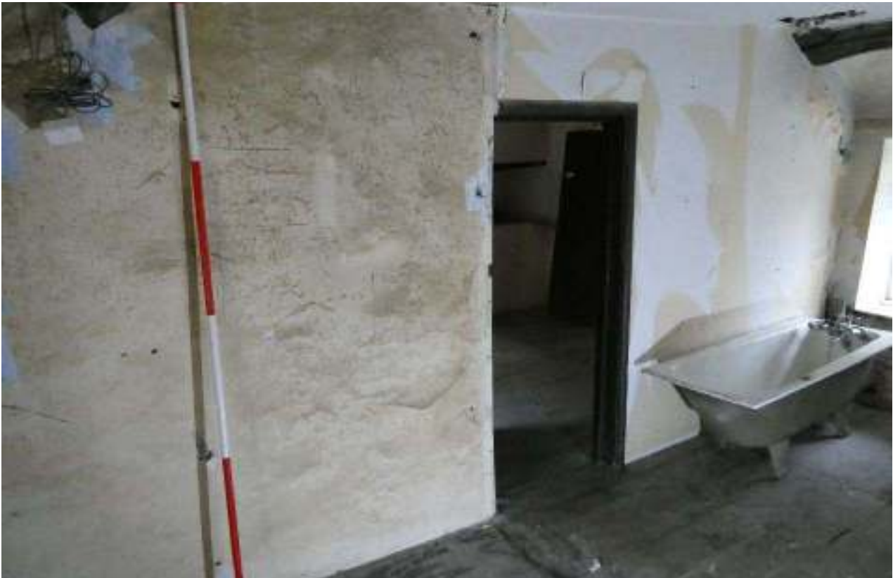
PL47: Central landing area, looking northwest - western truss above.
