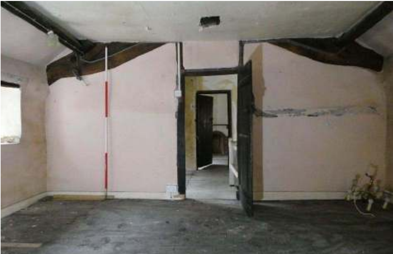
PL27: Central truss, eastern side.
