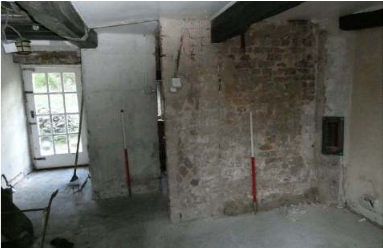
PL59: Ground floor lobby area.
