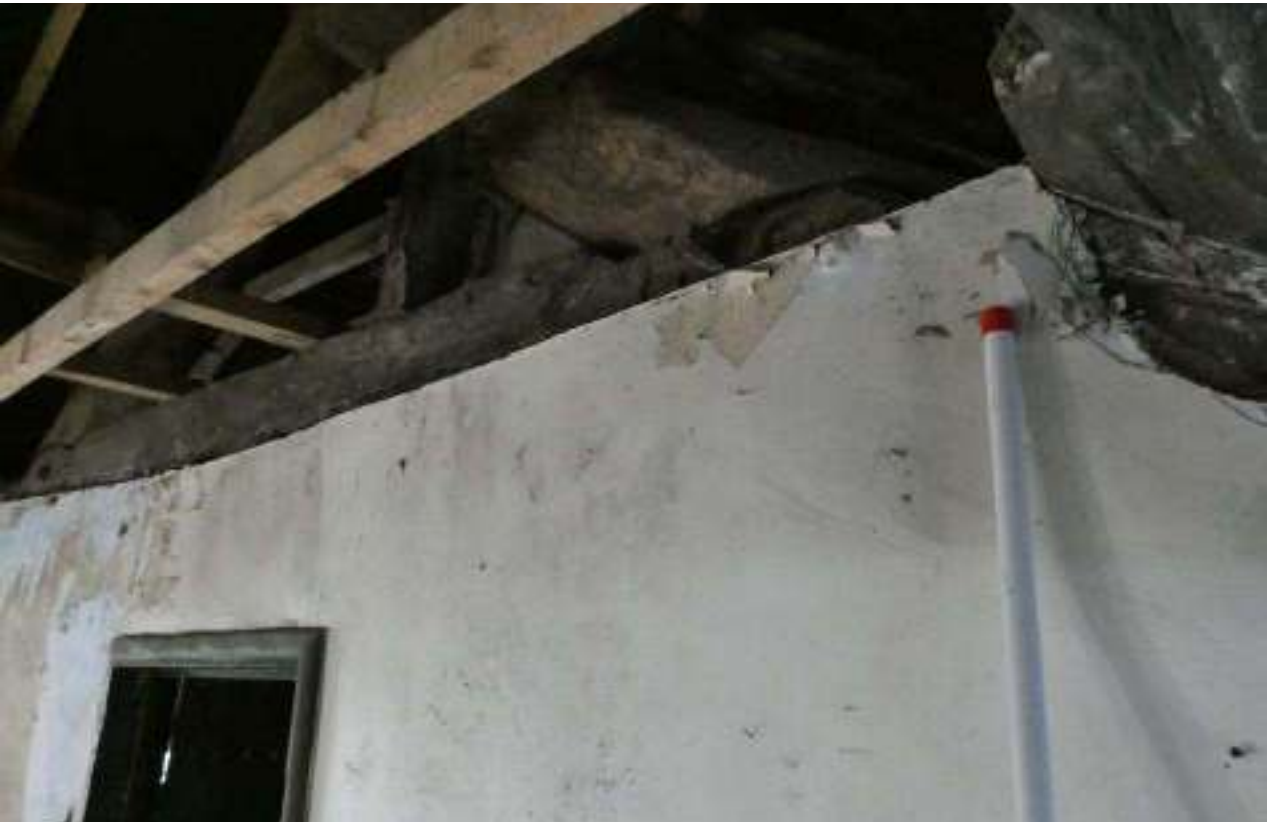
PL51: Western truss, western side.
