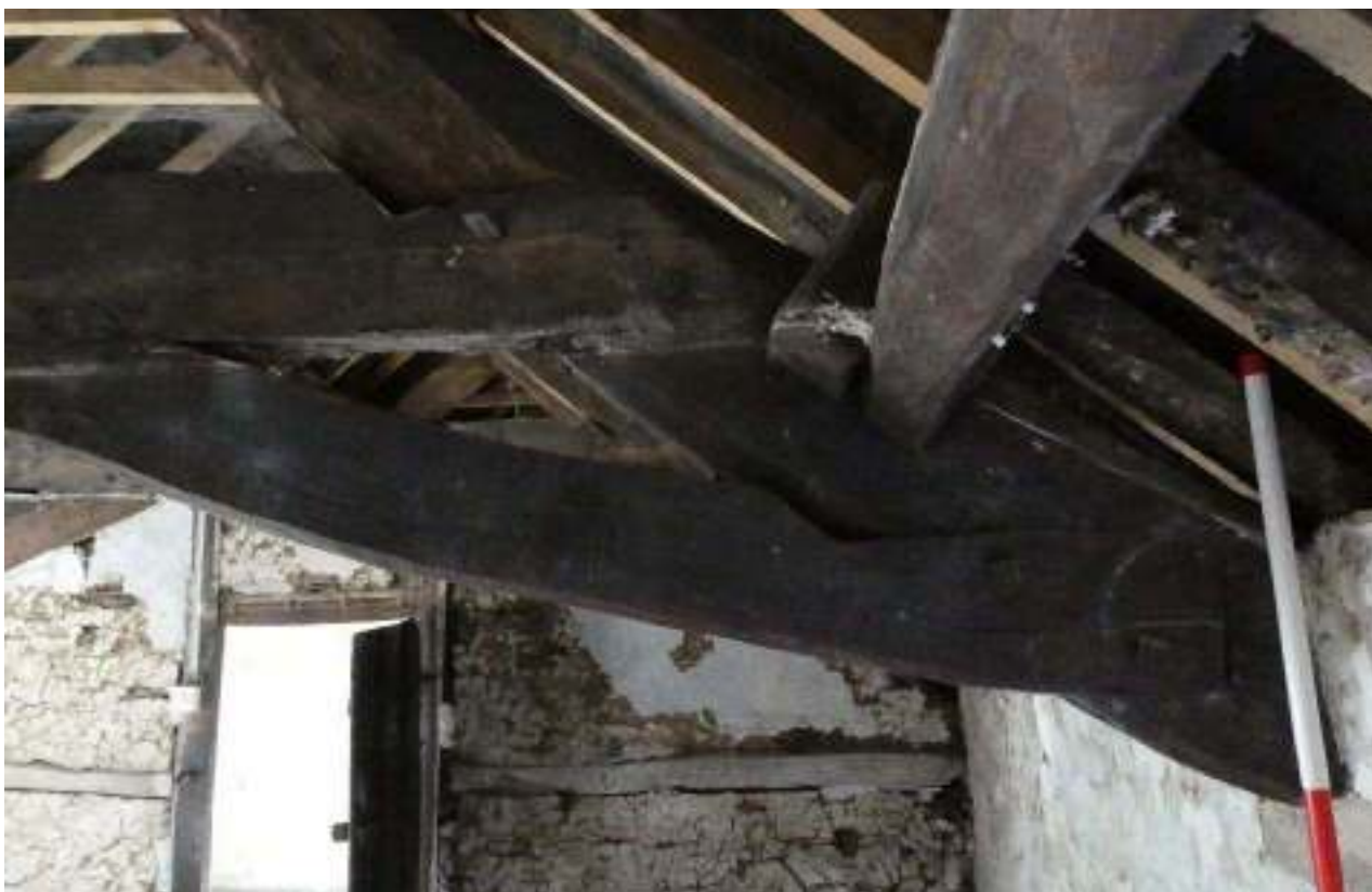
PL20: Eastern truss, eastern side, northern junction of principal rafter, arch brace and tie beam.
