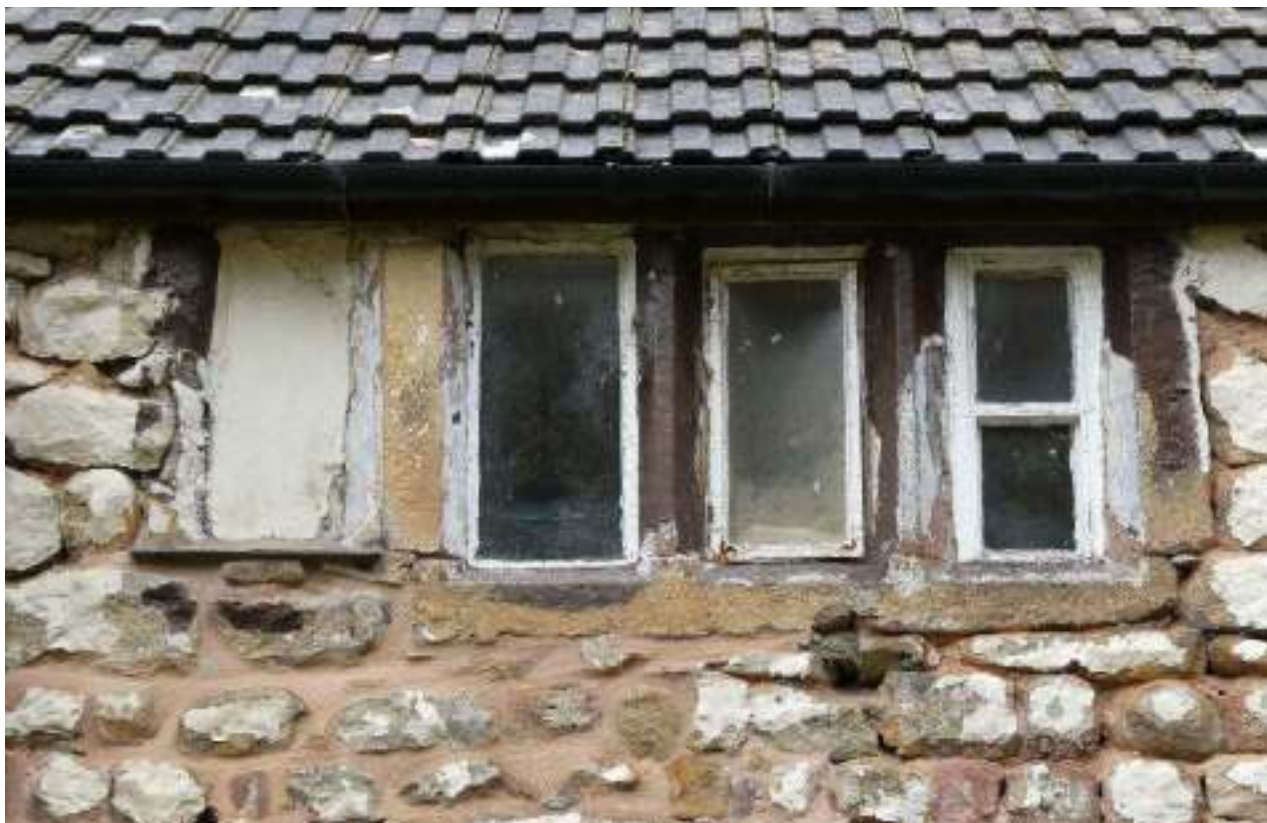
PL10: Southern elevation, first floor - central window.
