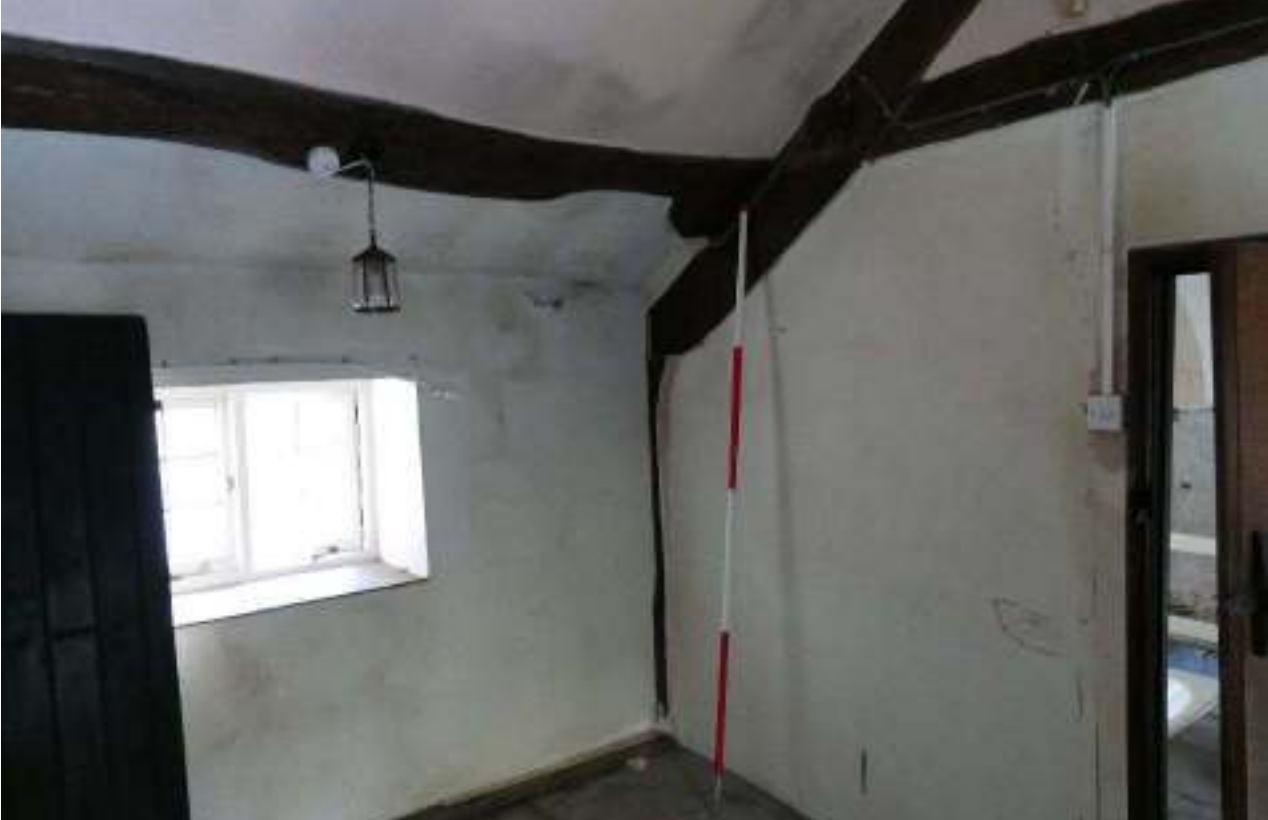
PL46: Central landing area, looking southwest.
