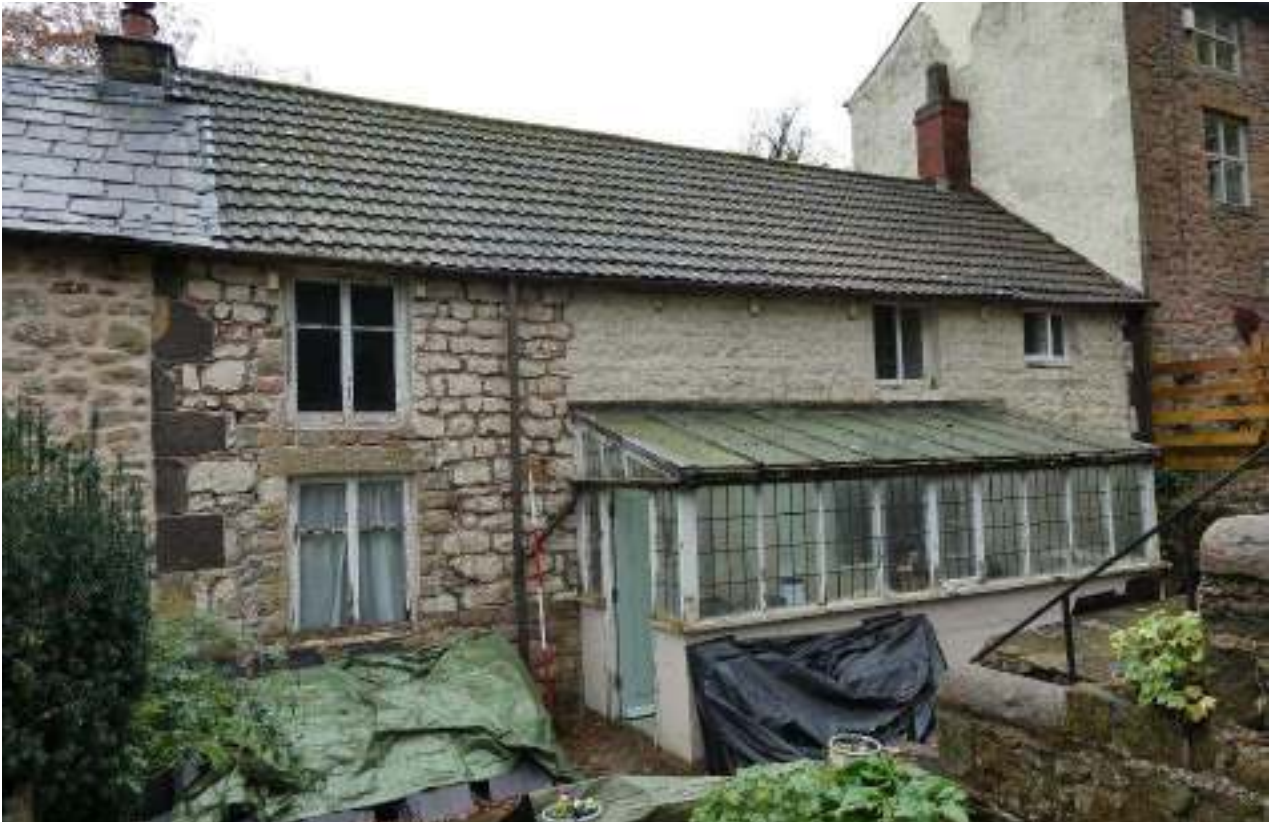
PL01: Northern elevation prior to the demolition of conservatory.
