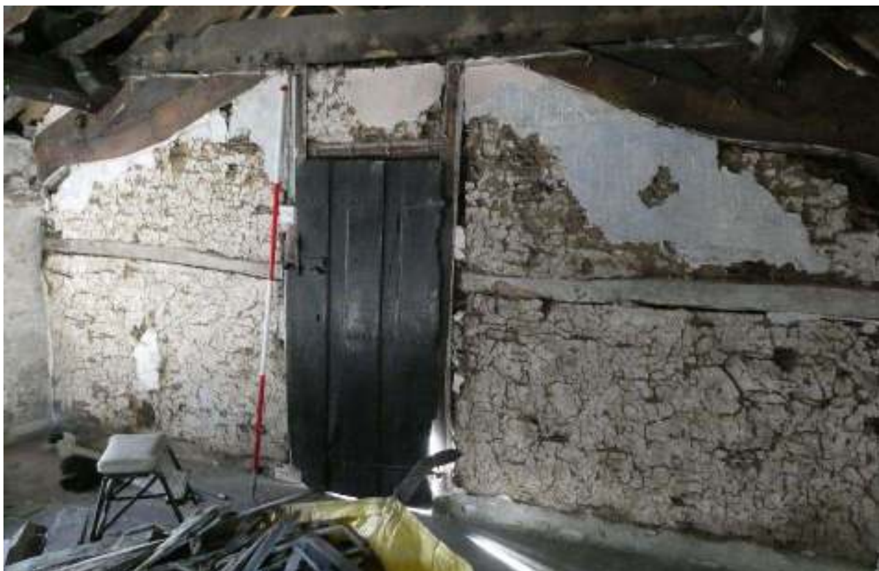
PL30: Central truss, eastern side.
