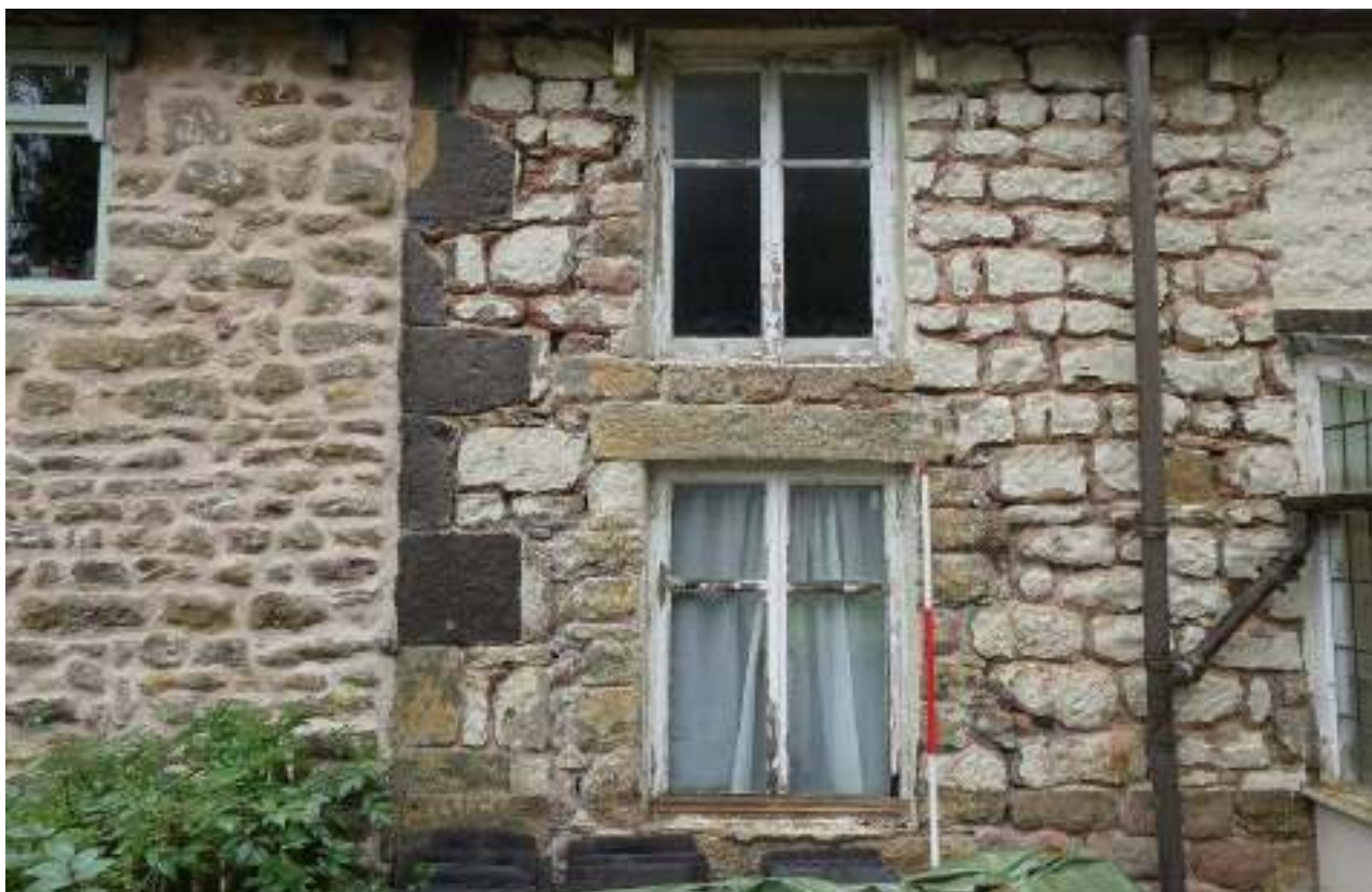
PL04: As above, first bay windows - likely altered.
