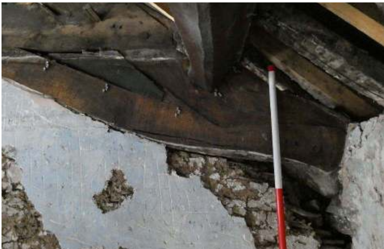
PL32: Central truss, eastern side - northern junction of principal rafter, arch brace and tie beam.
