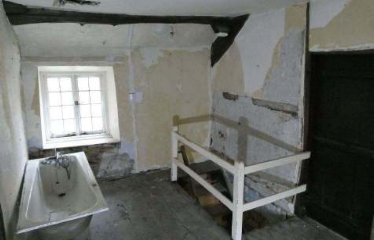
PL44: Central landing area, looking north.
