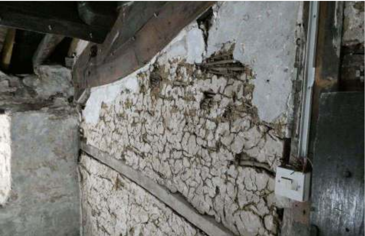
PL33: Eastern side, southern end of wattle and daub wall below central truss.
