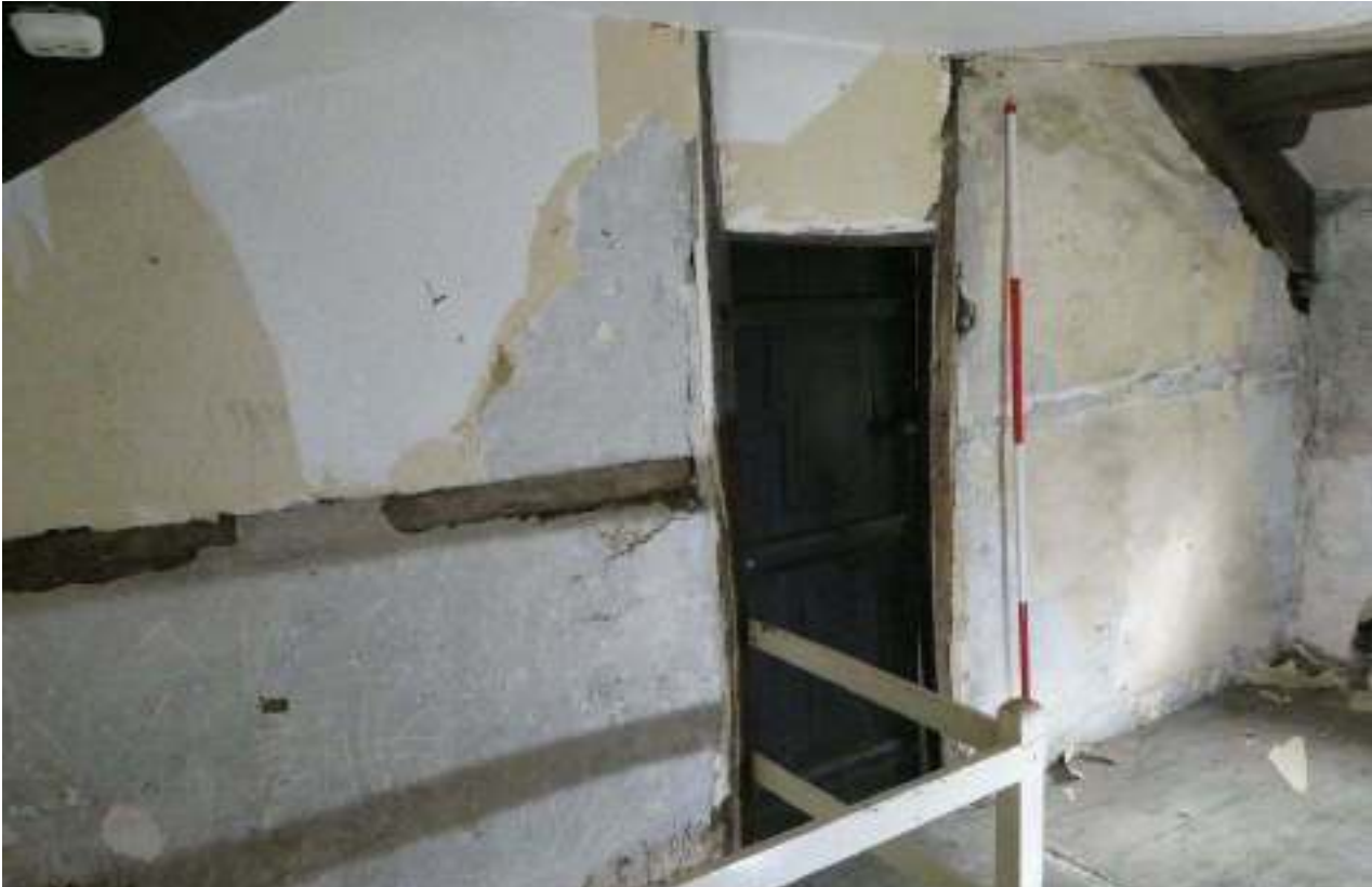
PL39: Central truss and wattle wall, western side.
