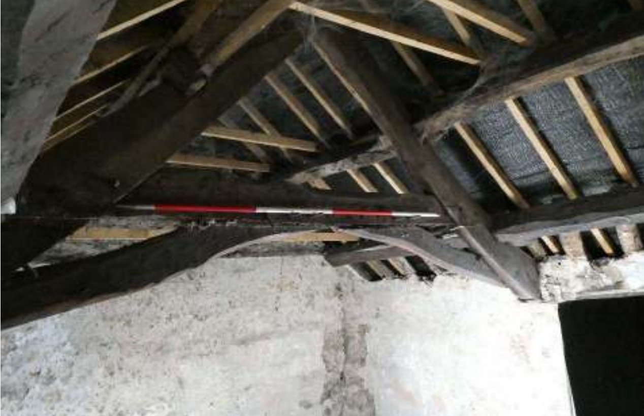
PL22: Eastern truss, western side.
