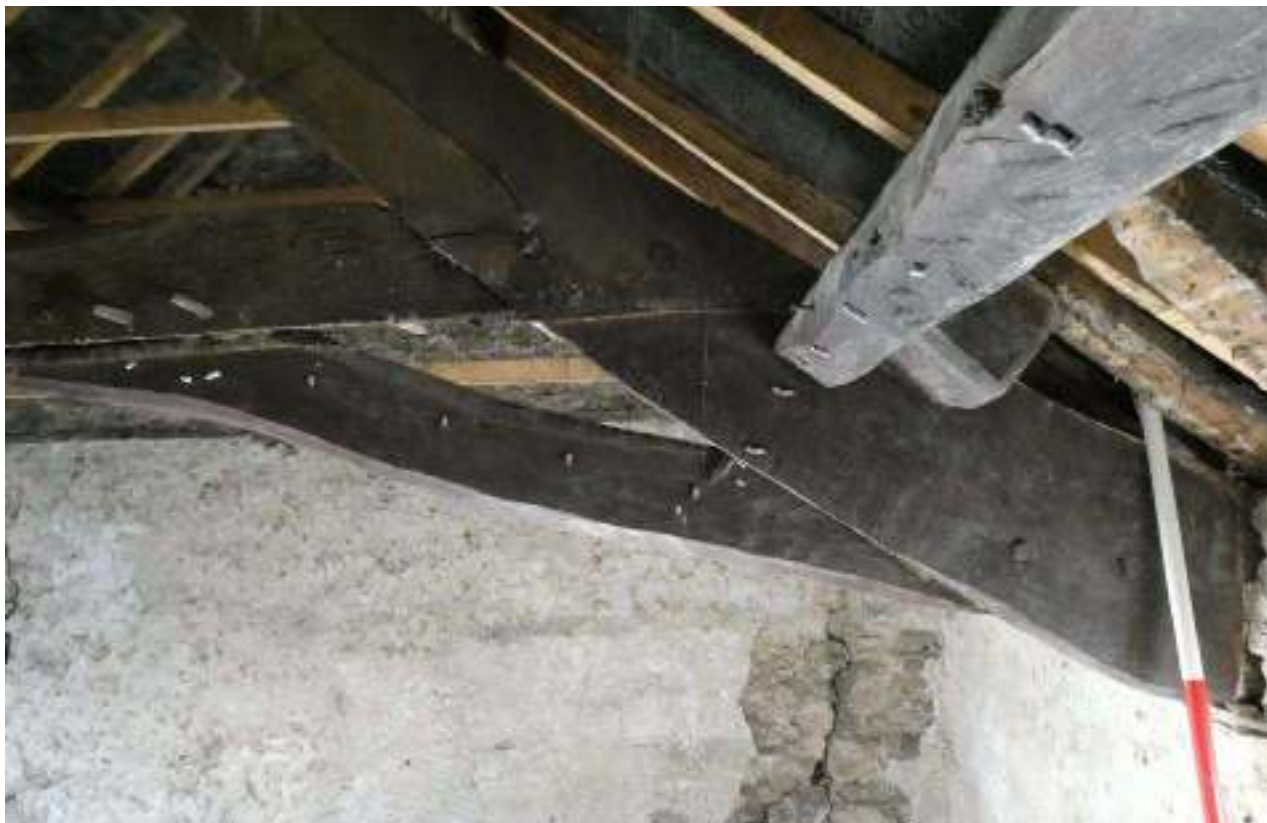
PL23: Eastern truss, western side, southern bearing.
