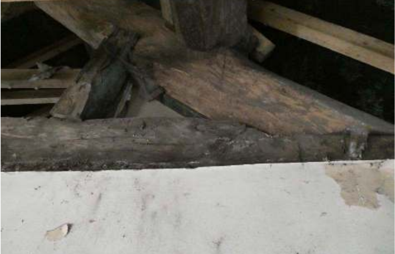
PL50: Western truss, western side, southern bearing with strutt between the tie beam and principal rafter.
