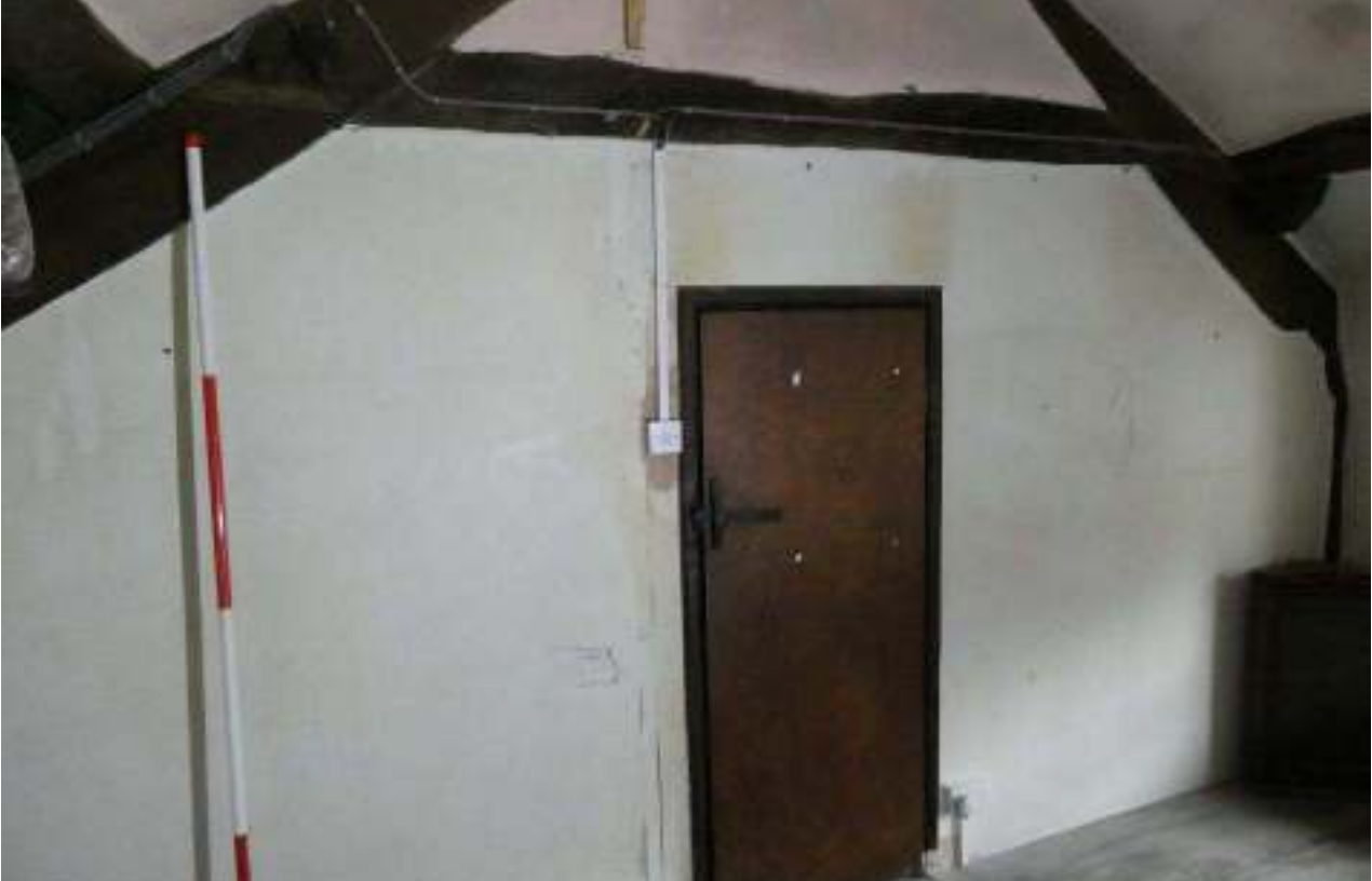
PL48: Western truss, western side.
