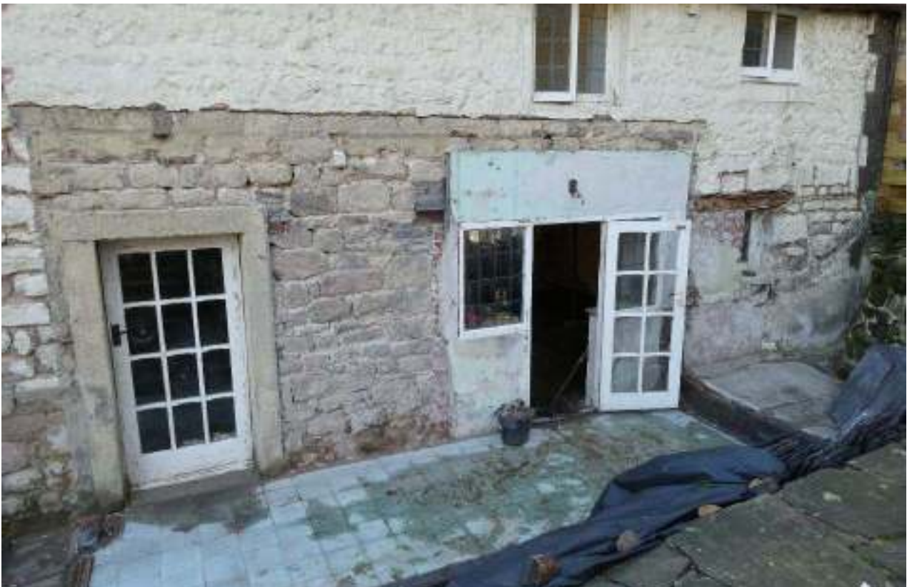
PL02: Northern elevation following the demolition of the conservatory.
