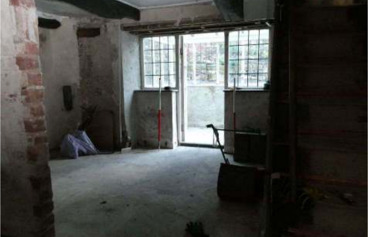
PL58: Ground floor lobby area.
