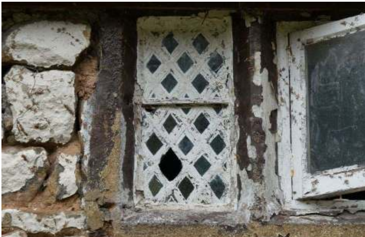
PL09: Southern elevation, first floor - eastern window
