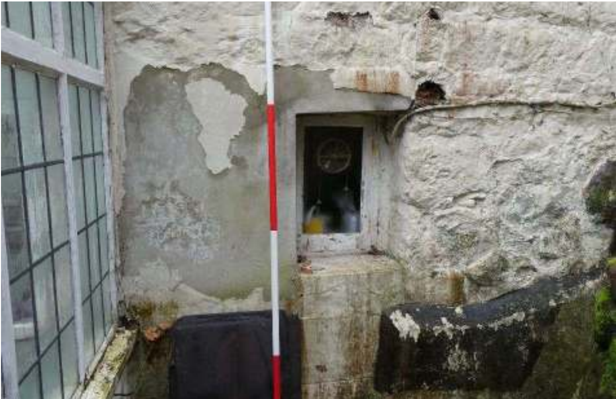
PL05: Northern elevation - infilled window.
