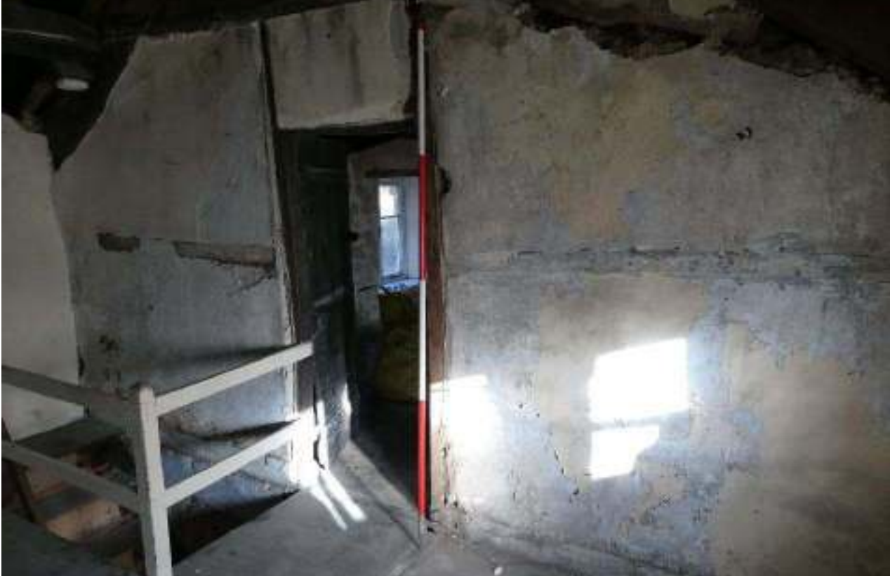
PL40: Central truss and wattle wall, western side.
