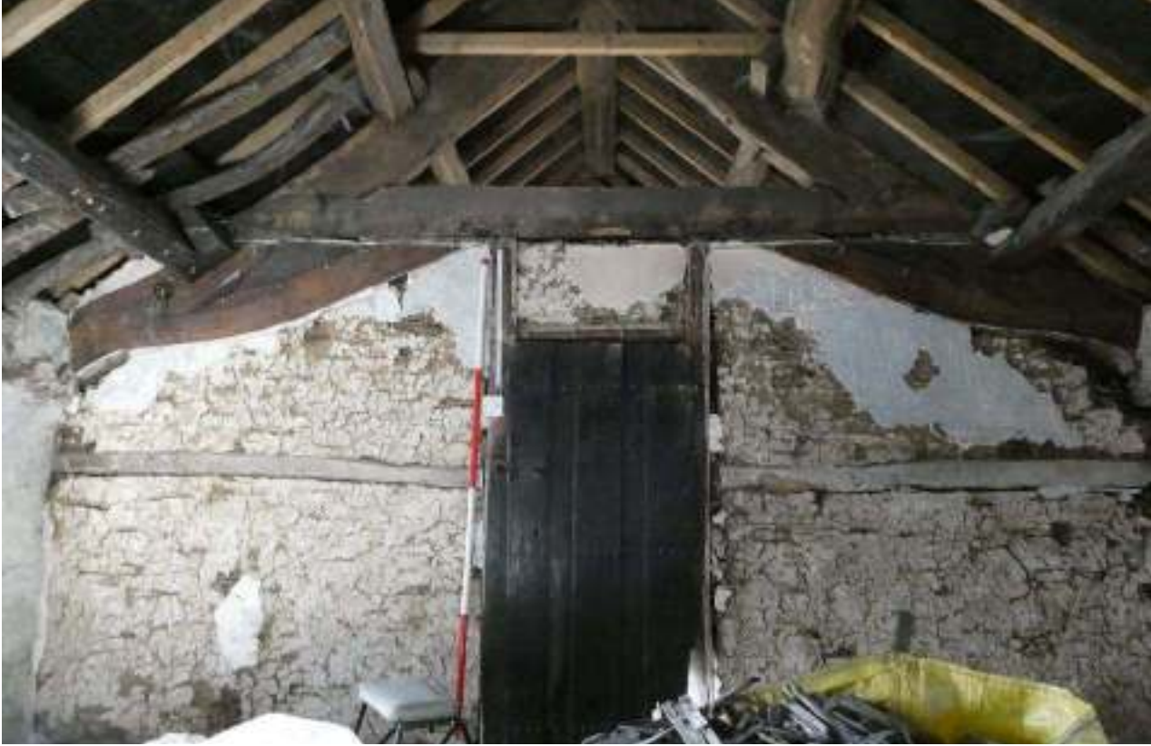
PL28: Central truss, eastern side.
