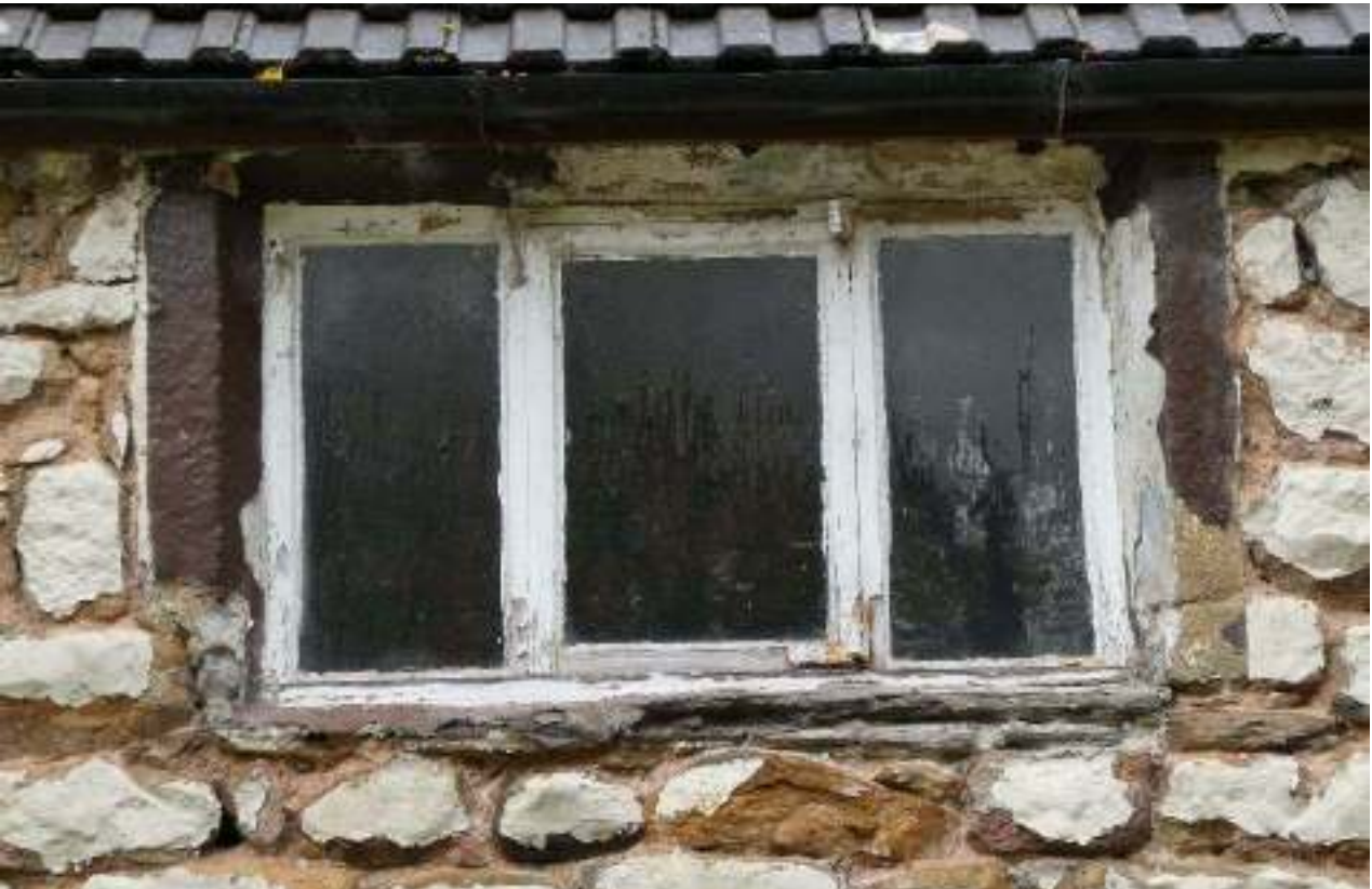
PL11: Southern elevation, first floor - western window.
