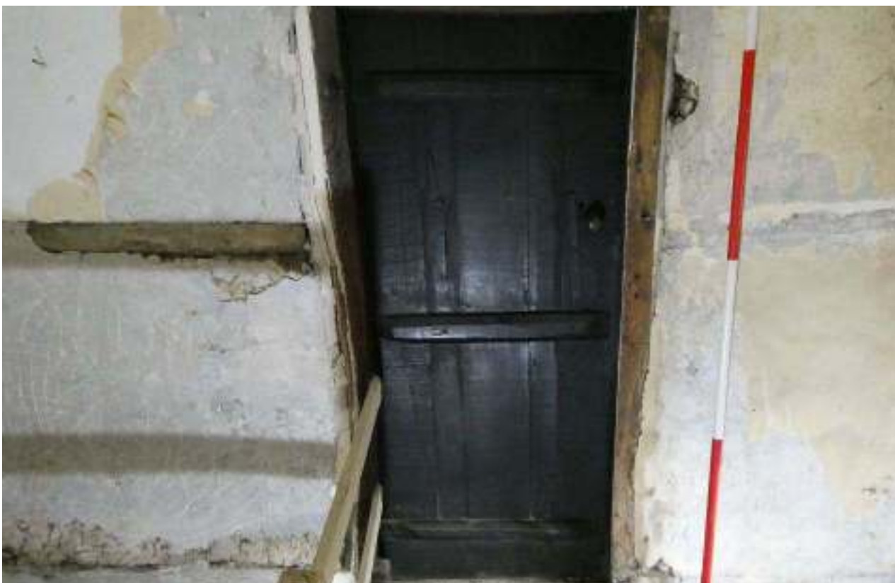
PL42: Western side of planked door.
