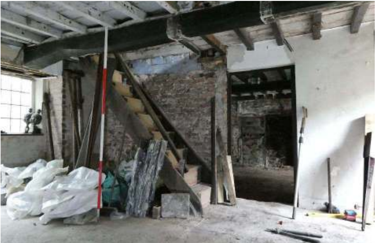
PL61: Ground floor lobby area.
