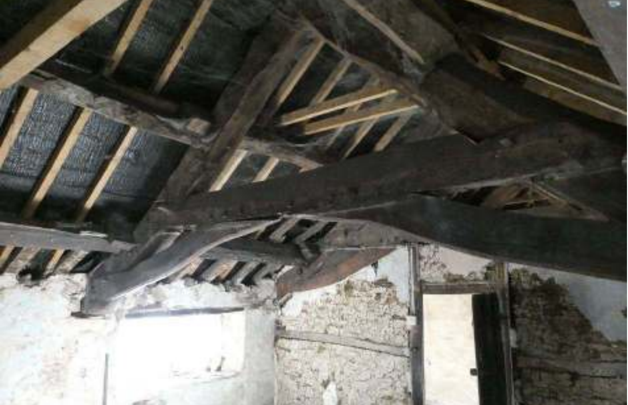
PL18: Eastern truss, eastern side.
