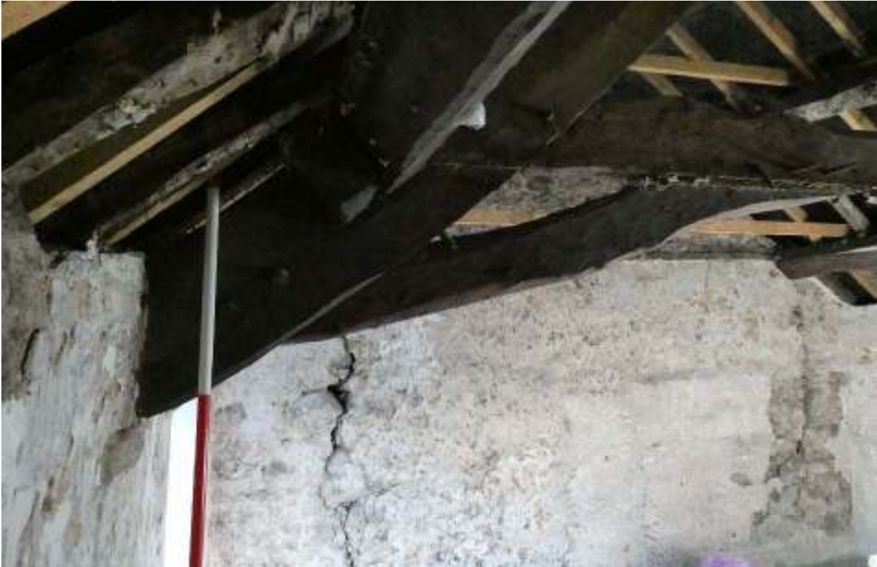
PL21: Eastern truss, western side, northern bearing.
