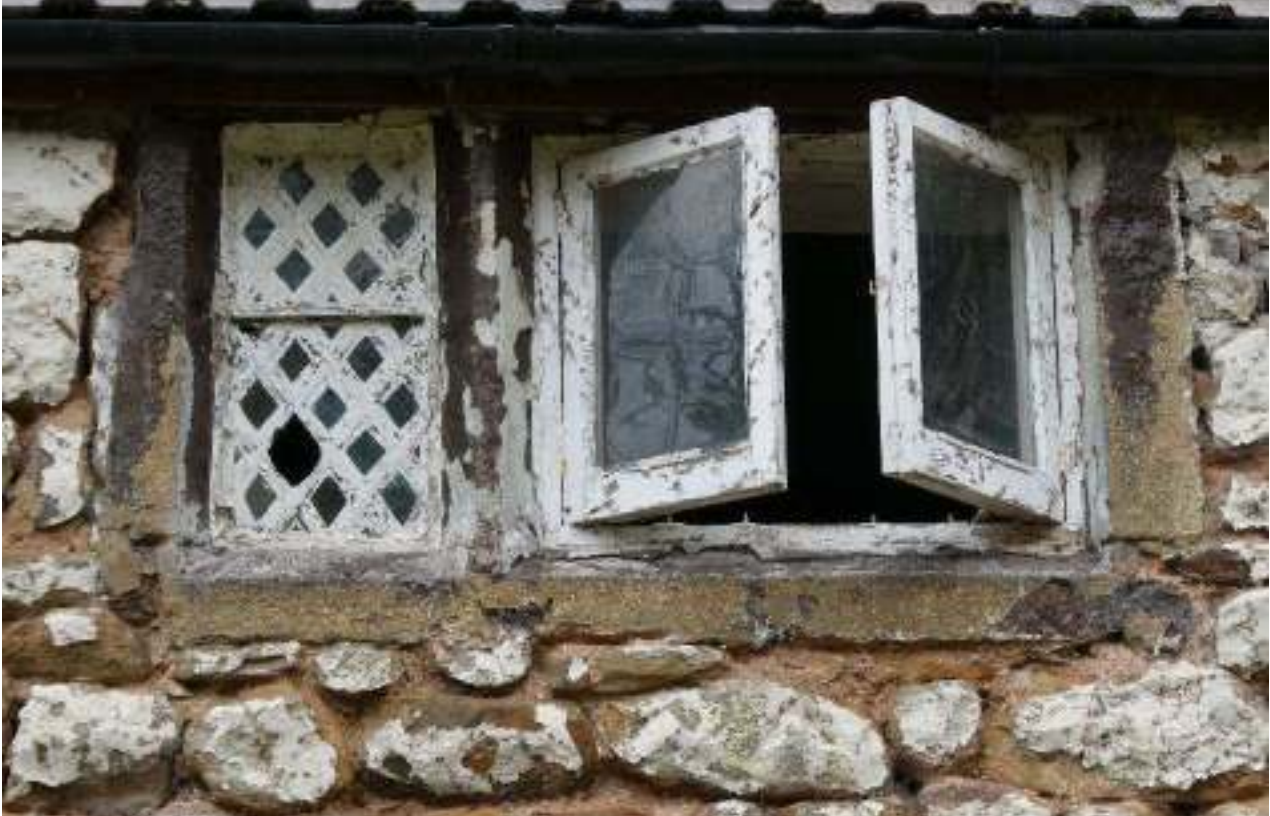
PL08: Southern elevation, first floor - eastern window.
