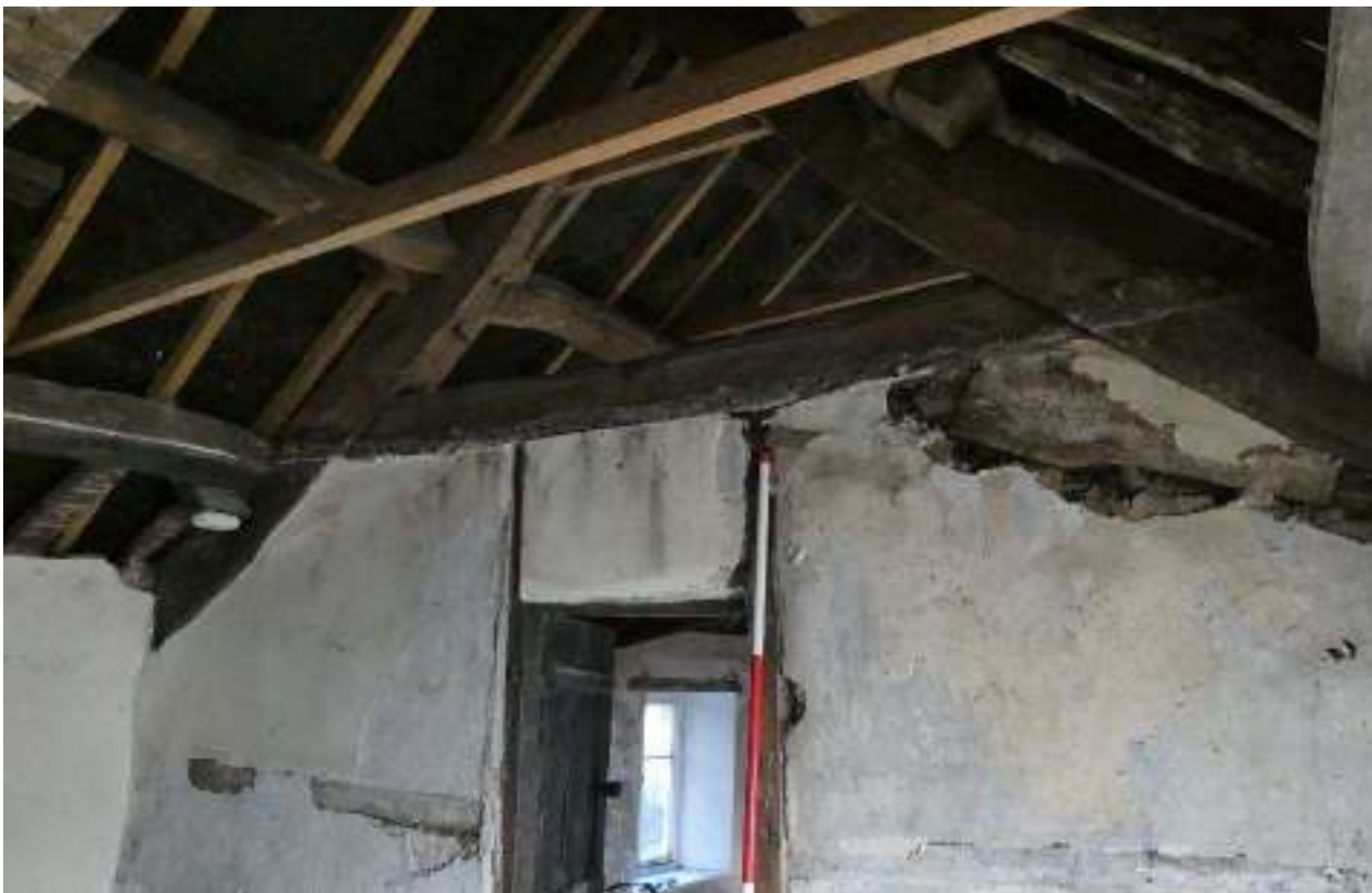
PL41: Central truss and wattle wall, western side.
