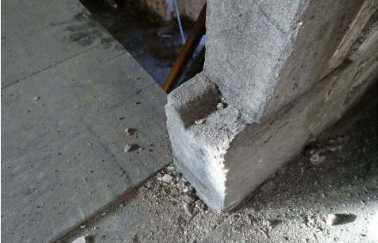
PL38: Grooved cill of wattle wall.
