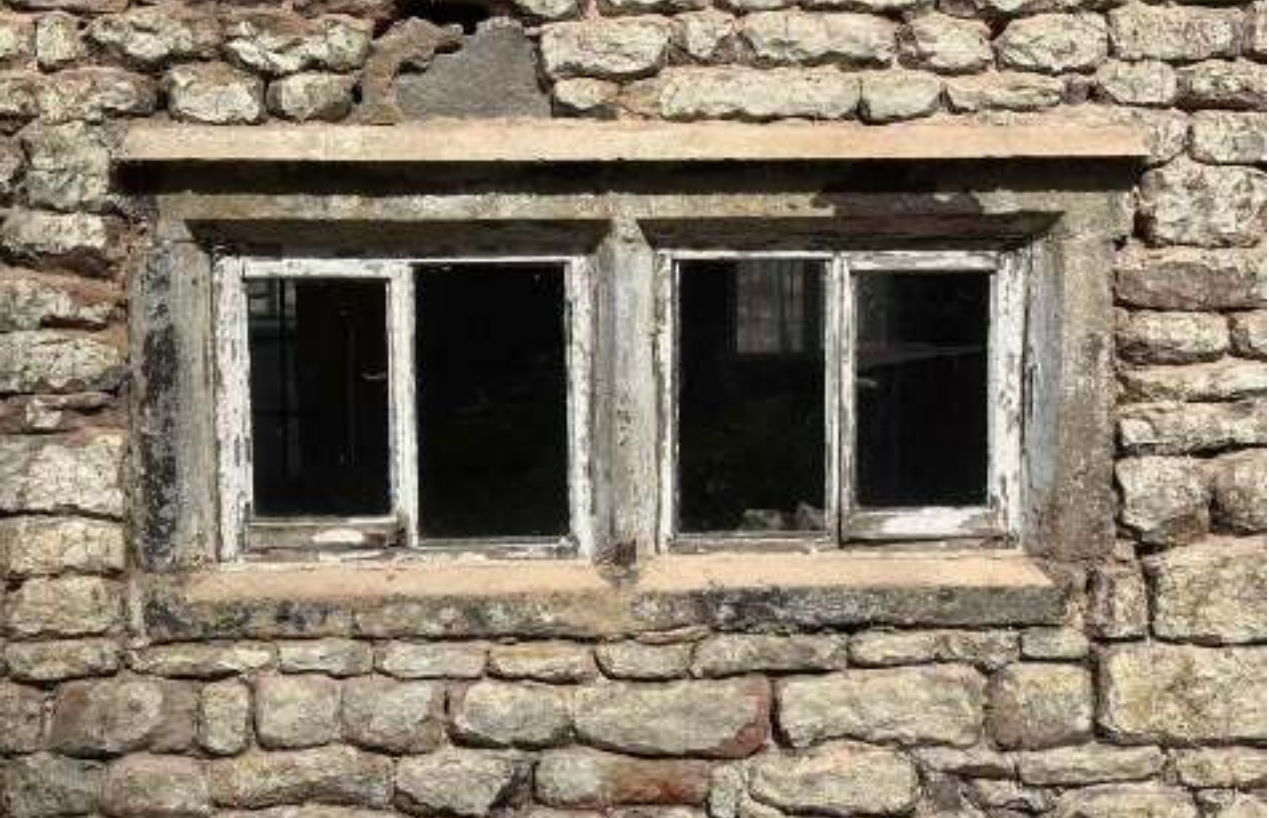
PL12: Southern elevation, ground floor - eastern window.
