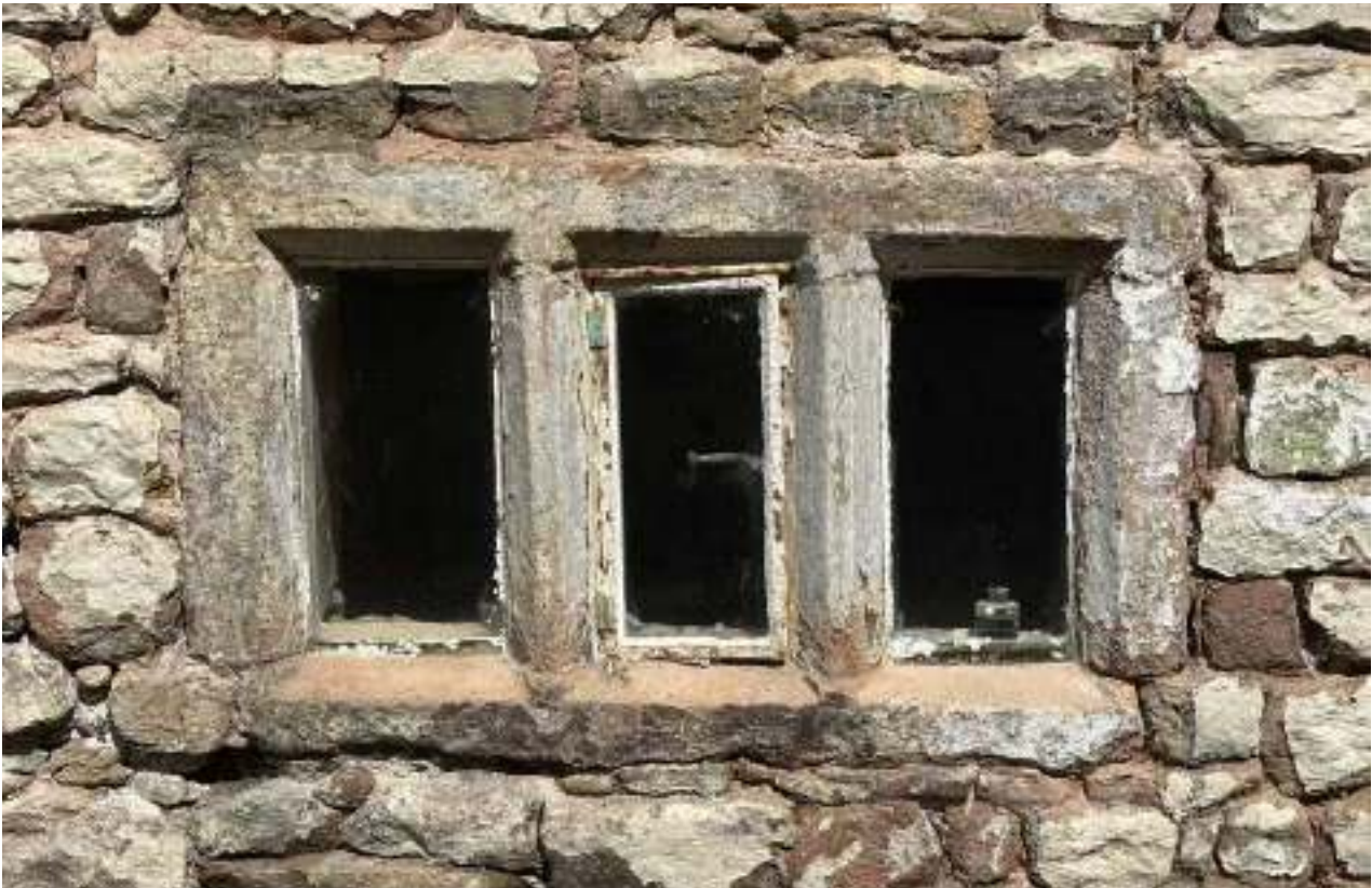
PL15: Southern elevation, ground floor - western window.
