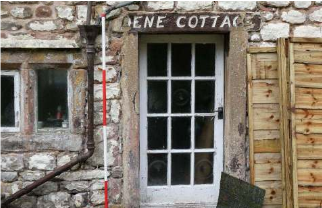
PL13: Southern elevation, ground floor - doorway.
