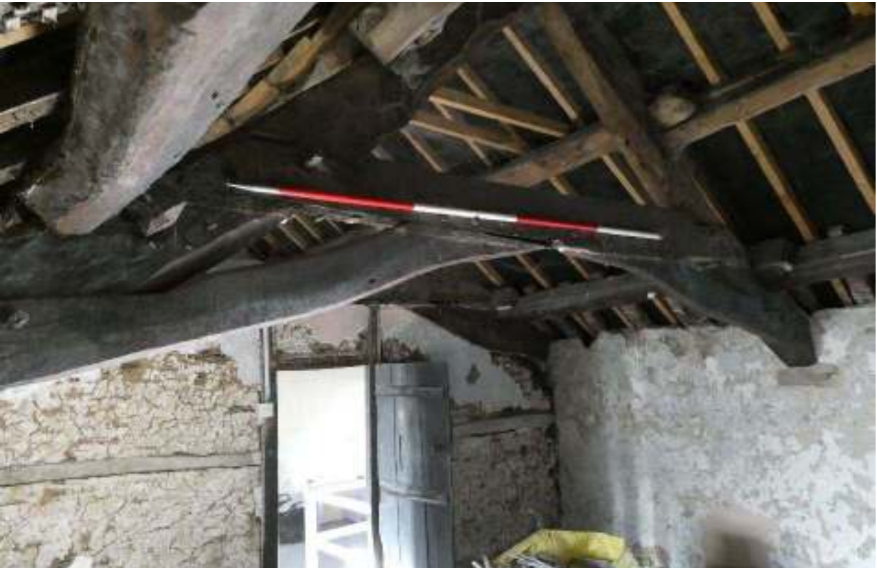
PL17: Eastern truss, eastern side.
