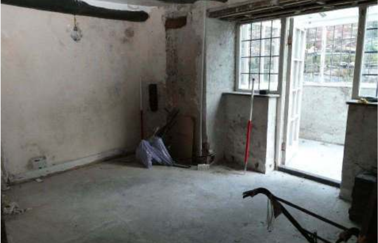
PL60: Ground floor lobby area.
