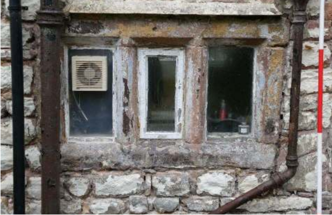
PL14: Southern elevation, ground floor - central window.
