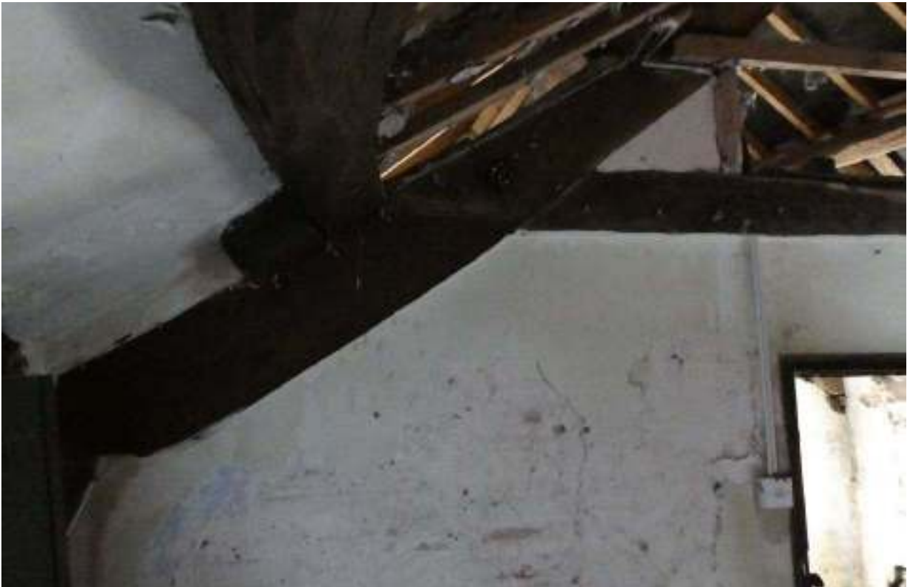
PL49: Western truss, western side, northern bearing.
