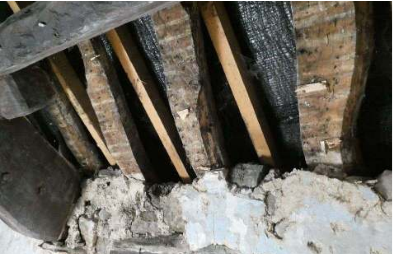
PL25: Remains of original riven rafters at eaves level, eastern bedroom.
