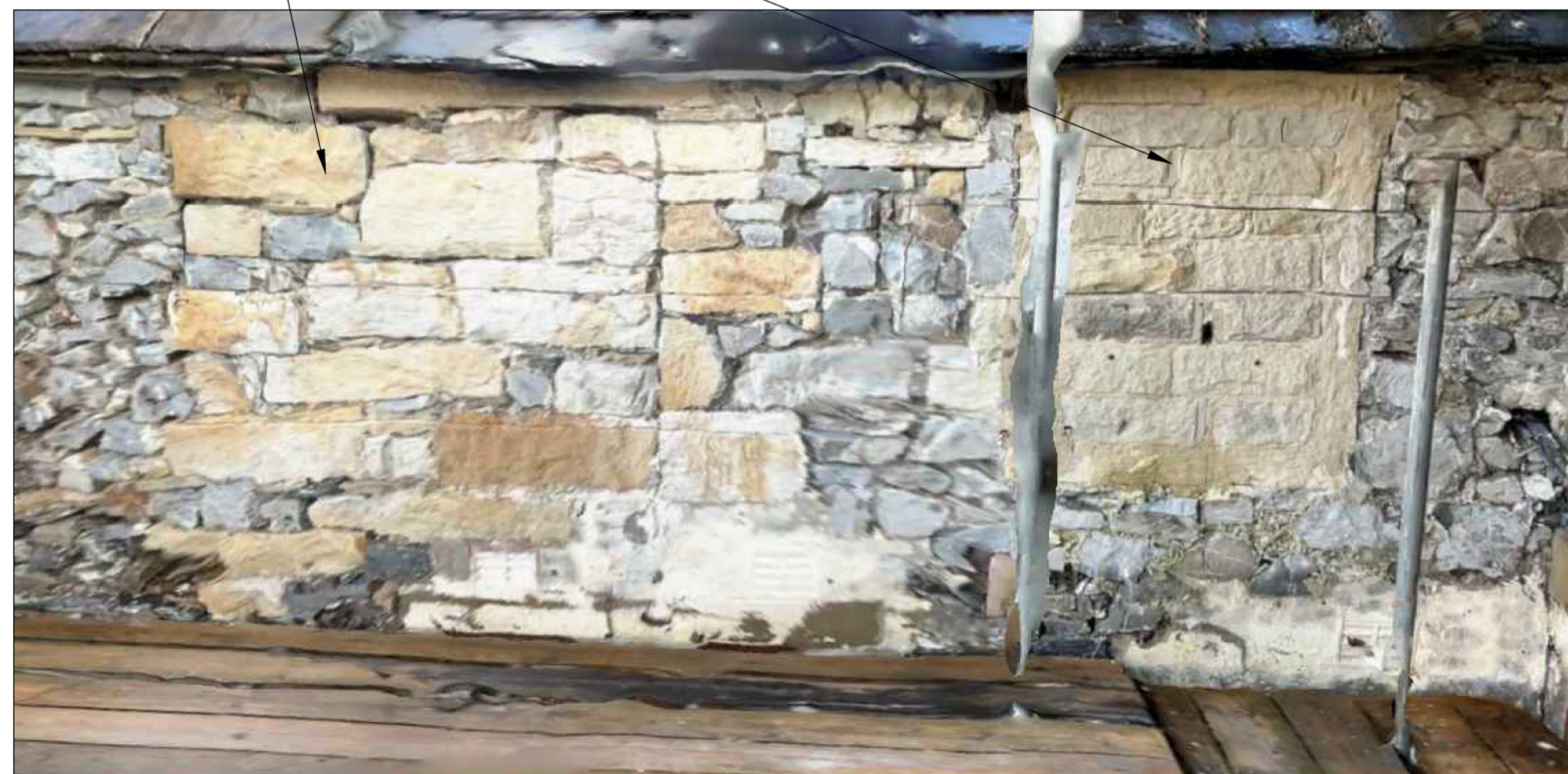
Image of Existing Wall
