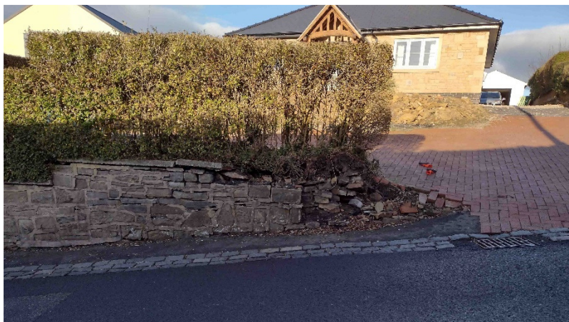
Condition of existing wall January 2026
