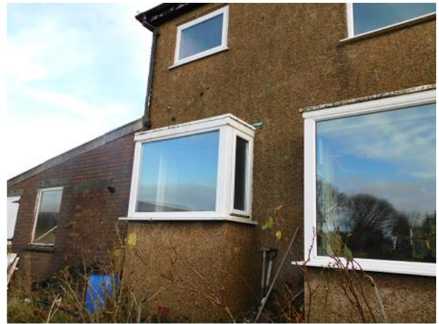
PHOTO 14 South-western View of Kitchen Dormer
