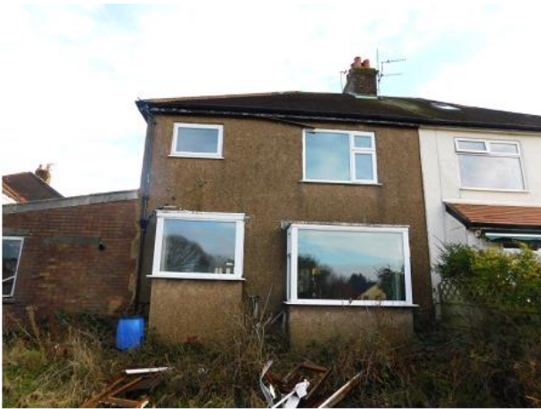
PHOTO 13 Western Elevation of Dwelling
