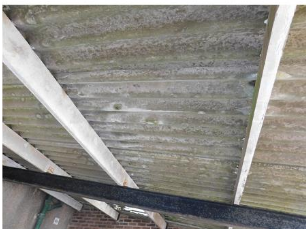
PHOTO 21 Underside of Carport Roof
