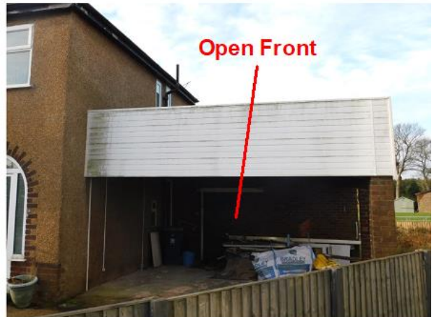
PHOTO 6 Eastern Elevation of Carport
