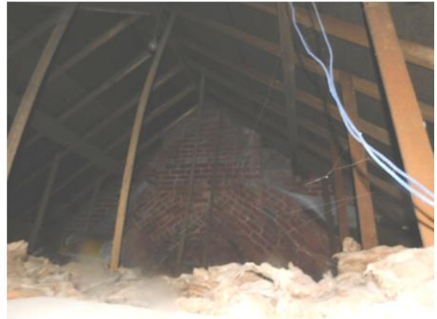
PHOTO 18 Underside of Southern Main Roof
