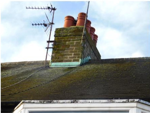
PHOTO 3 View of Eastern Roof
