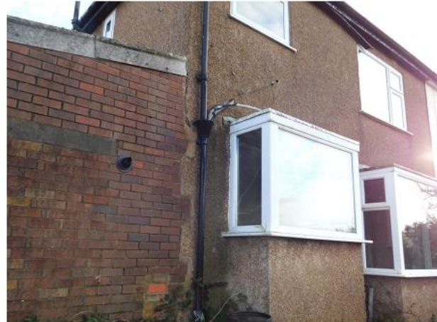
PHOTO 12 North-western Corner of Dwelling
