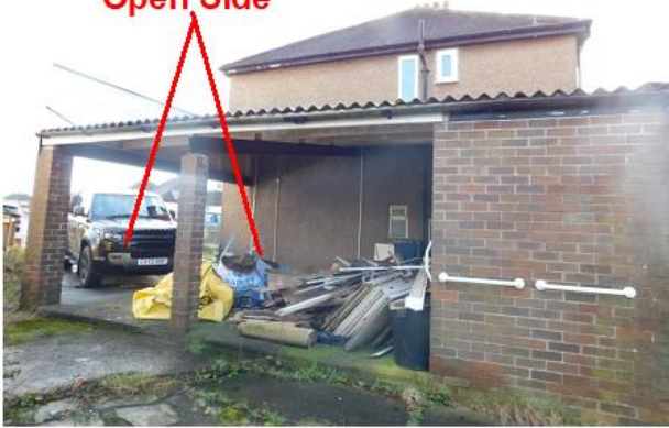
PHOTO 7 Northern Elevation of Carport
