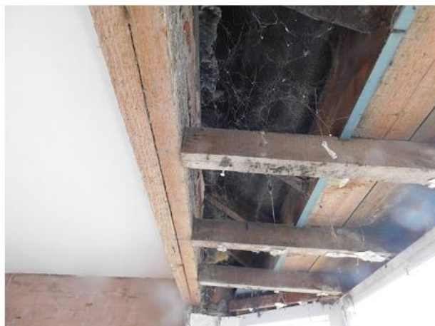
PHOTO 20 Underside of Internal Upper Eastern Dormer
