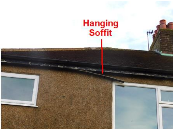
PHOTO 17 View of Western Roof
