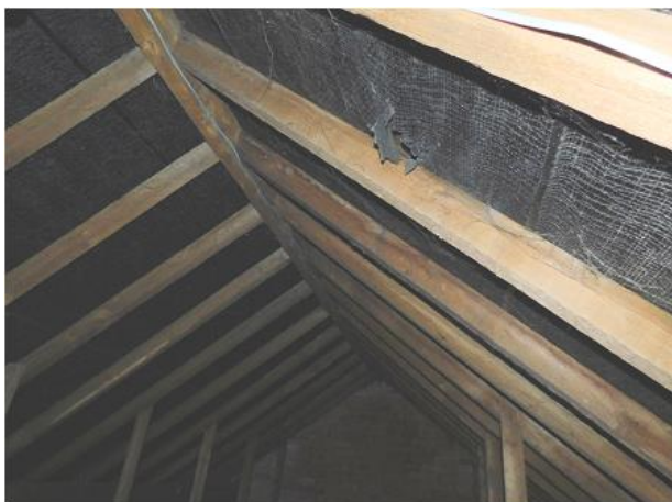
PHOTO 19 Underside of Main Roof
