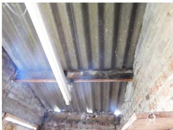
PHOTO 22 Underside of Boiler Room Roof
