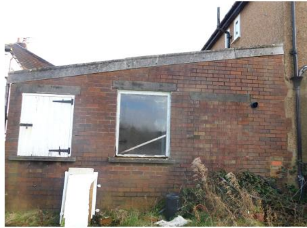
PHOTO 10 Western Elevation of Carport
