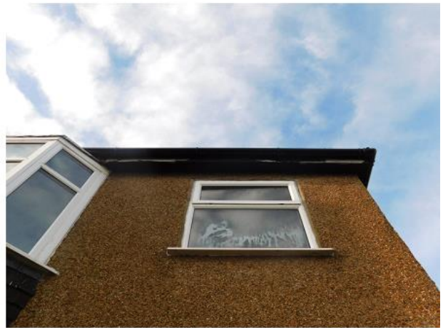
PHOTO 4 Underside of Eastern Soffit
