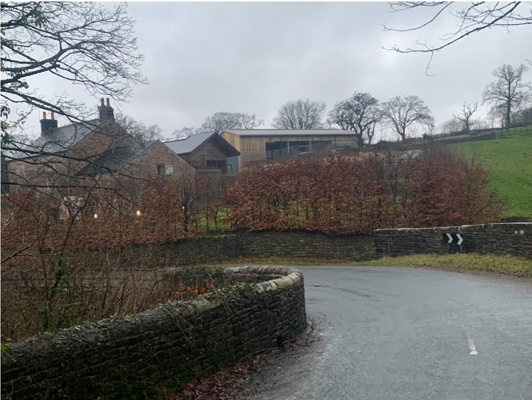
Looking North towards the barns from the road bend, the middle barn is not visible.
