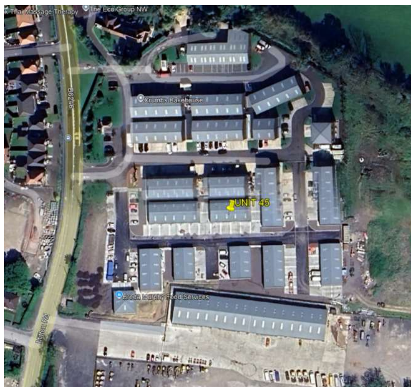
Figure 1: The Site and Wider Context of Mitton Road Business Park
