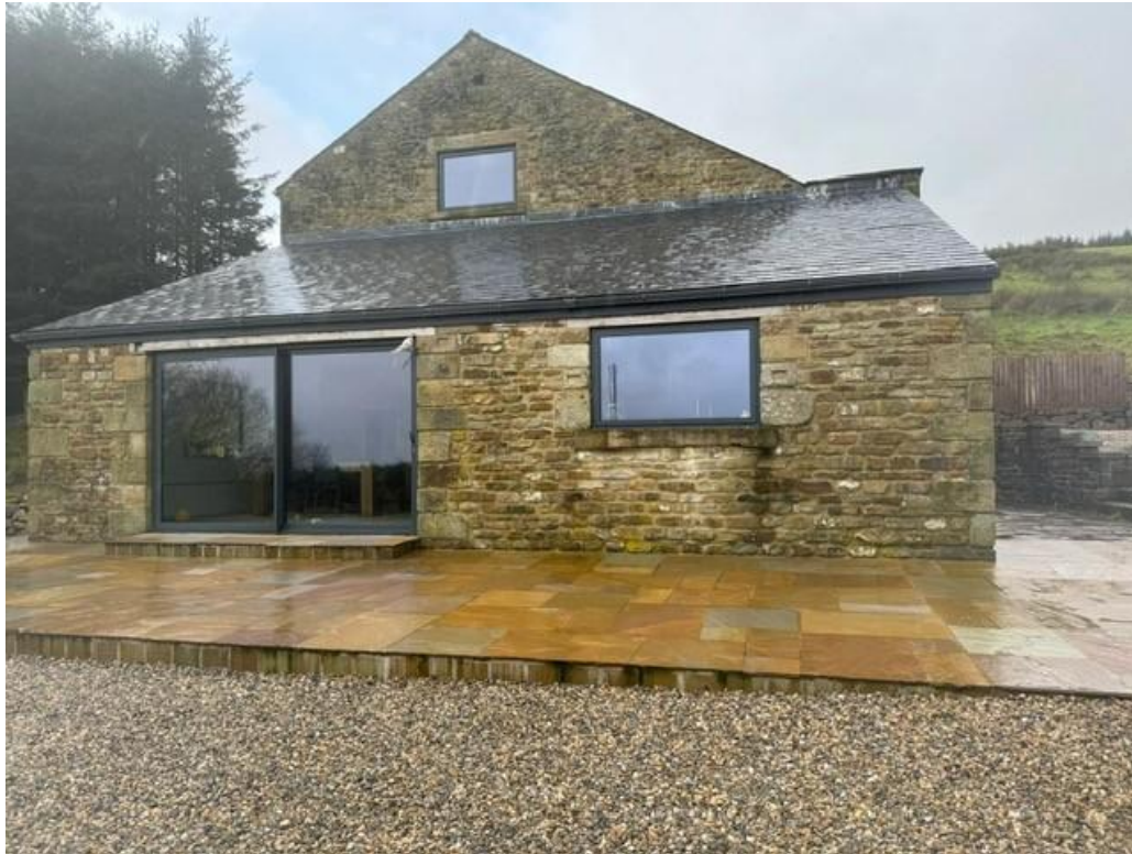
East elevation showing the kitchen extension
