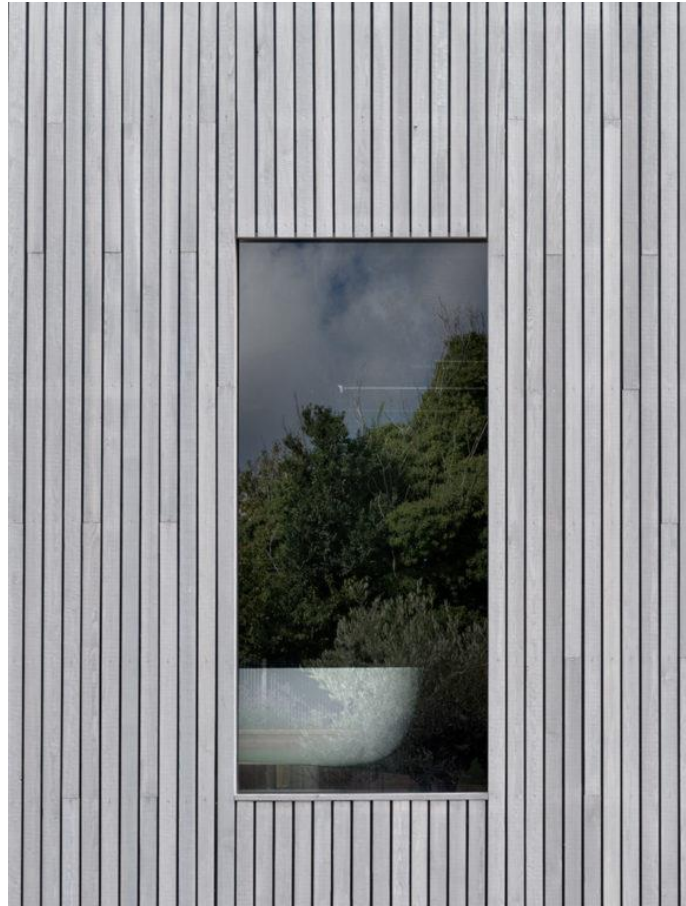
Pl. 7 Photograph showing a silver aged grey larch vertical cladding
