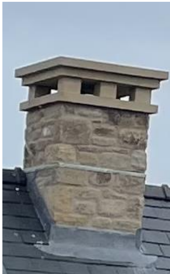
Pl. 5 Photograph showing an example of the stone-built chimney detail
