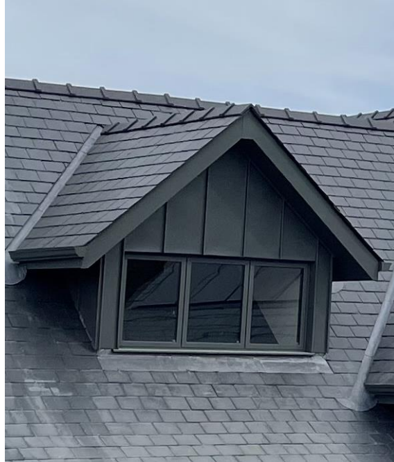
Pl. 2 Example of a dormer roof window
