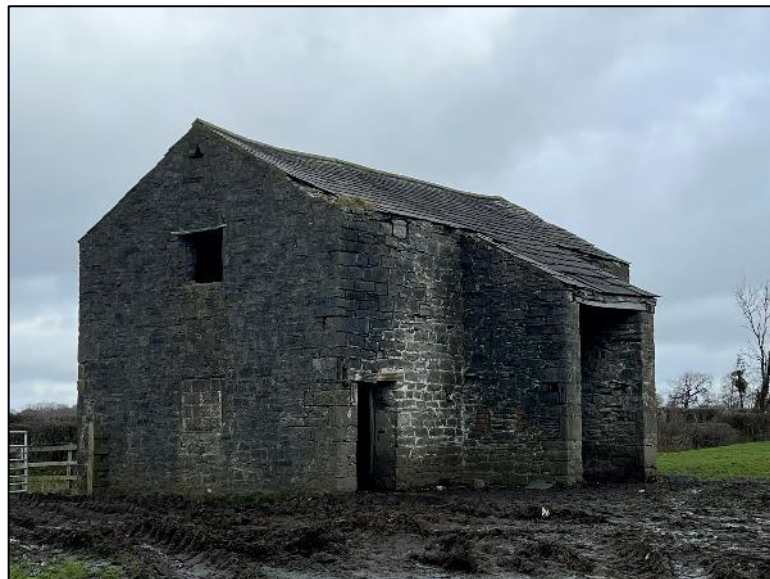
Photo 2: South and east elevations of the barn.
