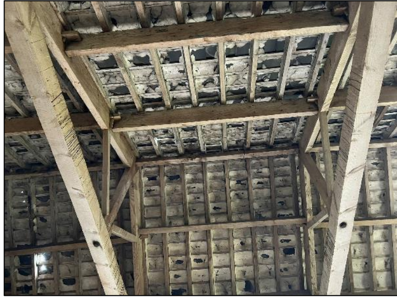
Photo 5: Internal view of roofing materials
