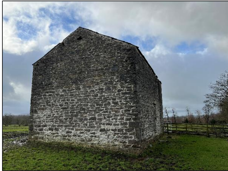
Photo 3: North gable end and west elevation of the barn.
