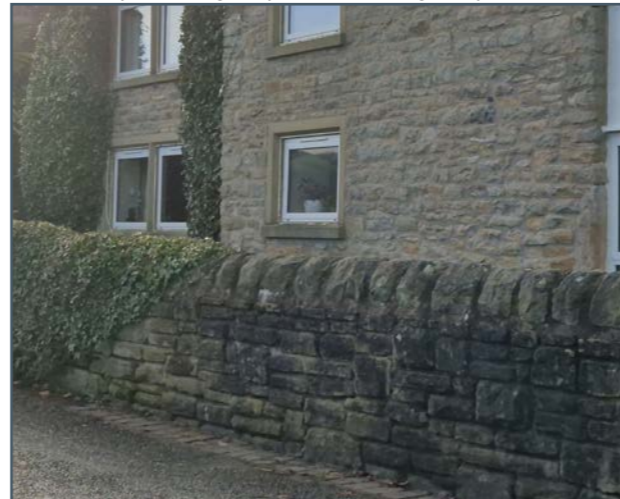
Boundaries: Stone walls, hedges and rural fencing
