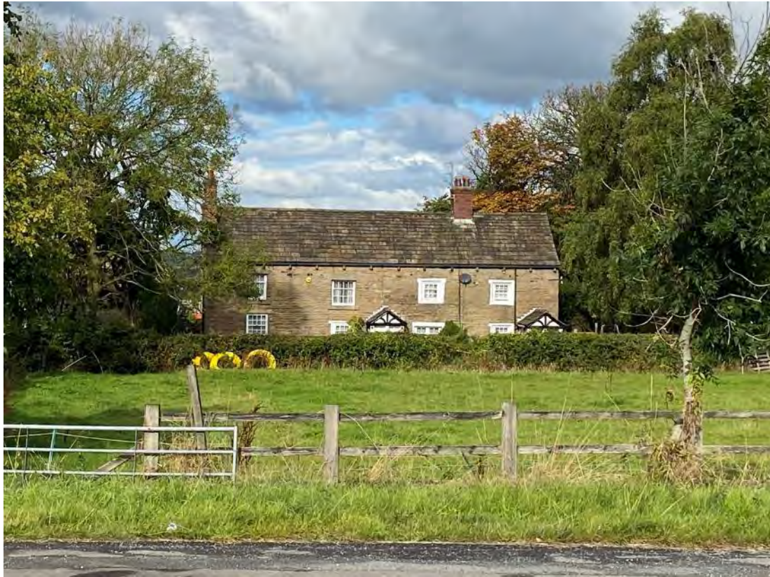
Plate 6. The south-eastern elevation of Causeway Farmhouse from Longsight Road
