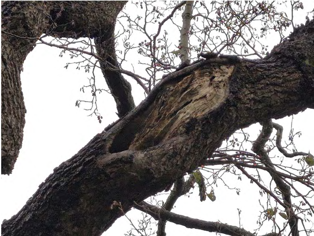
Photograph 9 – T7.6, PRF in the form of a tear out on a northern limb. The cavity extends further into the branch.
