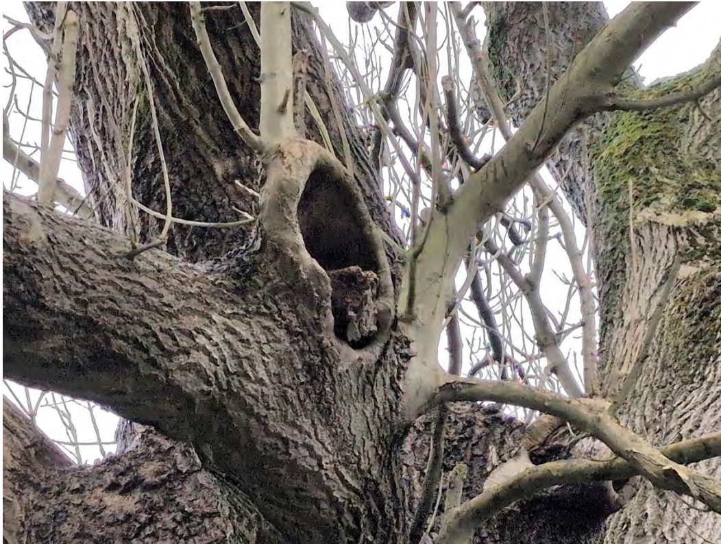
Photograph 23 – T20.3, PRF in the form of a larger tear out on a northwestern limb. The cavity is approximately 10cm in depth and 4cm wide.
