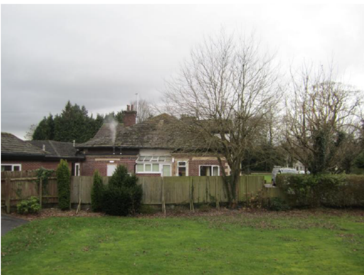
5 North east side elevation of Riverside Care home looking across the front garden of Spring Cottage
