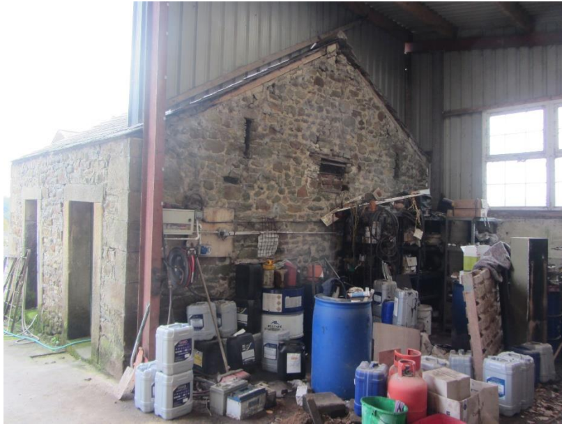
Photo 9 – Barn 3 – view from north west
