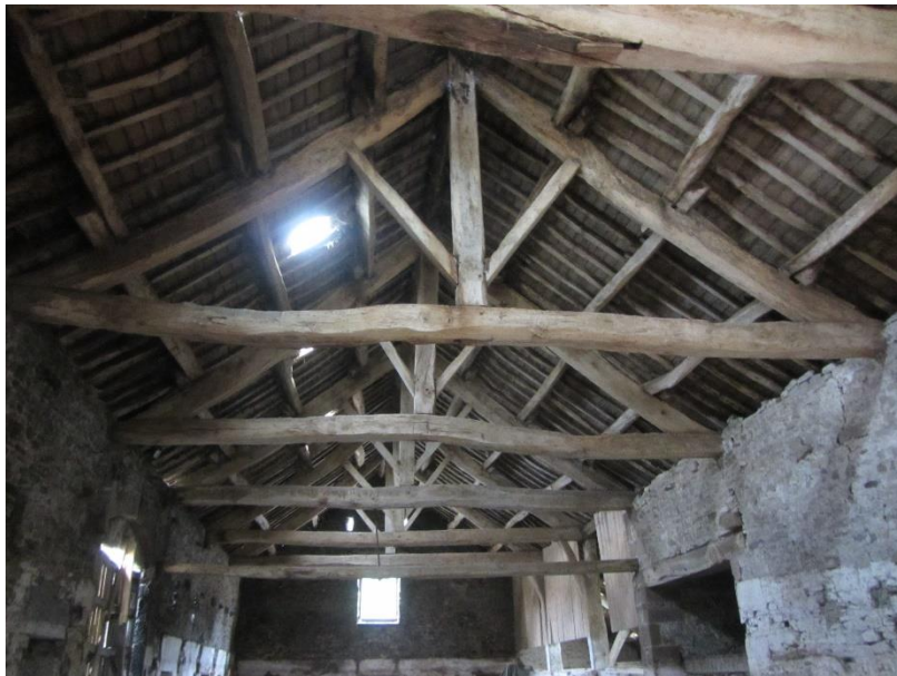
Photo 10 – Barn 1 – main roof structure
