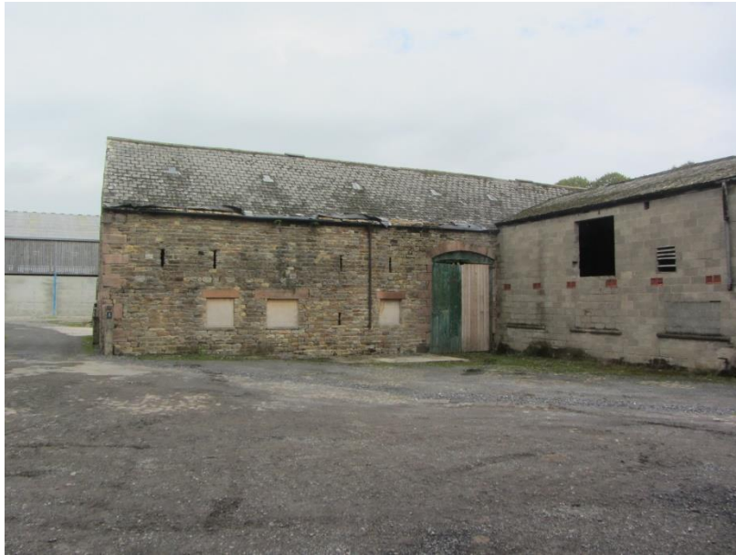
Photo 3 – Barn 1 – view from south
