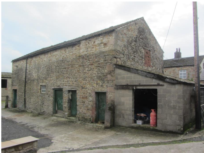
Photo 6 – Barn 2 – view from north west
