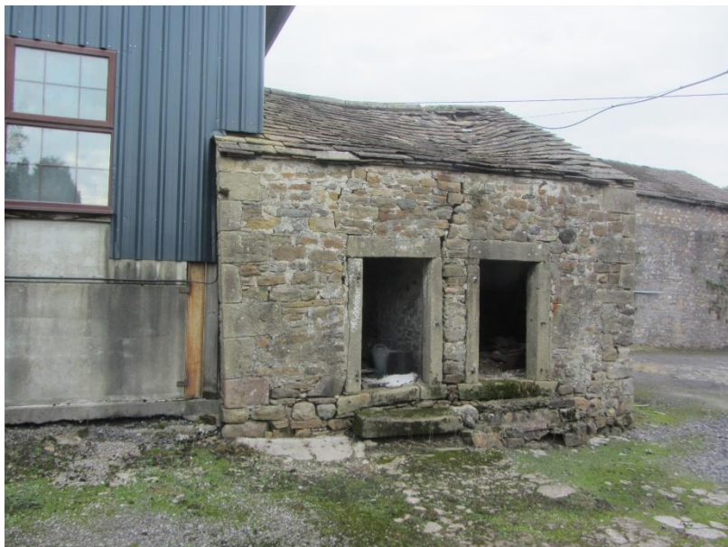
Photo 8 – Barn 3 – view from south
