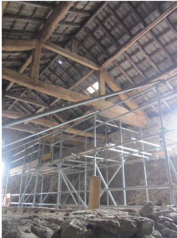
Photo 23 – Barn 2 – roof structure
