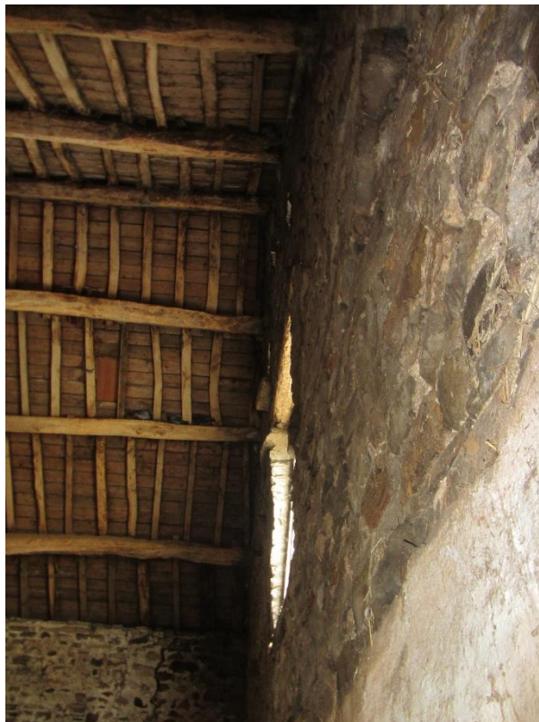
Photo 18 – Barn 1 – west wall
