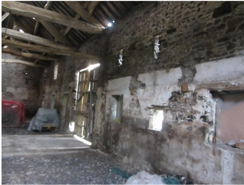
Photo 17 – Barn 1 - south wall
