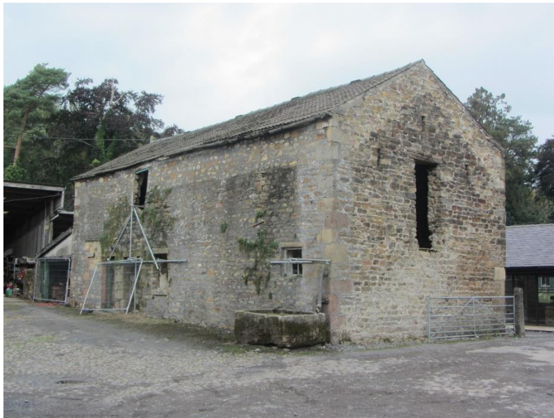
Photo 5 – Barn 2 – view from south east
