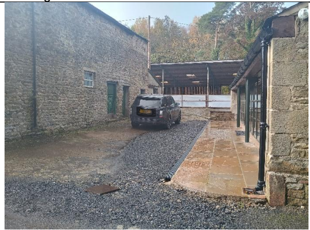
Photo 10: Northern elevation of Barn 2. Office building to right and existing agricultural building in distance to be demolished.
