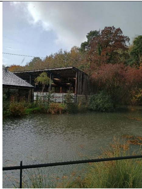
Photo 12: Existing agricultural building to be demolished.
