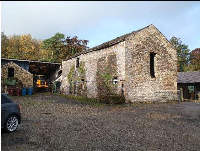
Photo 7: Barn 2 southern and eastern elevations
