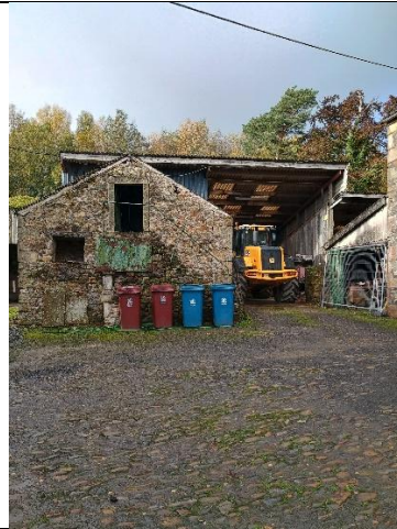
Photo 8: Barn 2 outbuilding. Existing agricultural building to rear to be demolished.
