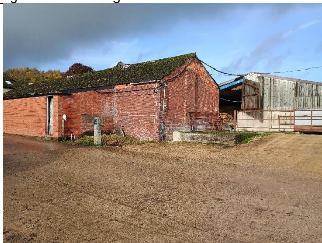
Photo 5: Existing agricultural buildings to south of Main barn to be demolished
