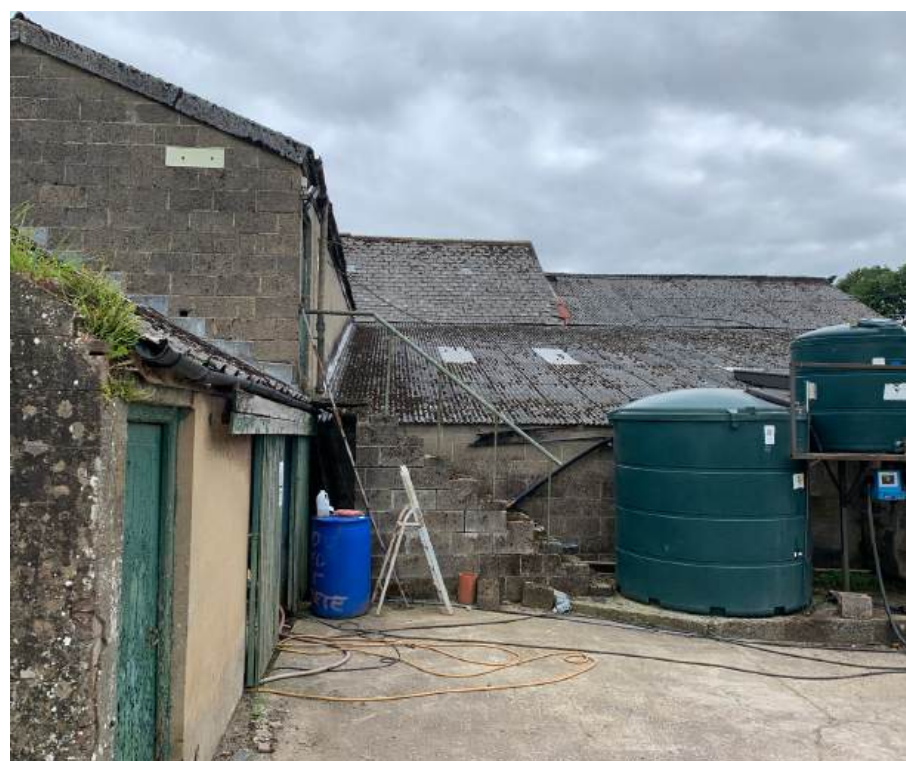
11. C20th farm buildings to south/east of 'main barn'
