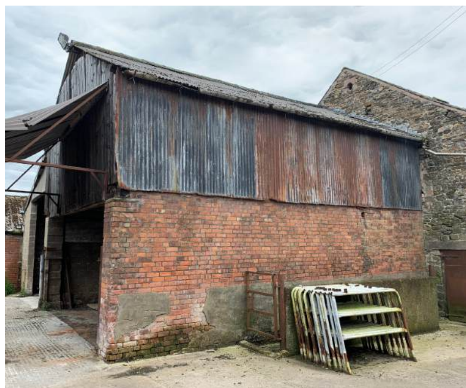
10. East elevation of 'main barn' covered by C20th extension
