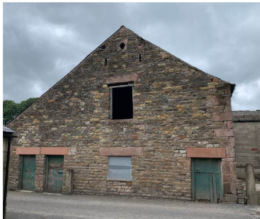
8. West gable of the 'main barn'
