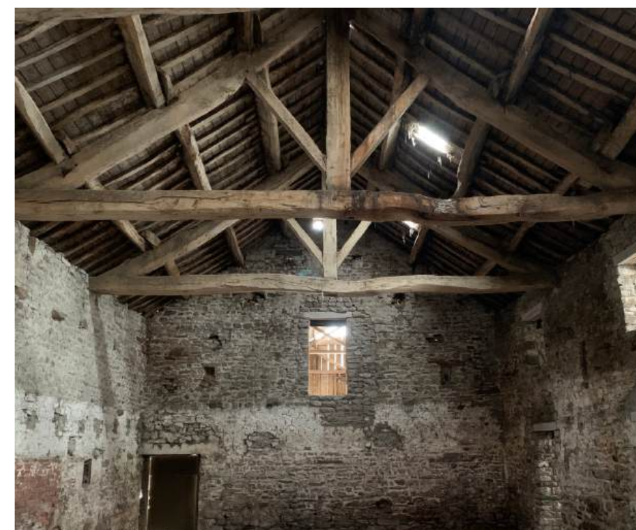
12. Internal view of the hall to 'main barn' with king post trusses
