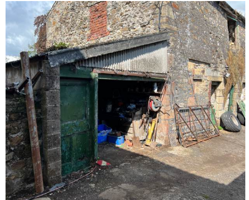
15. C20th lean-to to western gable of 'barn 2'
