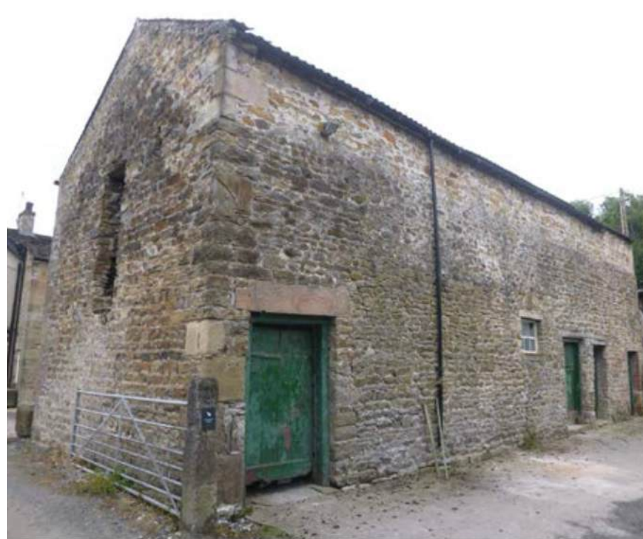
14. North/east elevations of 'barn 2'
