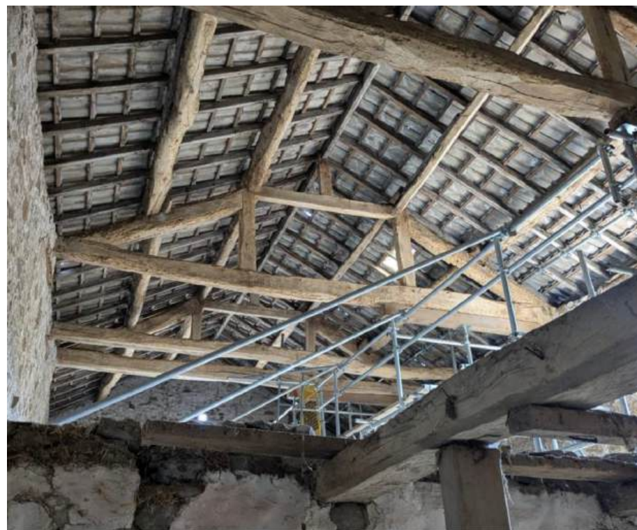
16. Internal view of 'barn 2' with queen post trusses
