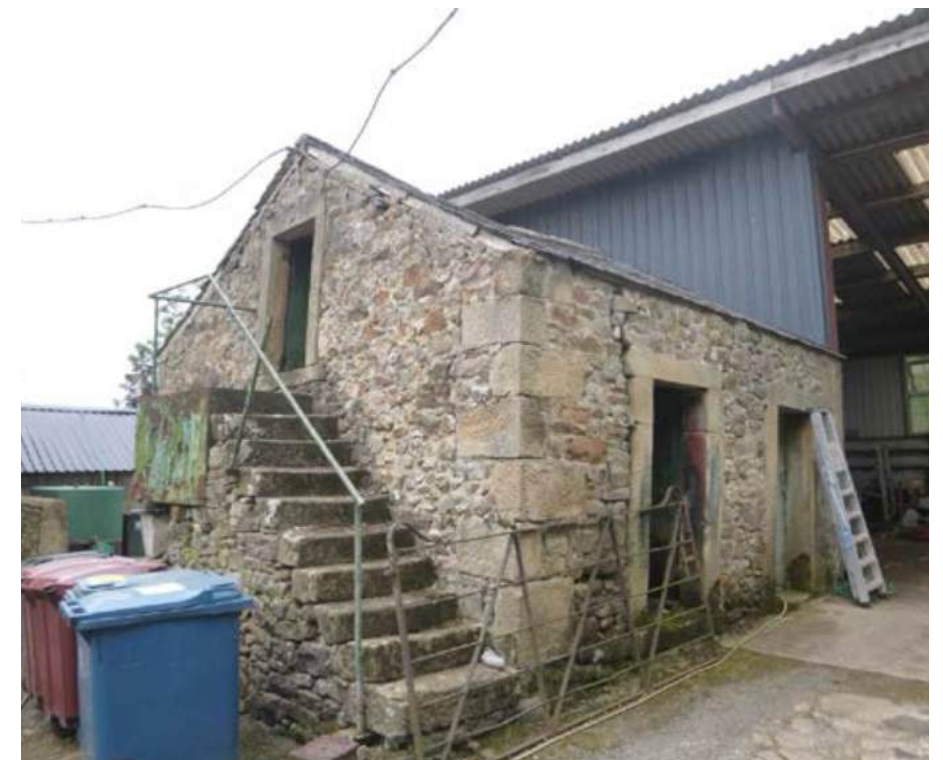
18. North/East of 'barn 3' with external stair to east gable
