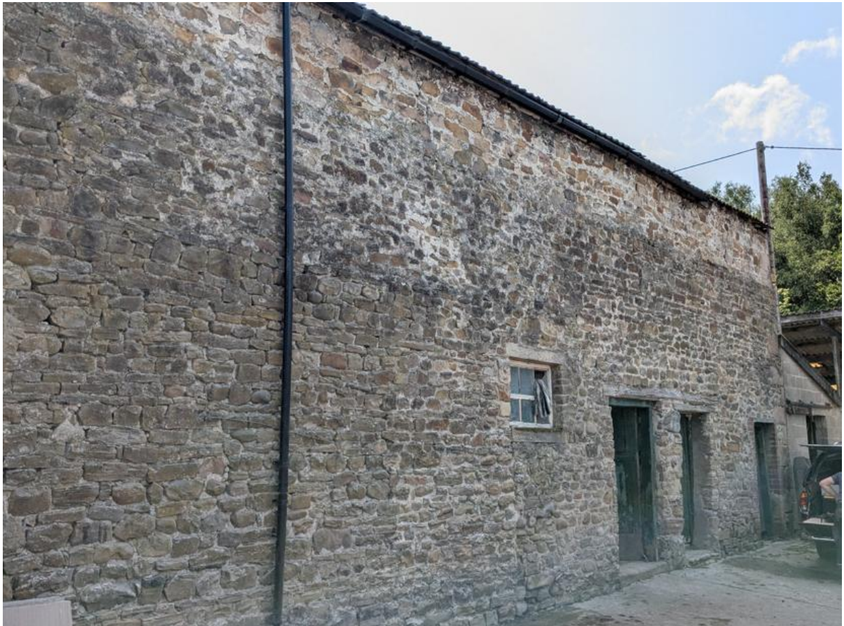
Figure 19) Northern elevation showing altered openings and lower line of a smaller building.
