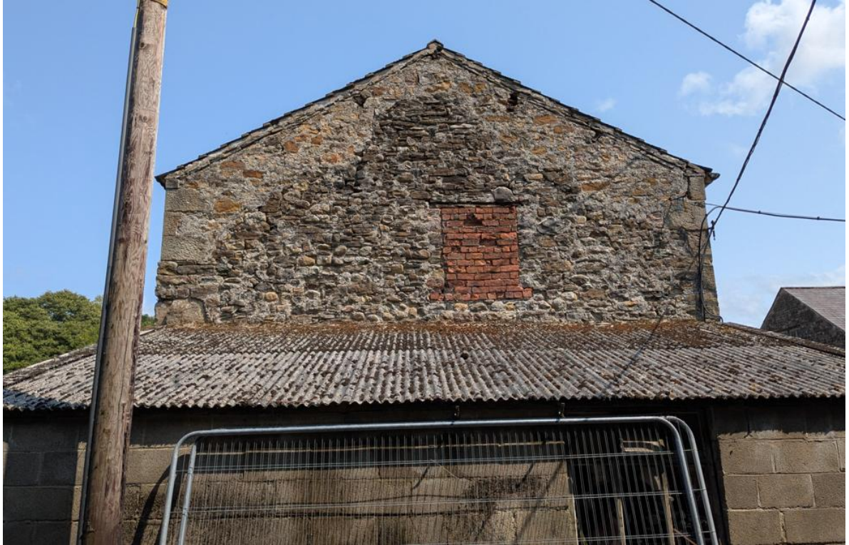
Figure 18) Western gable with adjoined block addition, pitching hole and outline of smaller gable
