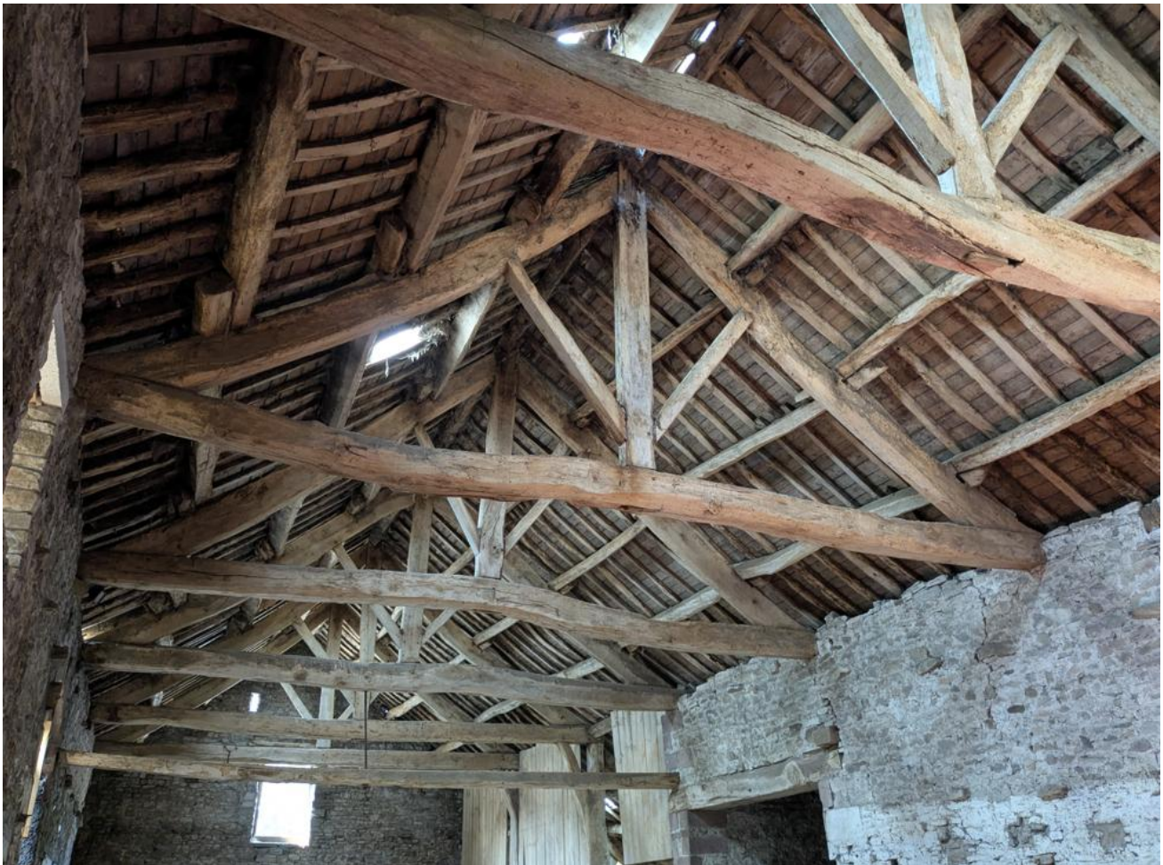
Figure 12) The seven bay king post roof structure inside the main barn with lapped and trencled purlins and over-boarded rafters
