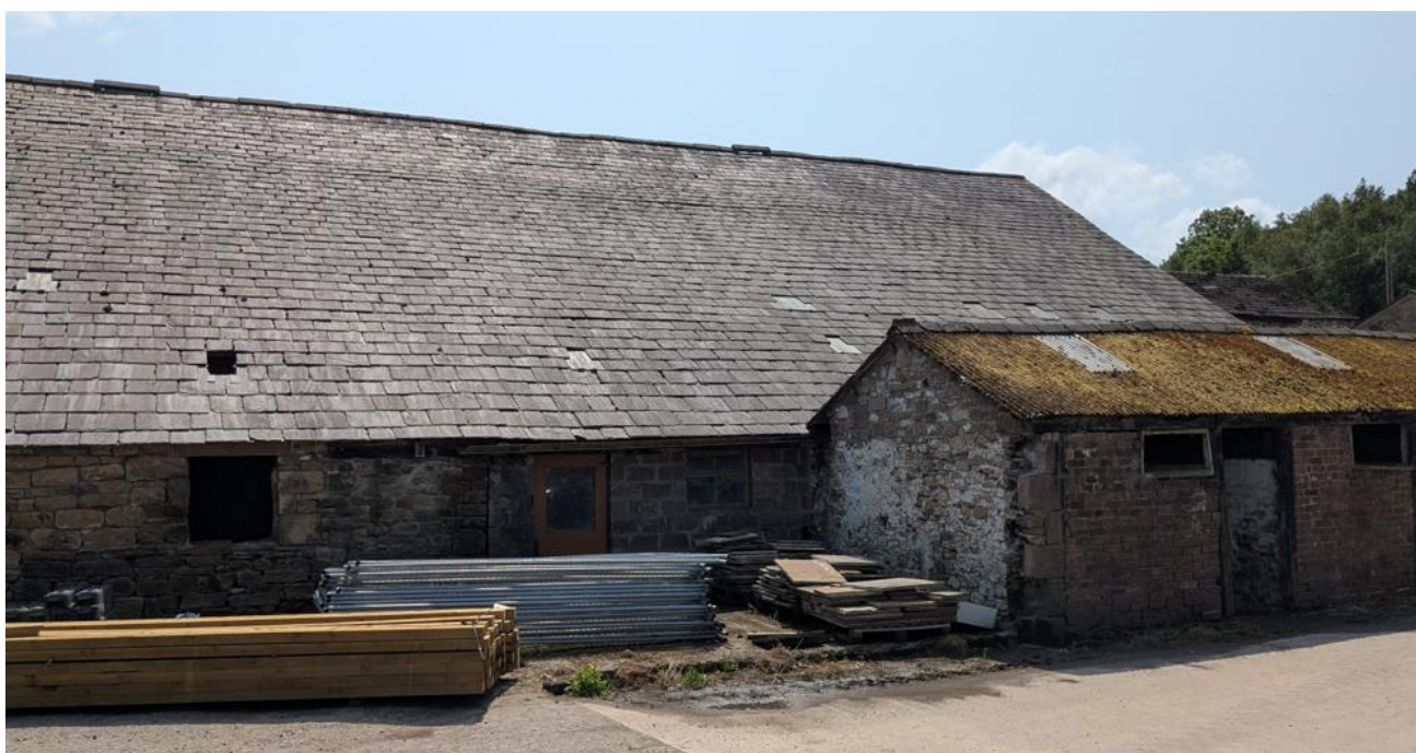
Figure 7) Northern elevation of the main barn with three room shippon which appears to have been shortened in length. There is a blocked large entry door to the main barn wall and signs of various alterations along this elevation where it is presumed the bark mill machinery once operated
