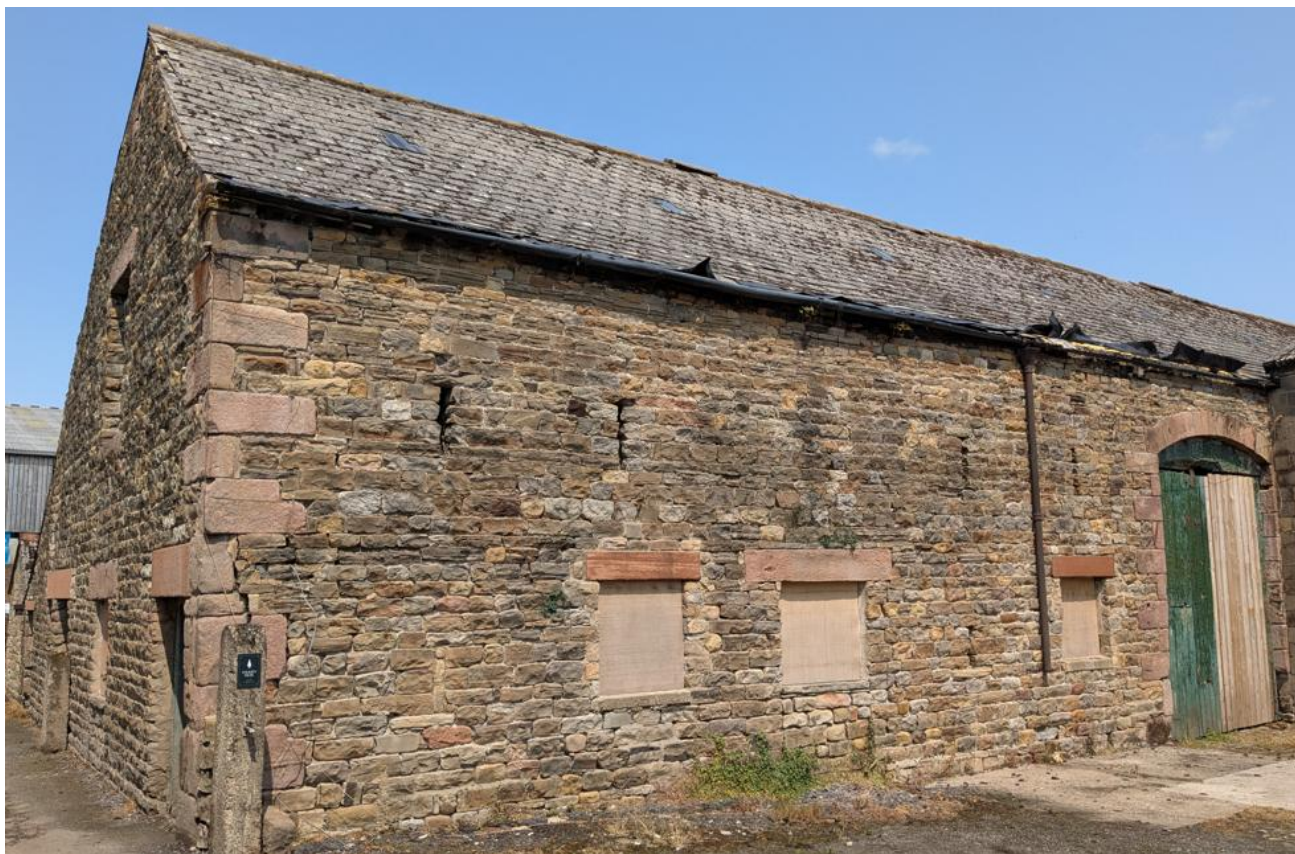
Figure 3) Main barn, west end of the southern frontage, with breather vents to the hay loft, central cart entry (right) and inserted windows to the former ground floor shippon. Blocked former breather vents at lower level suggest this entire end of the building was originally used for crop storage then later altered for cattle housing
