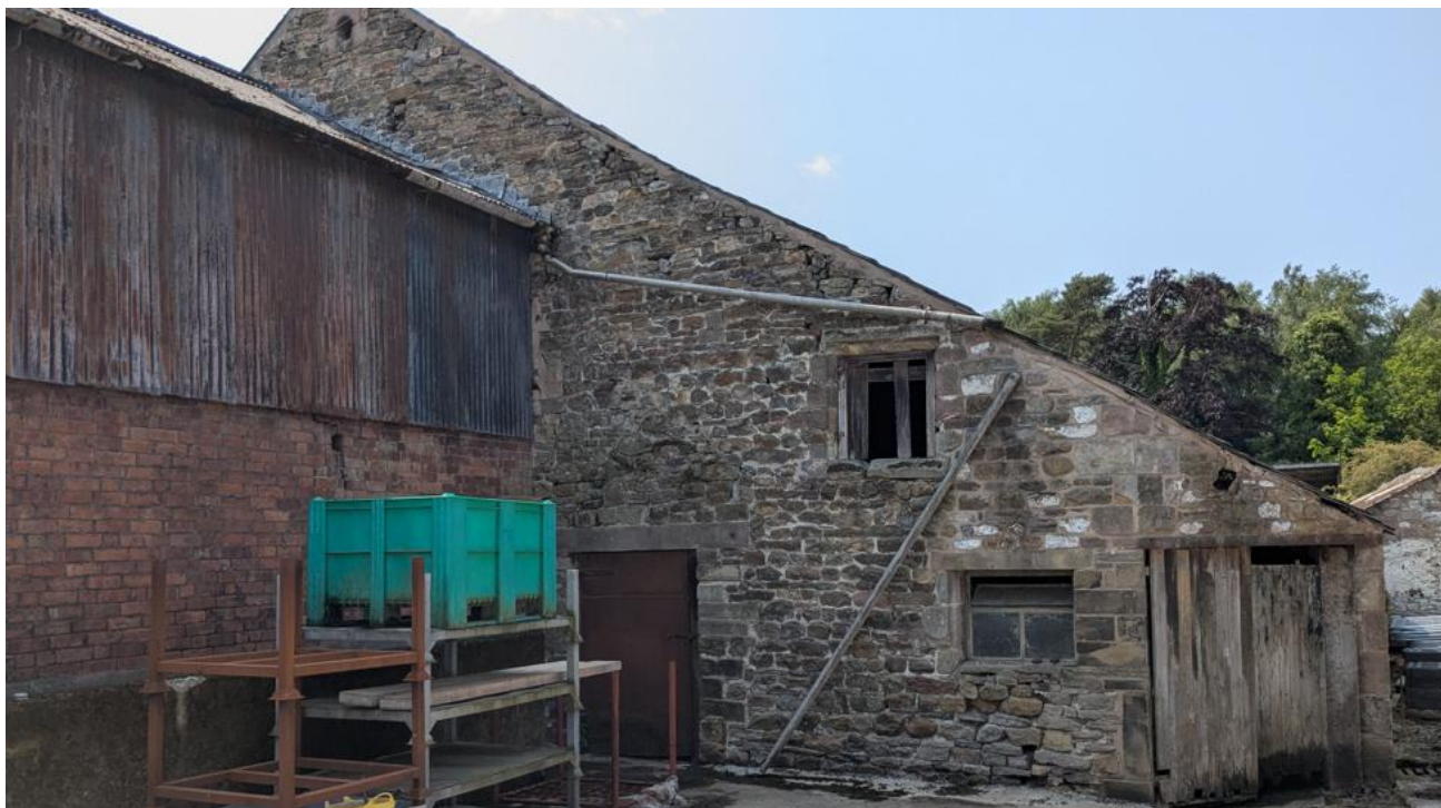
Figure 9) Eastern end of the main barn showing alterations to the lean-to part (right) and large brick addition (C20th) to the centre.
