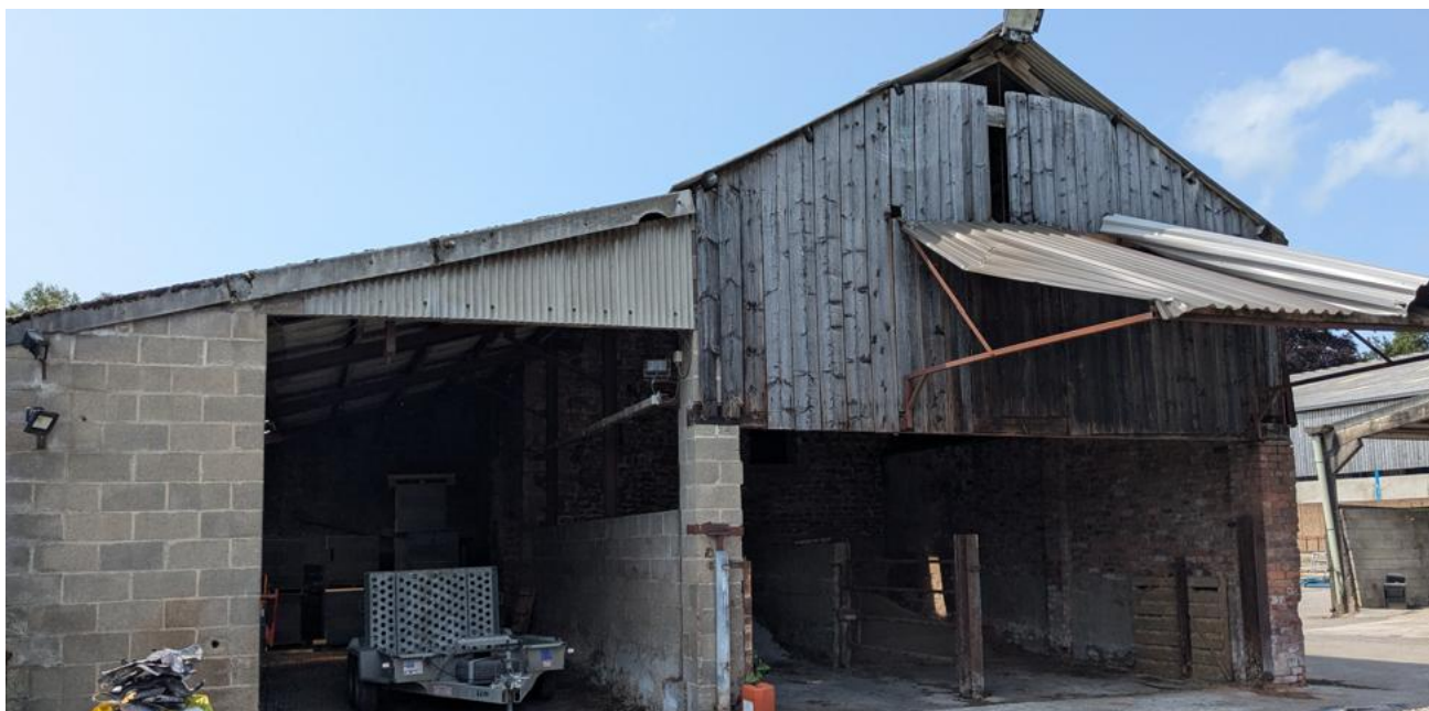
Figure 10) Bricks and block addition to the eastern end of the main barn
