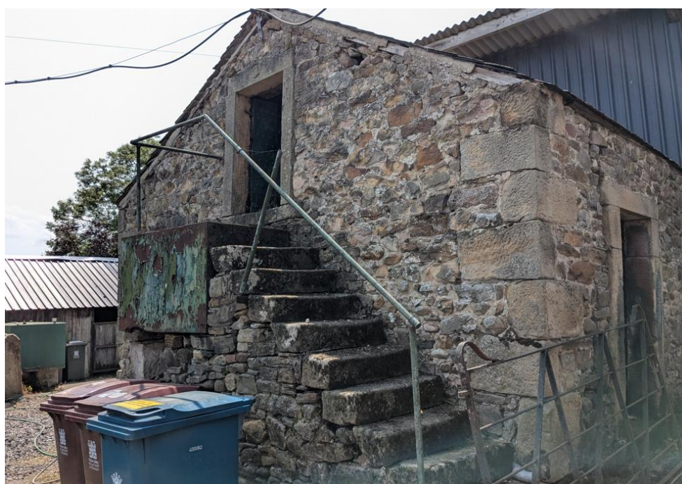
Figure 23) Eastern gable with upper door and stair
