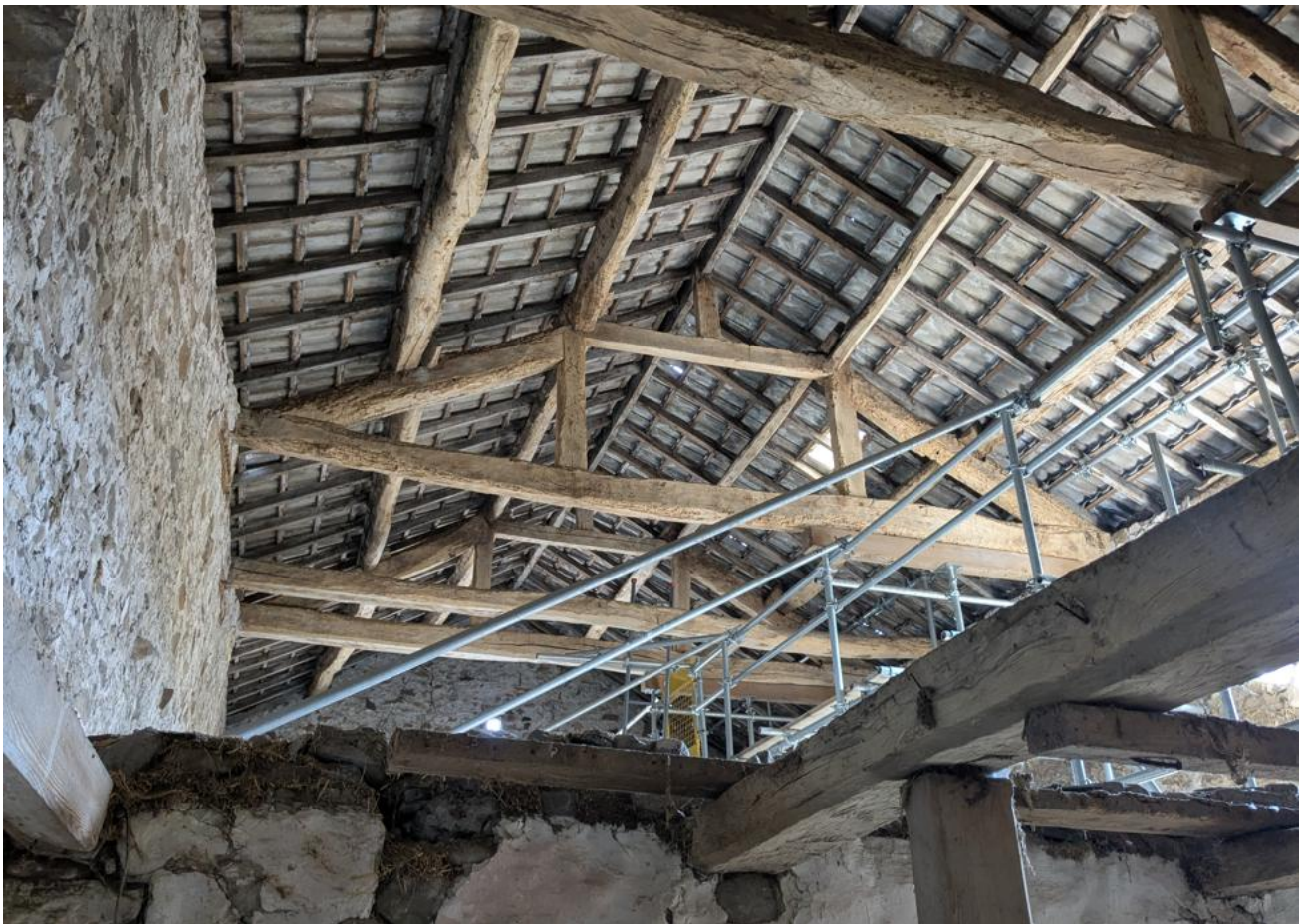
Figure 21) Queen post roof trusses with lapped purlins
