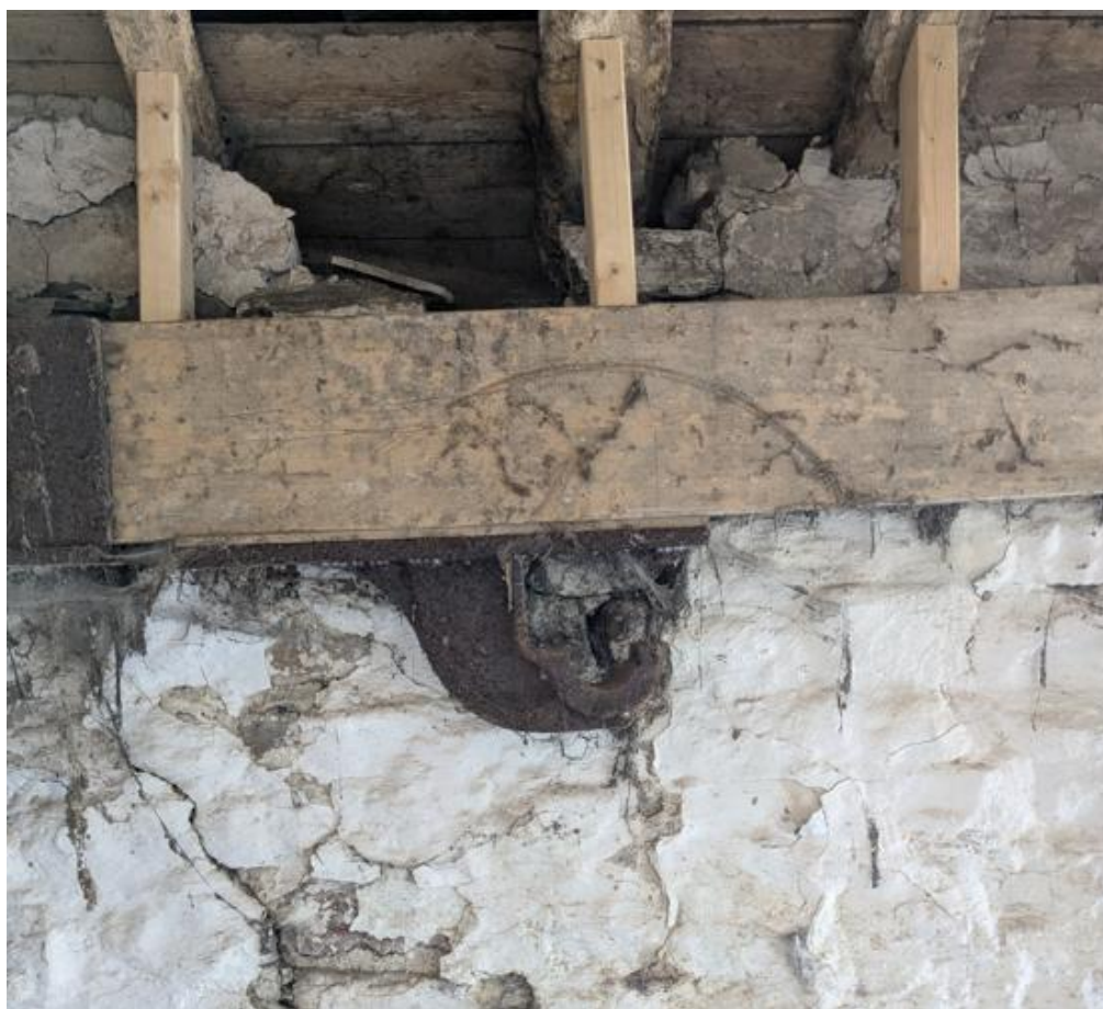
Figure 16) Iron axle bearing in the northern shippon
