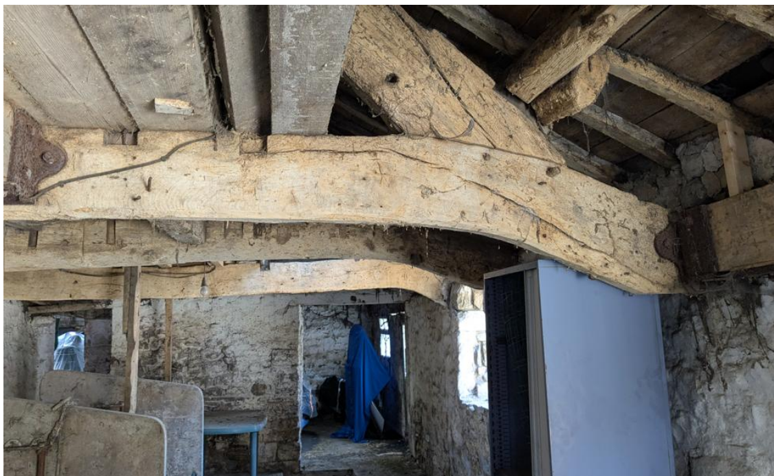
Figure 15) Roof assembly over the lean-to shippon to the north side of the main barn, with unusual cranked tie beam bearing ends - presumably used to increase head height inside the building. Note also iron bracket bearings connecting longitudinal members, possibly associated with the support of milling mechanisms and inserted later rather than original
