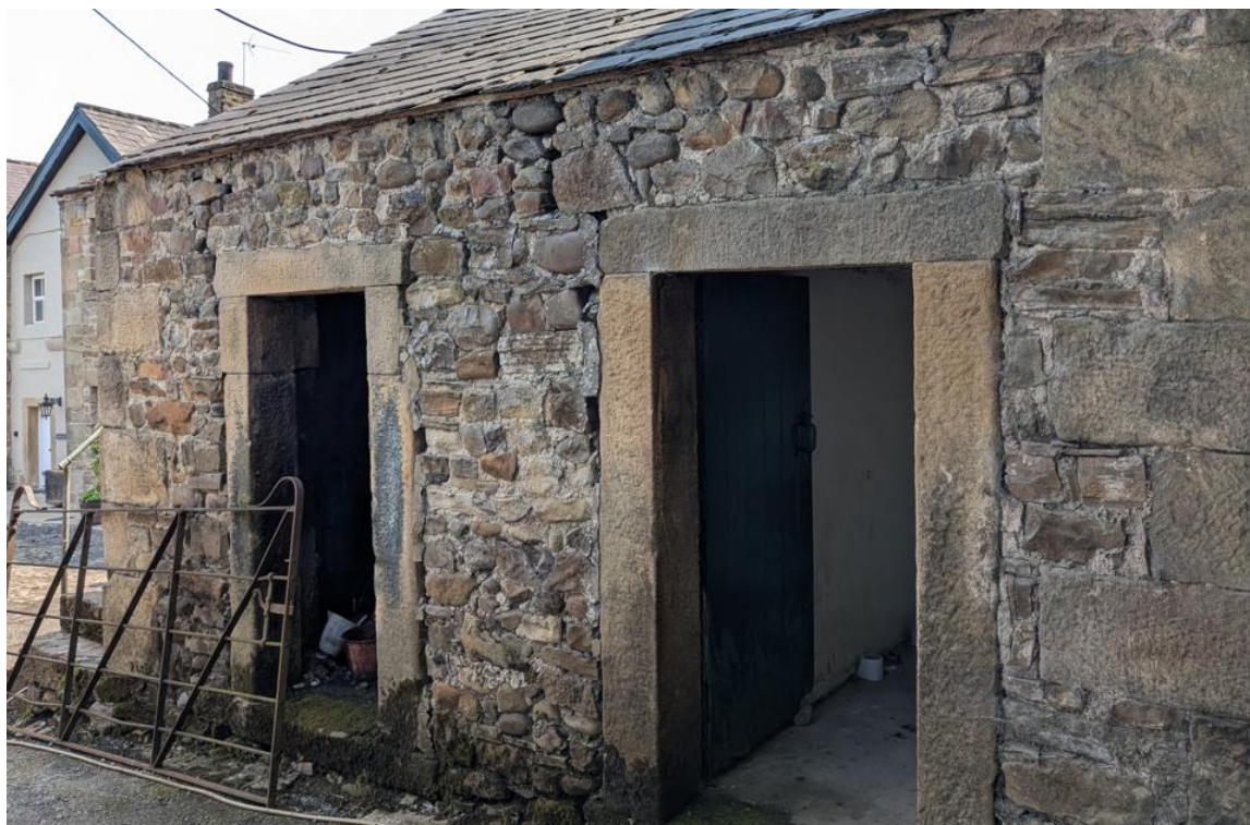
Figure 22) Former pigsty/store northern elevation
