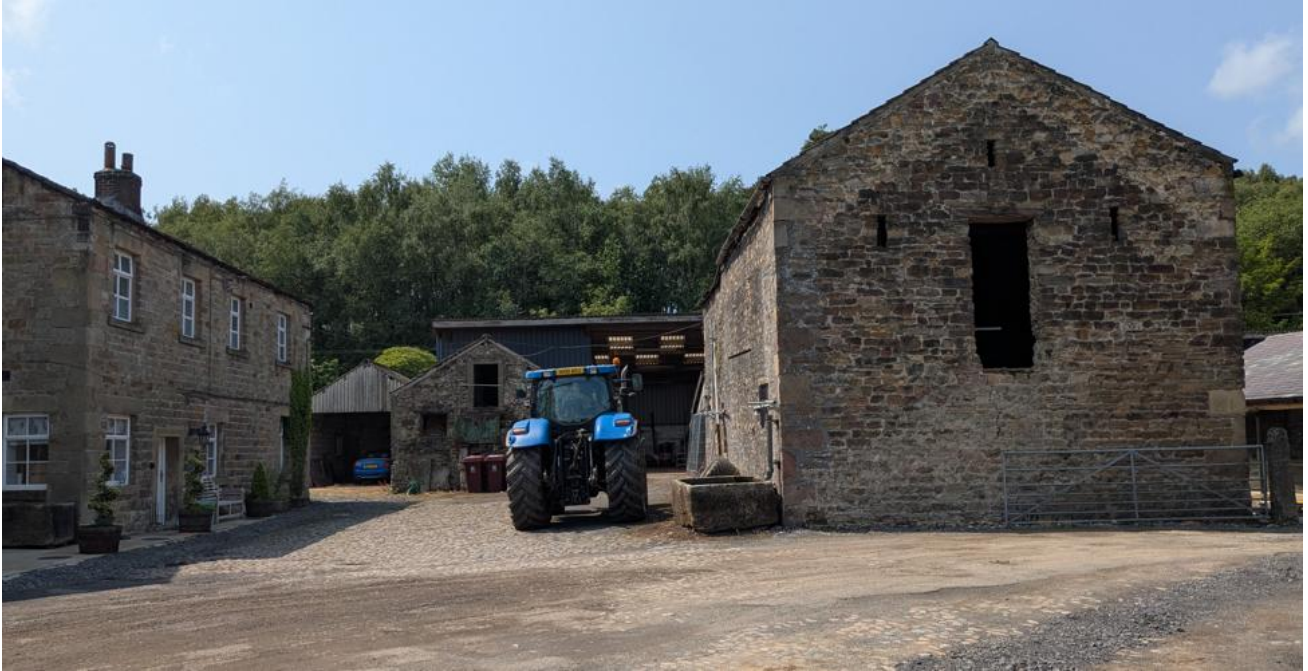
Figure 20) Eastern gable showing breather vents, pitching door and proximity of the hall (left). The outline of the lower building is also evident on the gable
