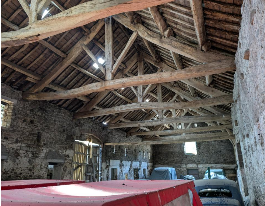
Figure 13) Main barn interior looking towards the west end
