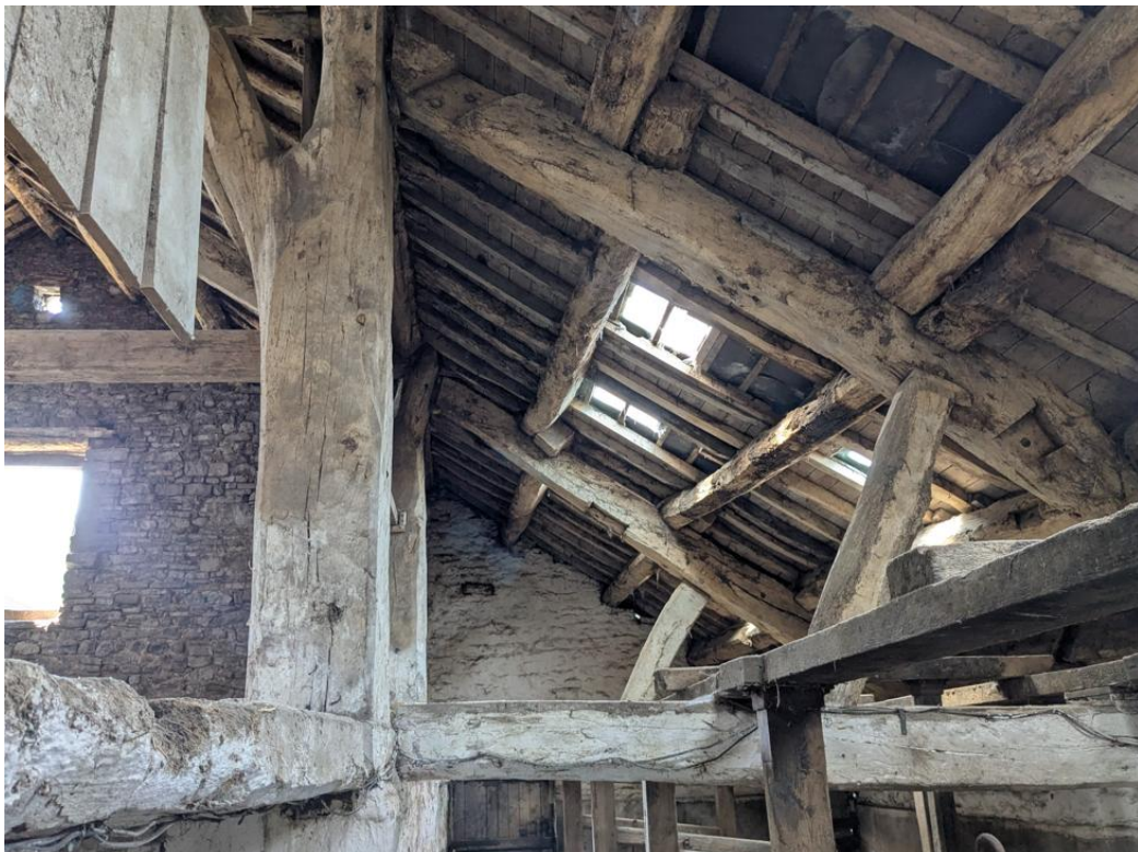
Figure 14) Western end of the main barn – here the main volume is partially aisled with vertical upright posts carrying the main roof trusses and the lean-to shippon roof. This open plan element suggests shared usage of space between the main volume and the lean-to (possibly connected to the bark milling process – e.g. drying space)
