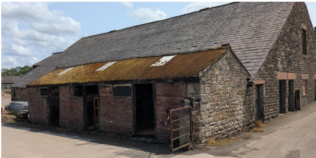
Figure 6) The main barn, north side, with the altered three room shippon addition in the foreground. The building has a brick front wall and stone flank walls. The brick walls may have enclosed a former open structure, possibly used for storing/processing tree trunks/bark as part of the bark milling process
