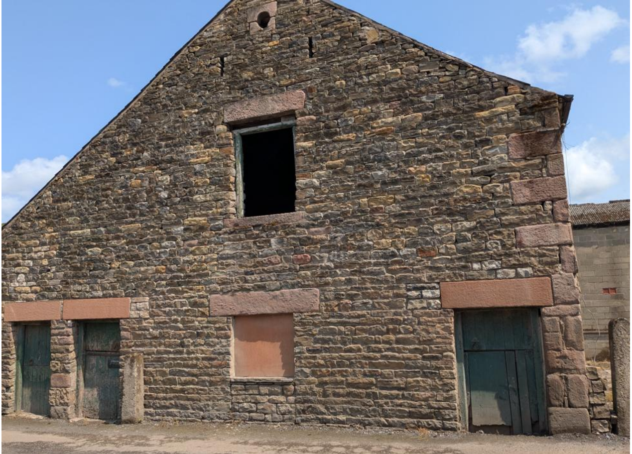
Figure 5) Western gable of the main barn. Note the loft pitching door, gable owl hole and three door formation (central door altered as a window) which is typical of the Lancashire barn typology, the outer doors being for access to the drain passages and the central door for the feed passage. These all appear to be inserted openings rather than original formed when the building was altered for cattle housing. The extreme left door accesses the lean-to part, also last used as a shippon
