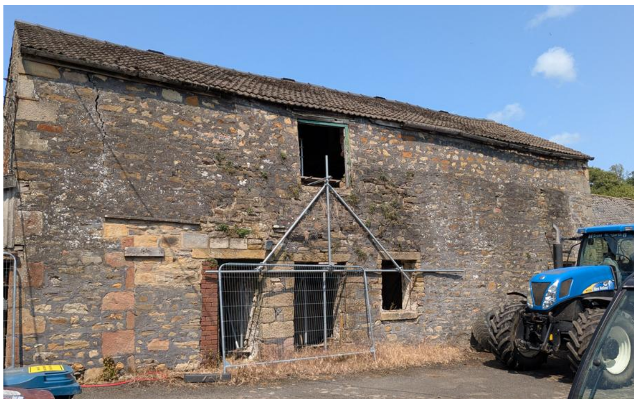
Figure 17) The secondary barn, southern elevation facing the hall. Note the upper central pitching door, altered doors at ground floor level and the outline of a lower building
