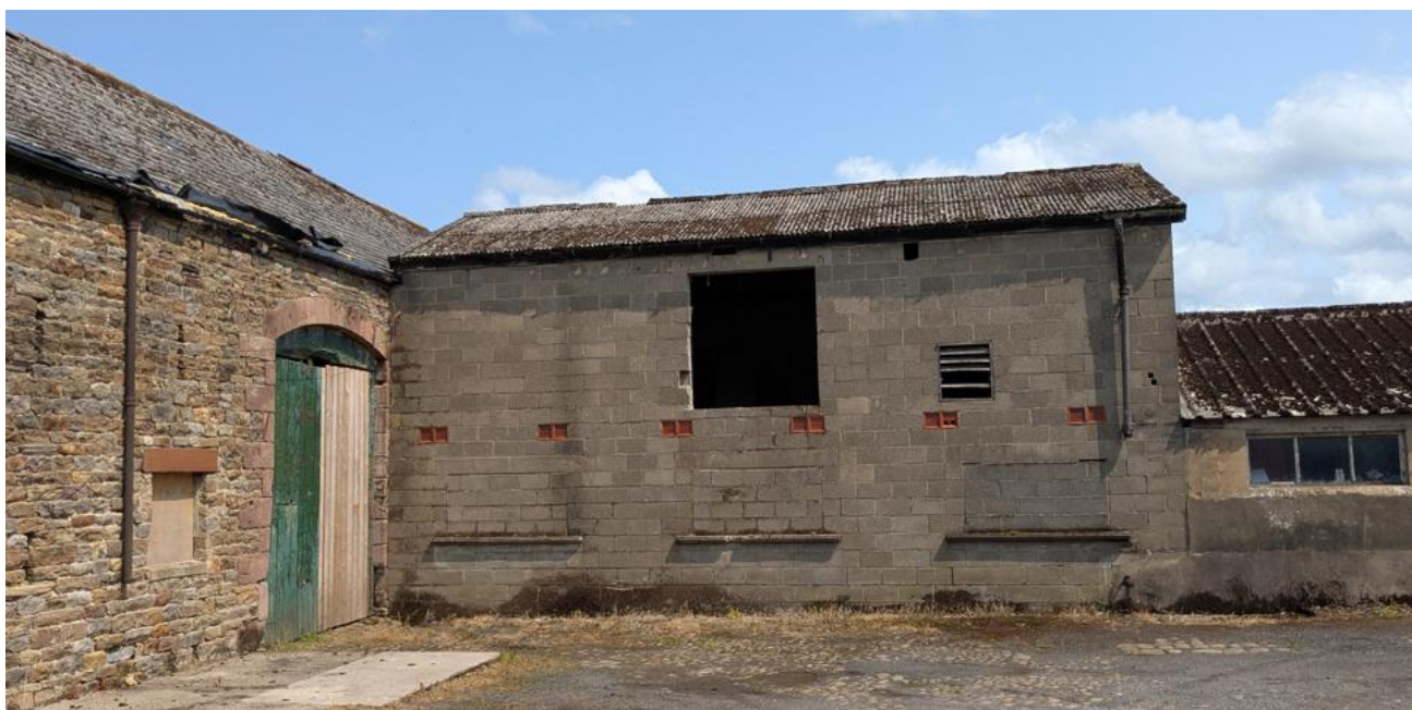
Figure 4) Large C20th block addition to the main barn south side
