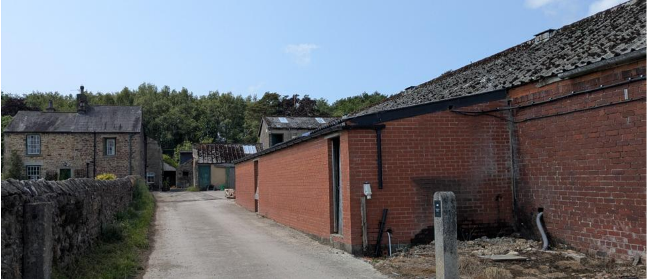
Figure 11) Large modern brick extension to the main barn with Winkley Hall distant left
