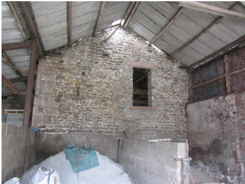
Photo 4 – Barn 1 – view from east (from within extension)
