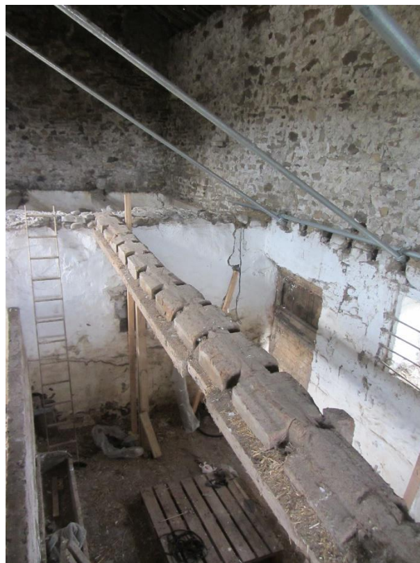
Photo 26 – Barn 2 – original floor beam
