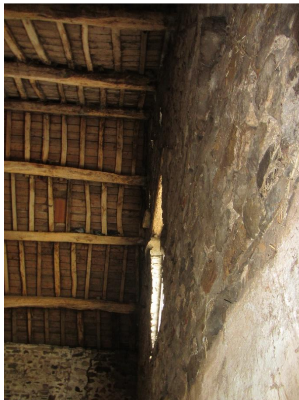
Photo 18 – Barn 1 – west wall
