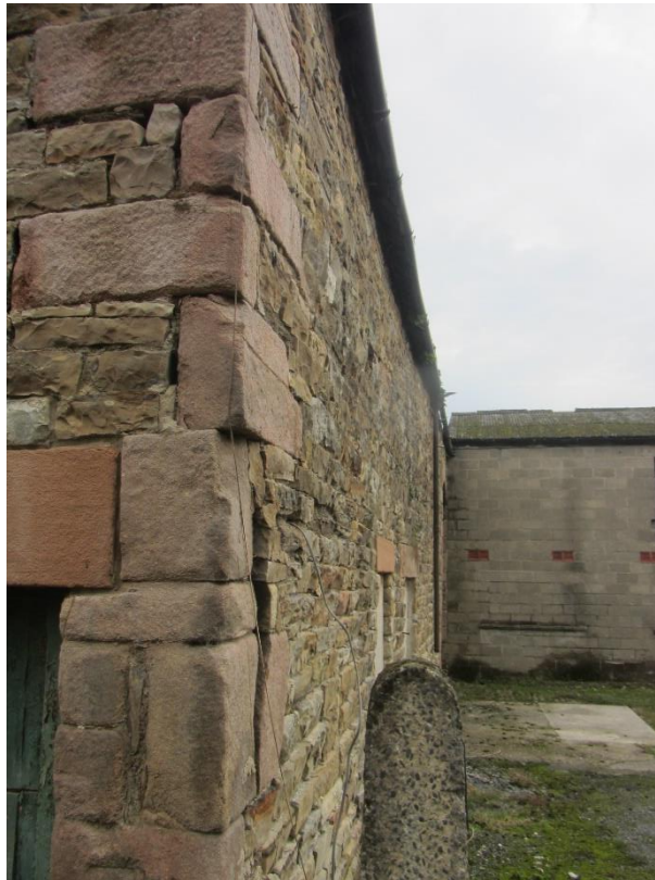
Photo 21 – Barn 1 - south west corner
