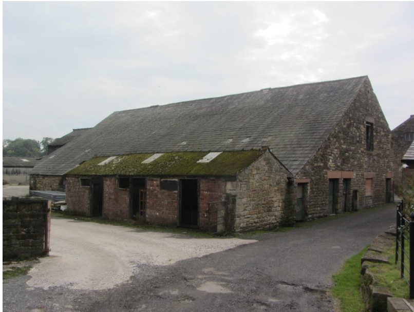
Photo 1 – Barn 1 - View from north west
