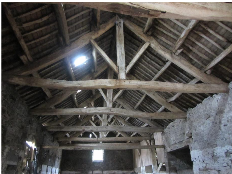
Photo 10 – Barn 1 – main roof structure
