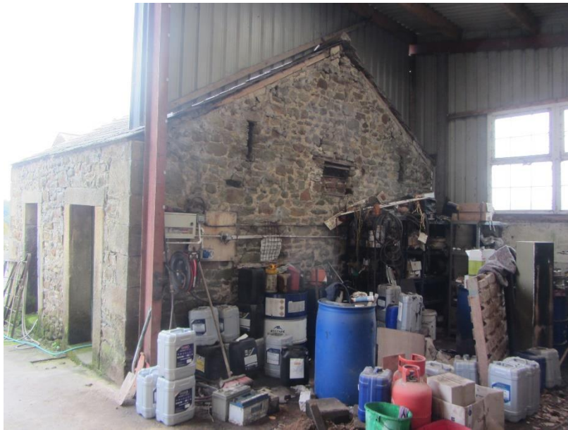
Photo 9 – Barn 3 – view from north west
