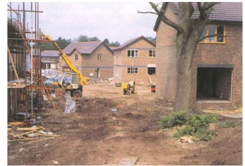
Ground protection is essential to maintain the health of tree roots on construction sites.
