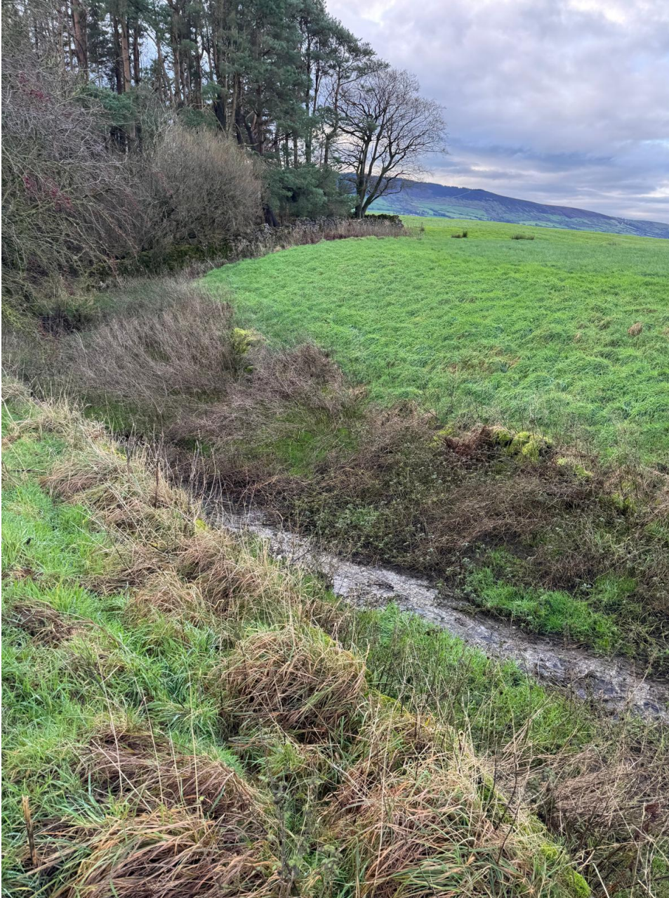
Photo 4 – Watercourse section south of the field
