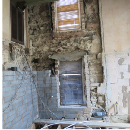
Wall with Masonry Leaf Removed and 1950s North Elevation with Inner Masonry Removed
