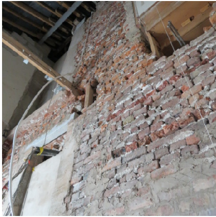
Wall with Masonry Leaf Removed and 1950s North Elevation with Inner Masonry Removed
