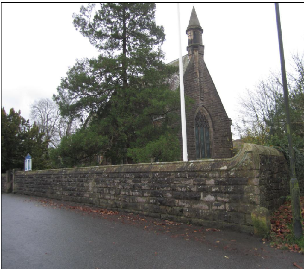
3 Stone boundary wall to All Saints Church
