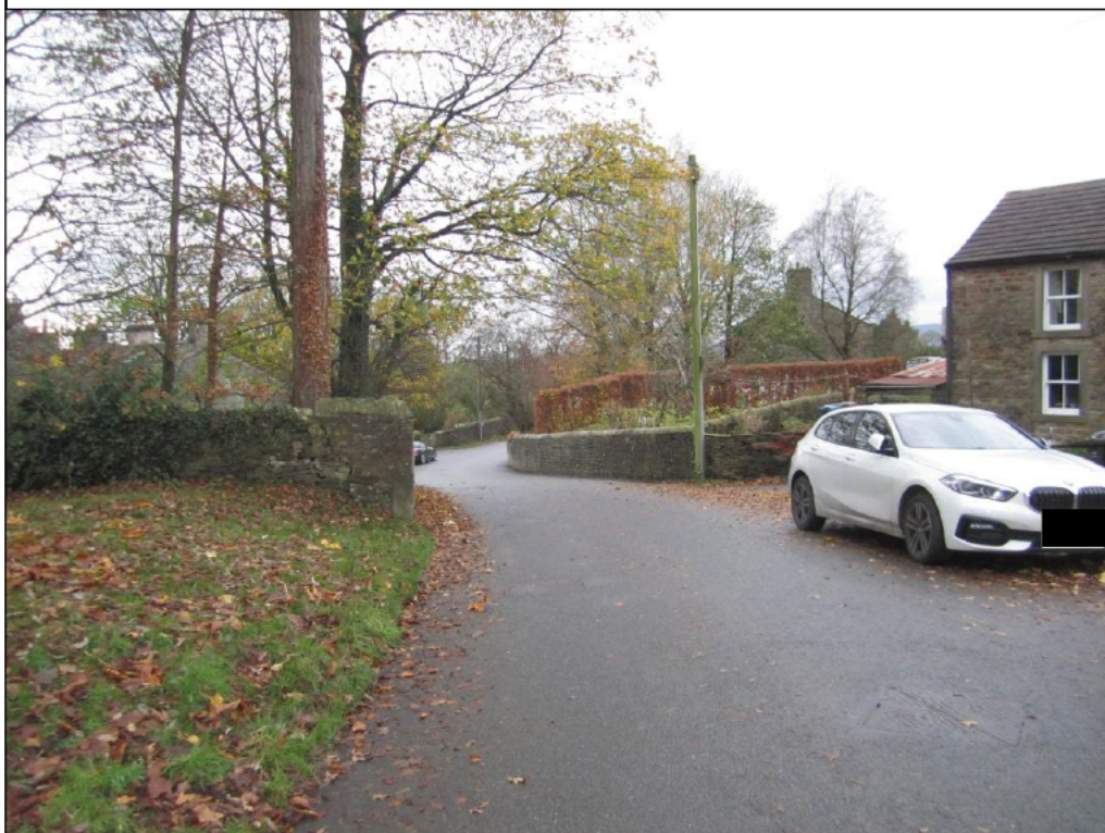
4 Boundary wall to the south of Dickinson Farm
