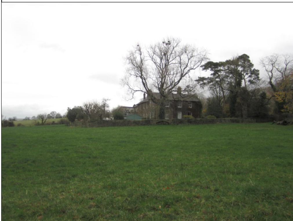
2 The stone boundary wall to the Vicarage looking north-east from the rear of The Old Village School
