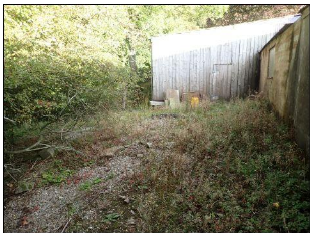
Photo 24: Building 2, eastern elevation
