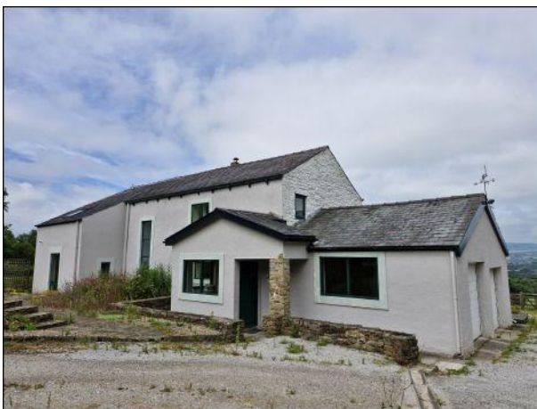
Photo 13: Building 1, southern elevation
