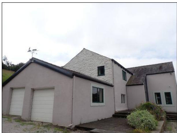
Photo 14: Building 1, eastern elevation
