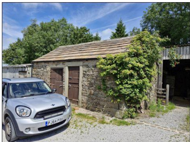
Photo 28: Building 3, southern and western elevations
