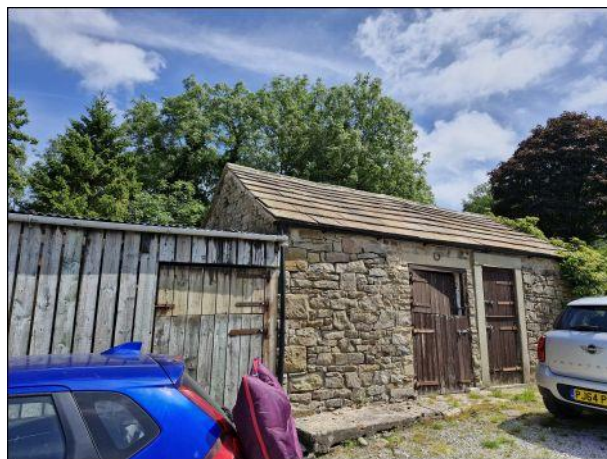
Photo 29: Building 3, northern and western elevations
