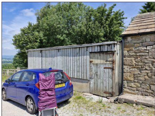
Photo 22: Building 2, north-western corner
