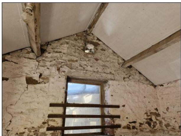
Photo 30: Building 3, internal area
