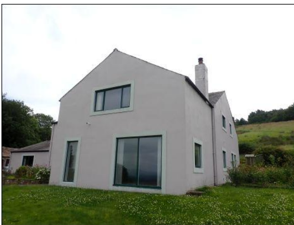
Photo 15: Building 1, northern elevation
