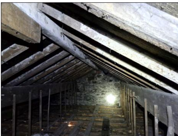
Photo 17: Building 1, eastern roof void
