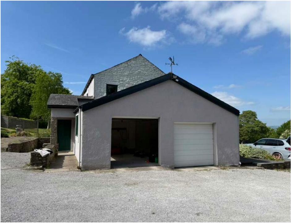
Garage and rear entrance porch.
