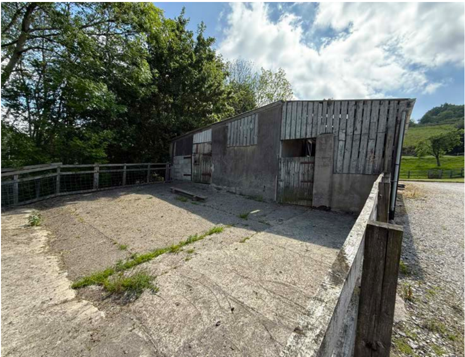
Outbuilding and stable yard.
