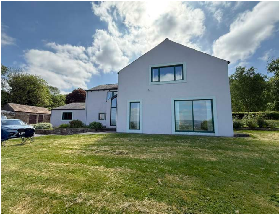
Front elevation and entrance.
