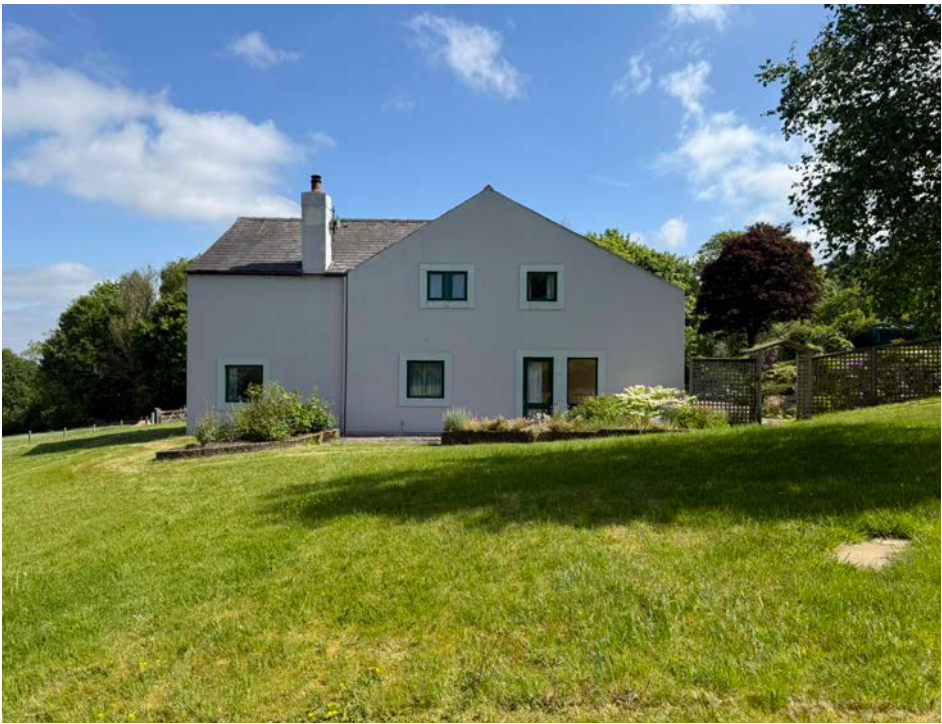
South-West elevation and rear garden.
