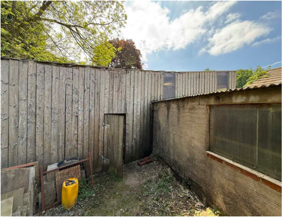
Rear of outbuilding.
