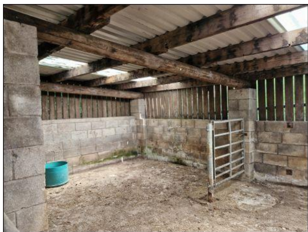
Photo 27: Building 2, internal area
