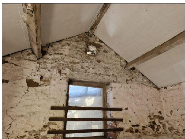
Photo 31: Building 3, internal area
