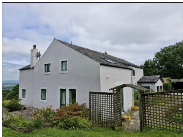
Photo 17: Building 1, western elevation
