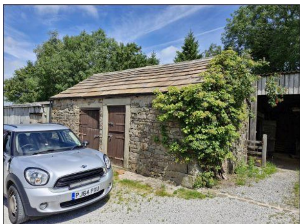
Photo 29: Building 3, southern and western elevations
