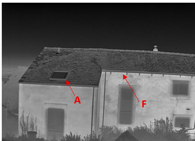
Photo 37: Dusk emergence survey position 4, showing Roost 2 Emergence Points A and F
