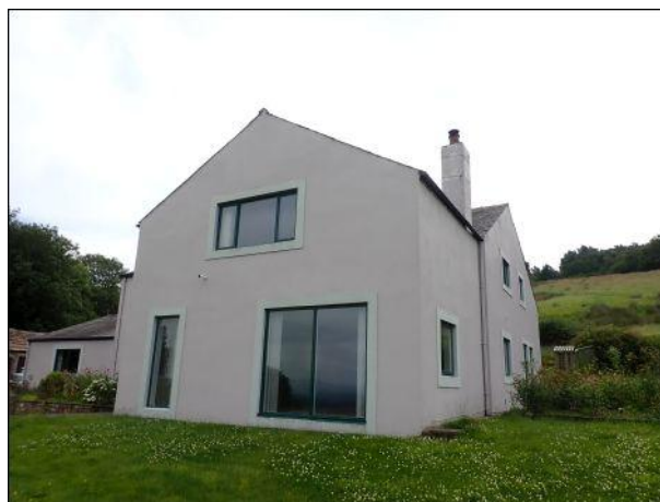
Photo 16: Building 1, northern elevation
