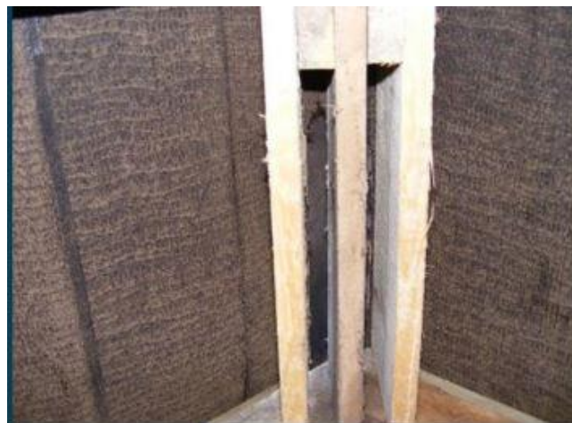
Insert 9: Examples of a 'Triple Ridge Board' system to be used within the bat house to create additional roosting locations for use by brown long-eared bats
