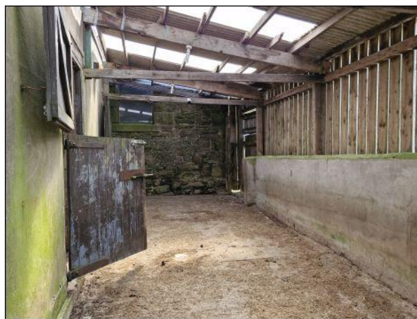
Photo 26: Building 2, internal area
