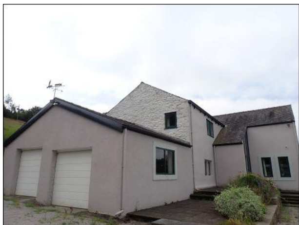
Photo 15: Building 1, eastern elevation
