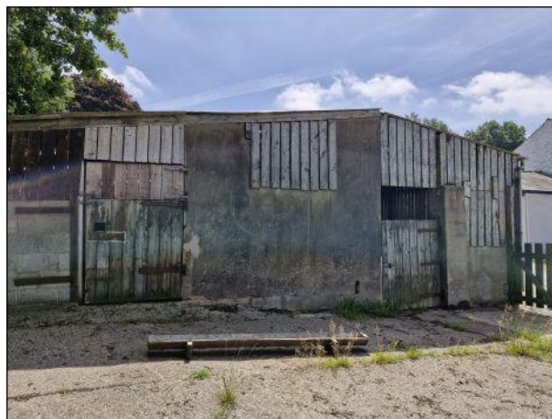
Photo 24: Building 2, northern elevation
