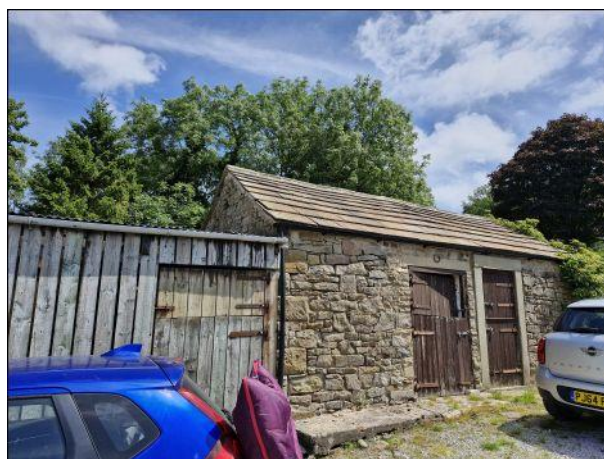
Photo 30: Building 3, northern and western elevations
