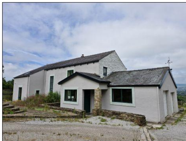
Photo 14: Building 1, southern elevation
