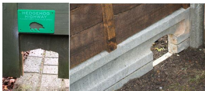
Insert 4: Showing wildlife access gap within fencing
